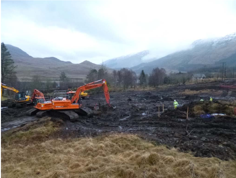
Plate 1 - General view of machine chain stripping peat
