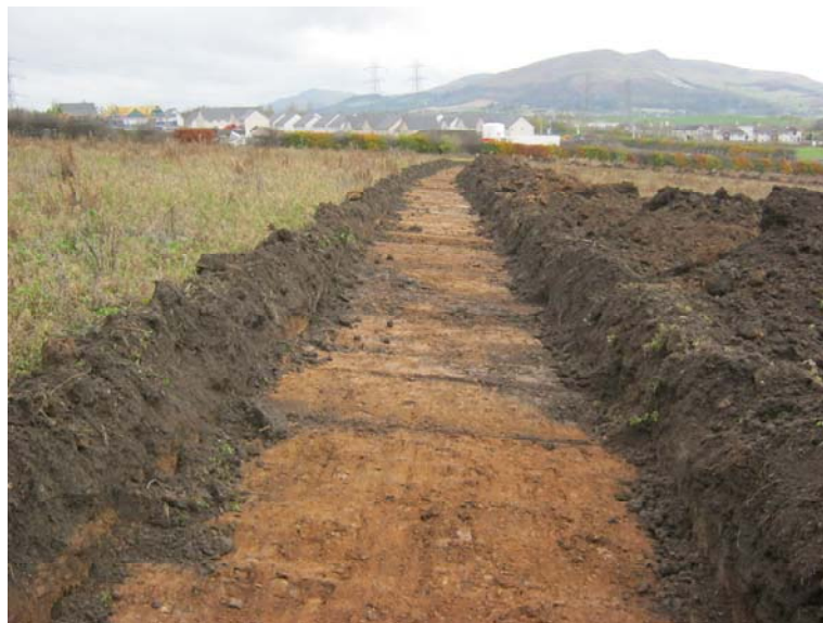
Plate 3: Trench 4 post-excitation from south-east
