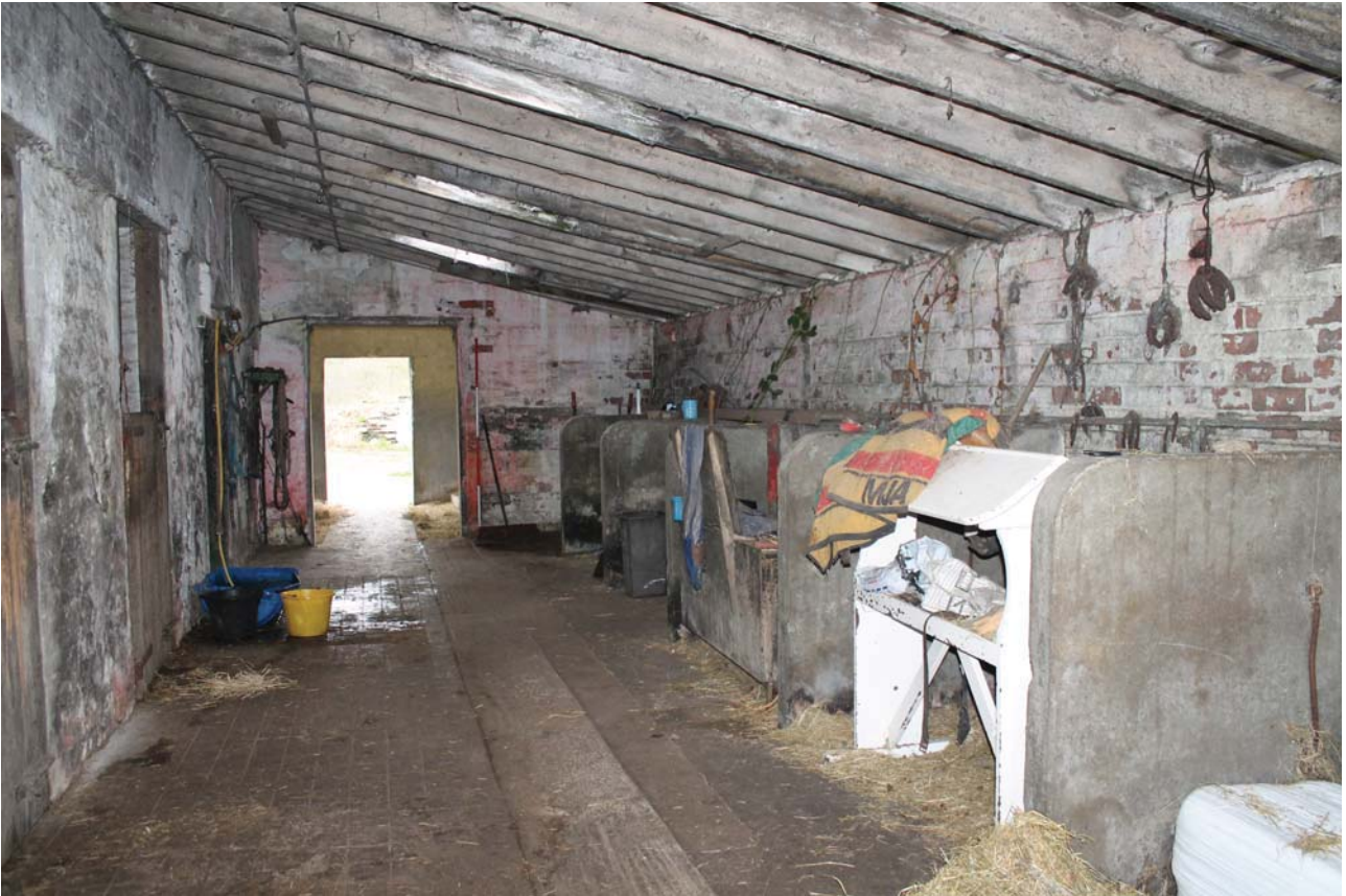
Plate 47: High Corton Farm, Barn B, general view of the brick extension from the north-west
