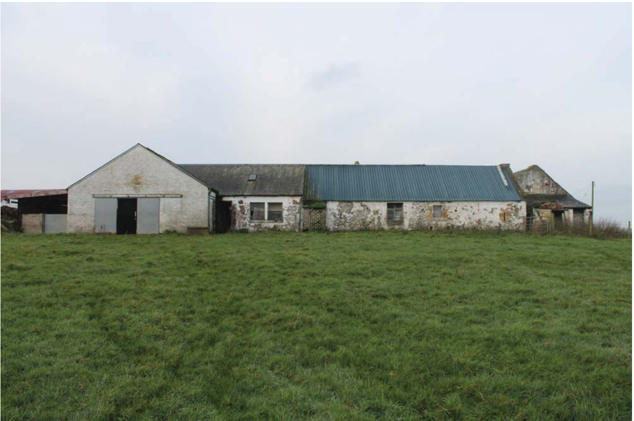
Plate 26: Laigh Corton Farm, Barns C & D, north-east elevation, general view from the north-east
