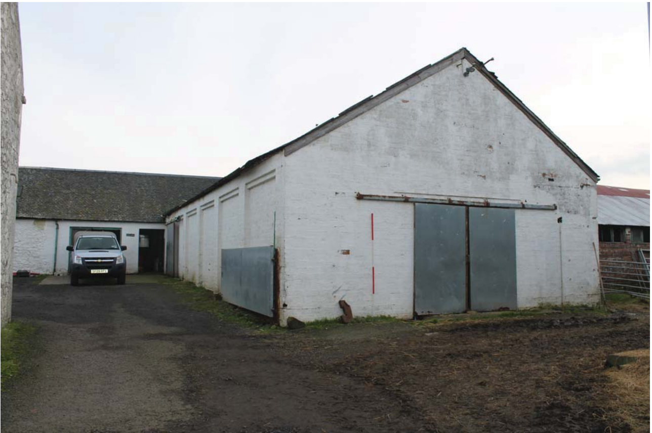
Plate 36: Laigh Corton Farm, Barn D, general view from the west
