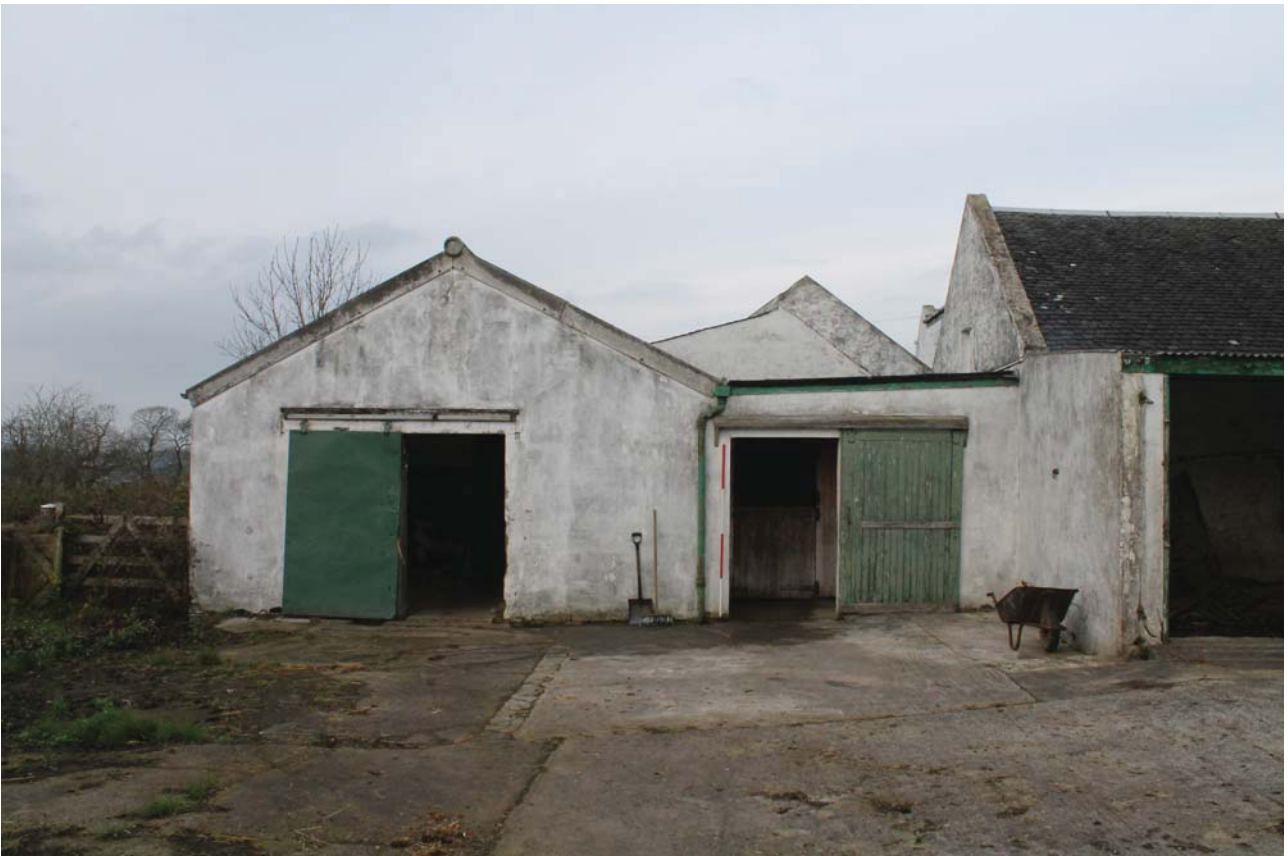
Plate 44: High Corton Farm, Barn B, general view of the south-east gable from the south-east
