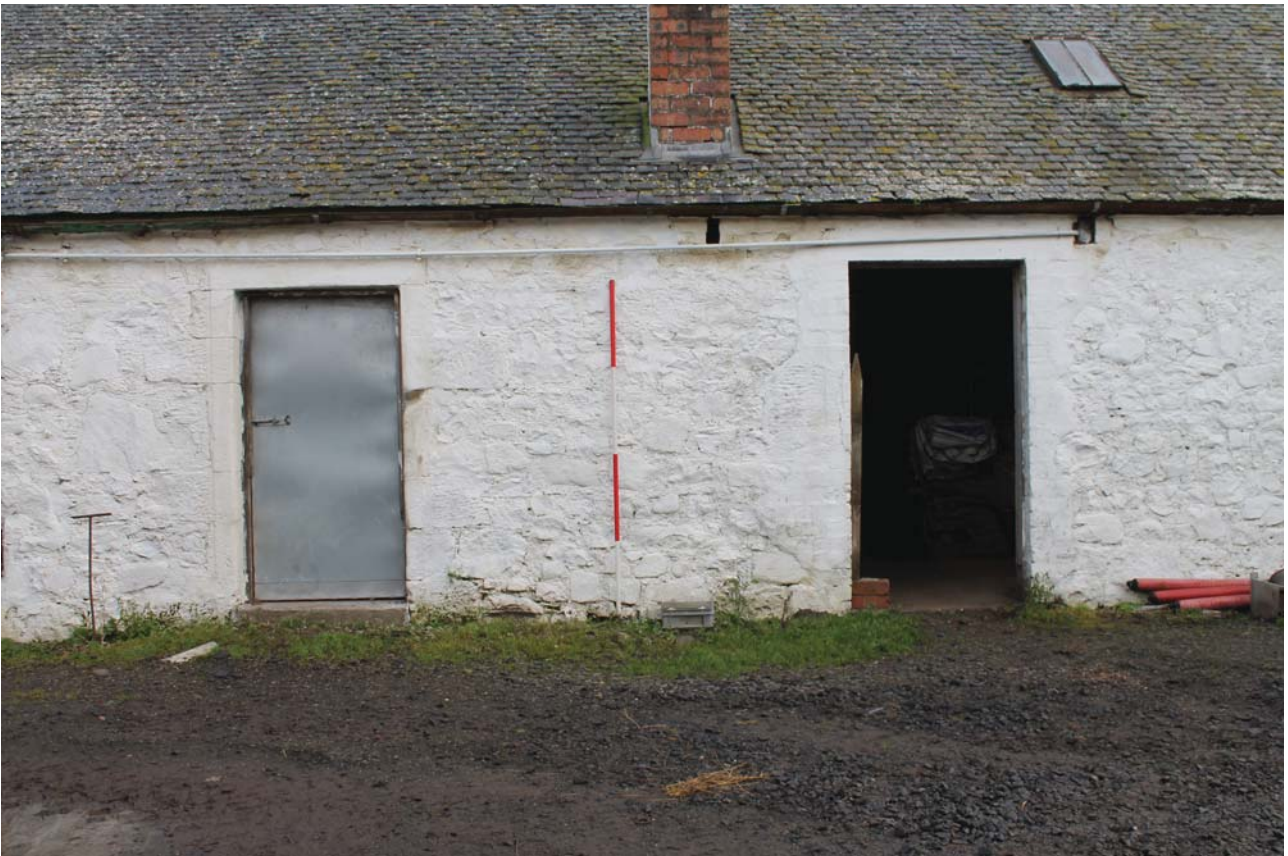
Plate 24: Laigh Corton Farm, Barn C, south-west elevation, detail of doorway and inserted doorway from the south-west
