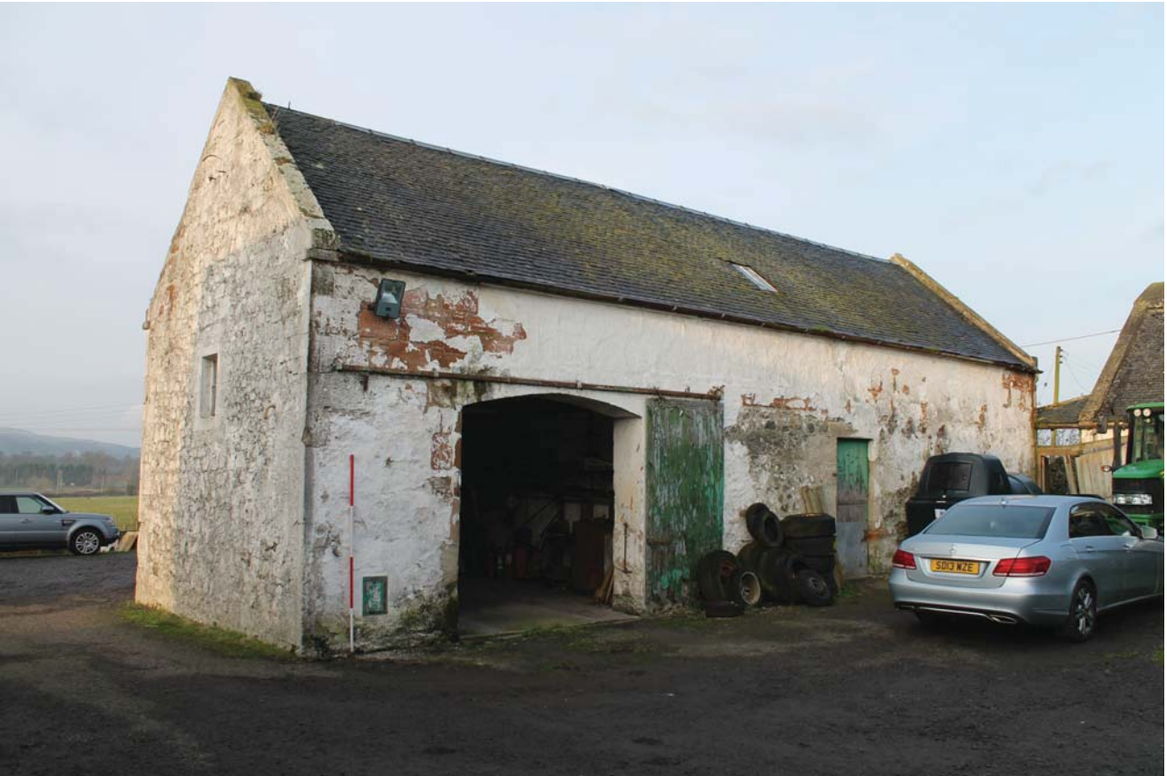
Plate 1: Laigh Corton Farm, Barn A, general view from the east
