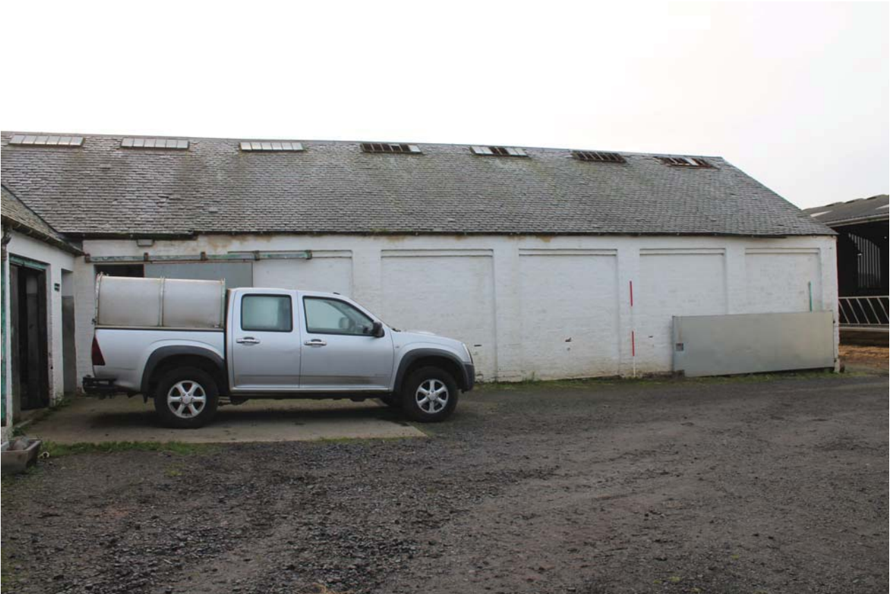
Plate 37: Laigh Corton Farm, Barn D, general view from the north
