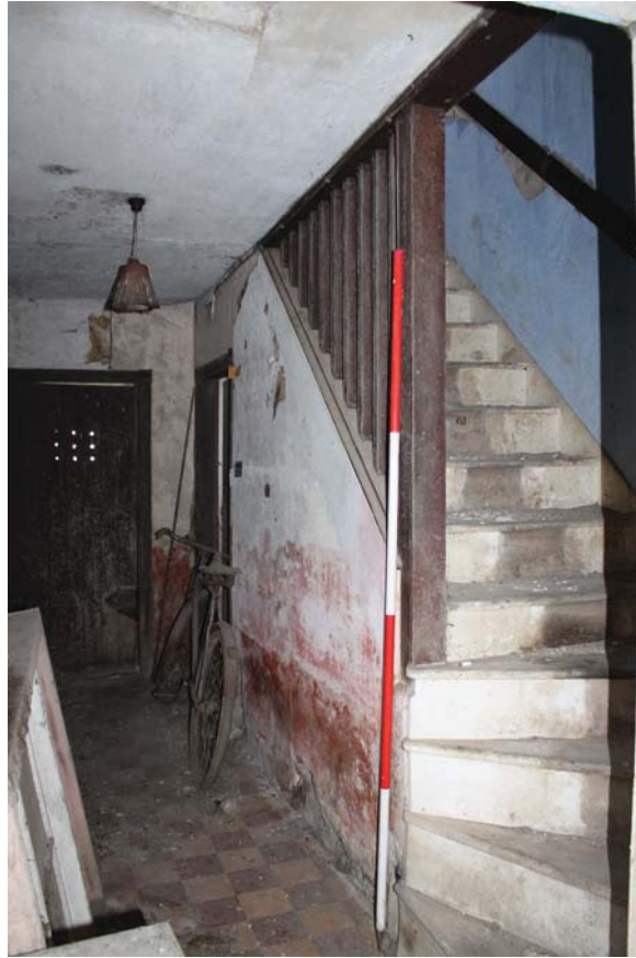
Plate 17: Laigh Corton Farm, Barn B, detail of central stairwell from the south
