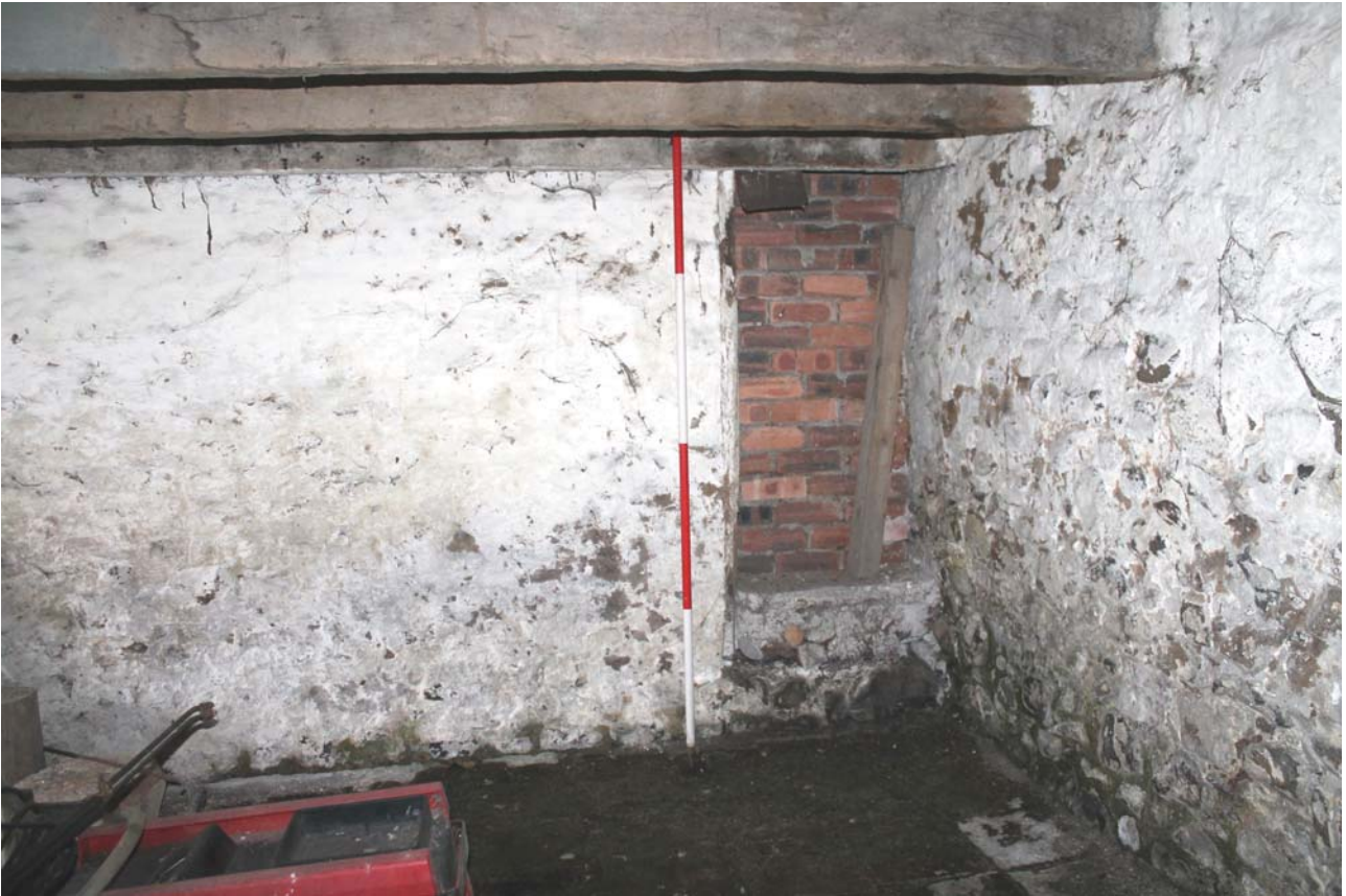
Plate 57: High Corton Farm, Barn C, detail of the bricked-up doorway on the north-east wall of the south-west barn from the west
