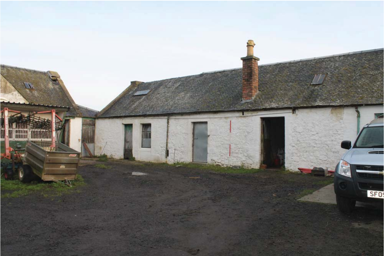
Plate 23: Laigh Corton Farm, Barn C, south-west elevation, general view from the south
