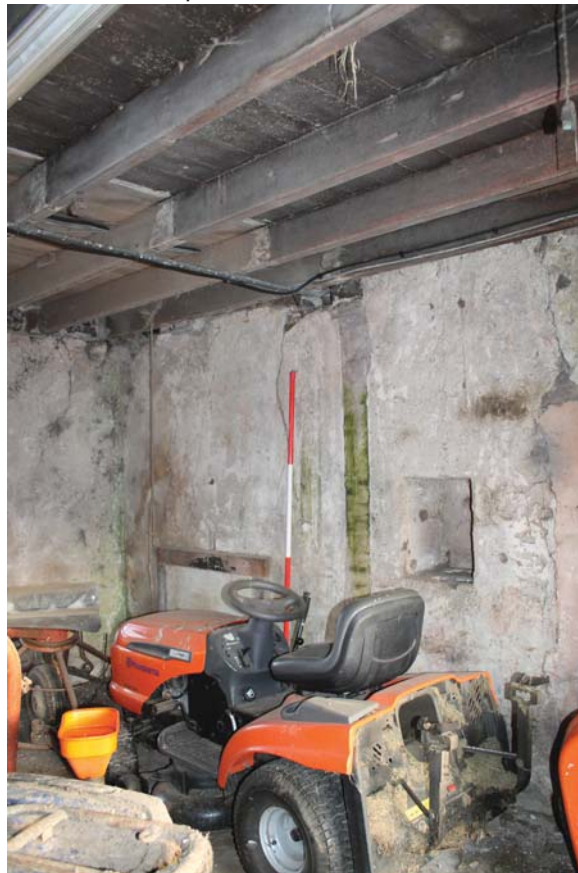
Plate 20: Laigh Corton Farm, Barn B, detail of the ground floor north-westernmost room, showing blocked fireplace from the SSW
