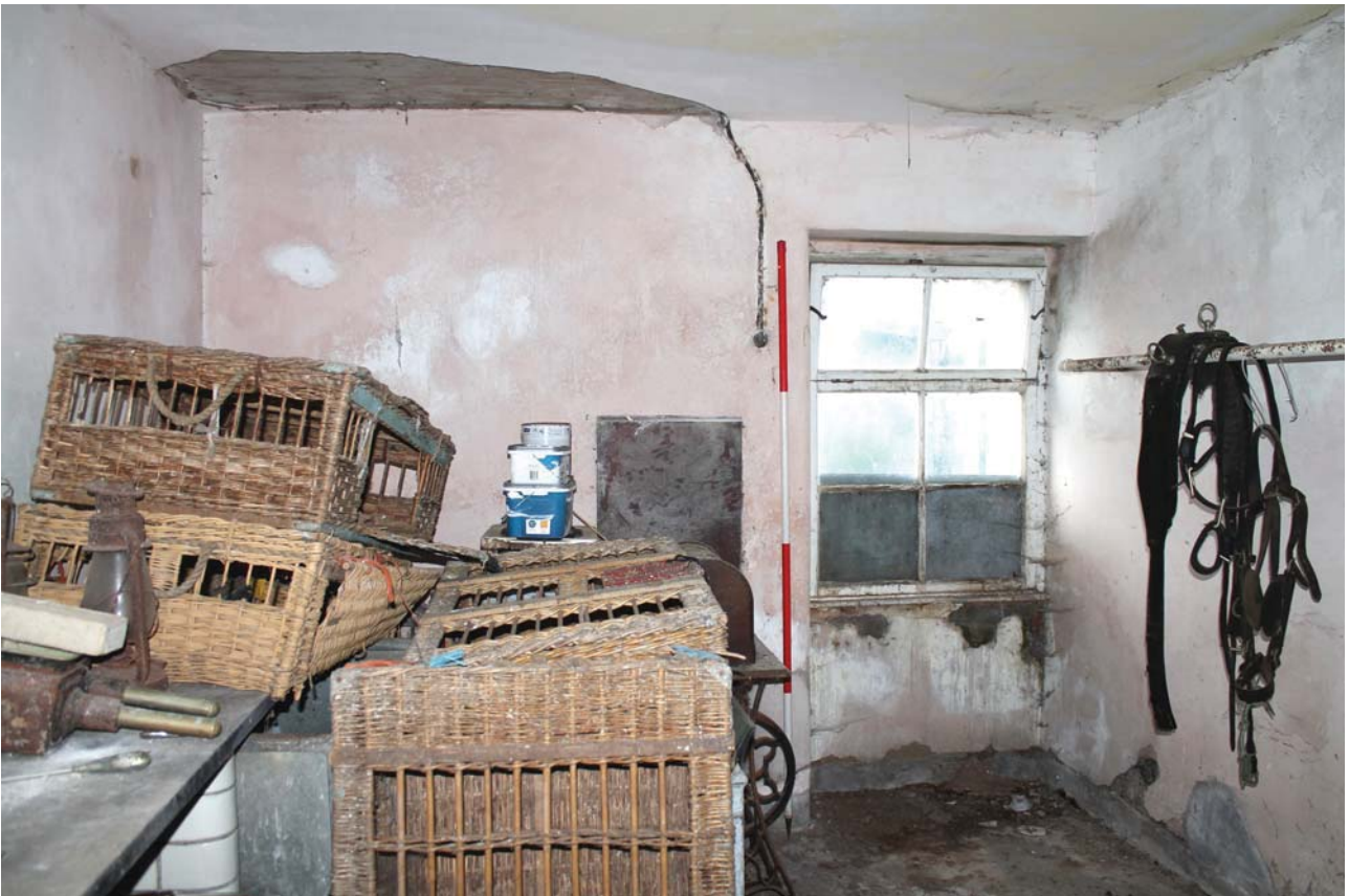
Plate 34: Laigh Corton Farm, Barn C, detail of second from the south-west, from the south-west
