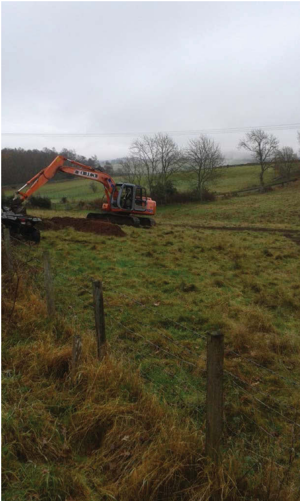
Plate 6 - View of development area from NW corner
