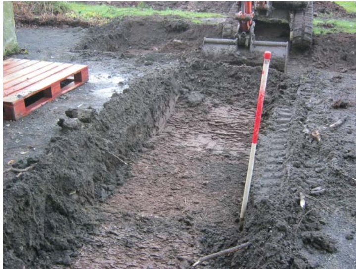
Plate 2. Eastern area of topsoil strip
