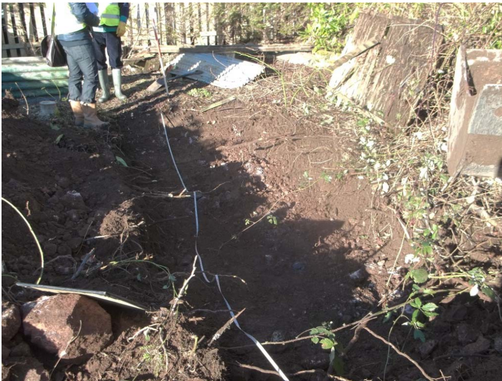
Plate 4 - Post excavation view of Trench 4
