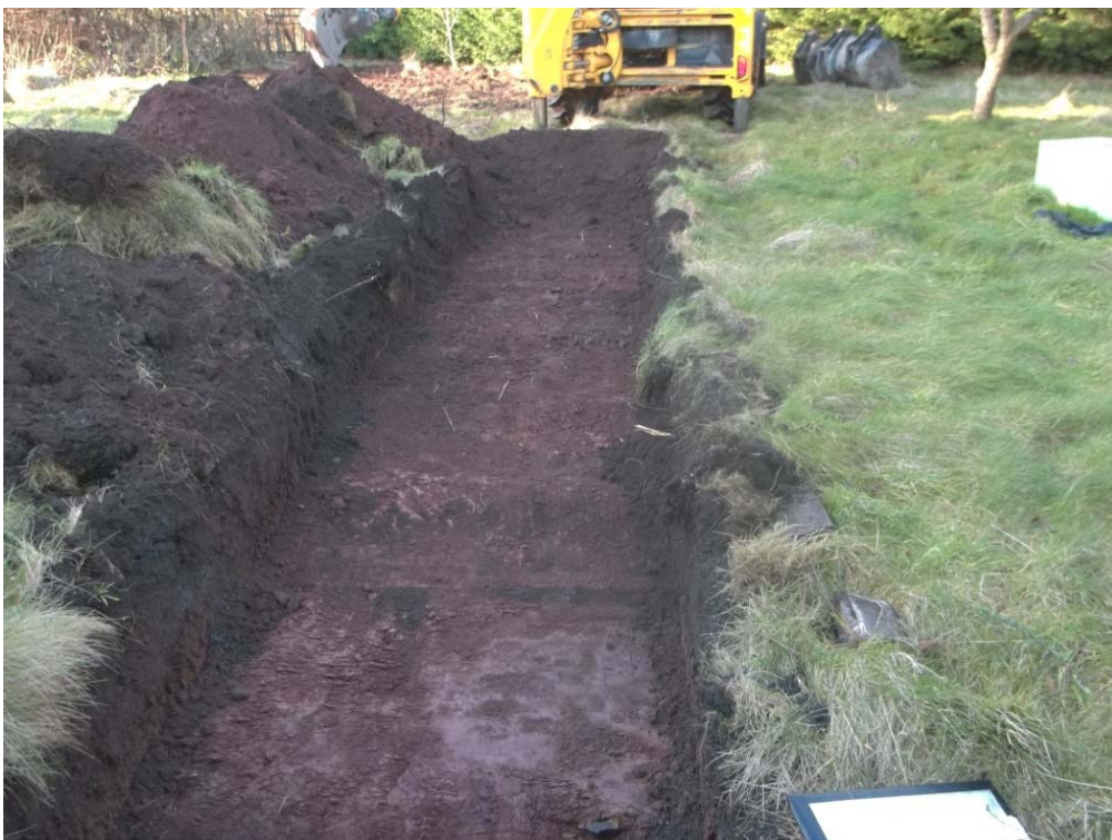
Plate 2 - Post excavation view of Trench 2
