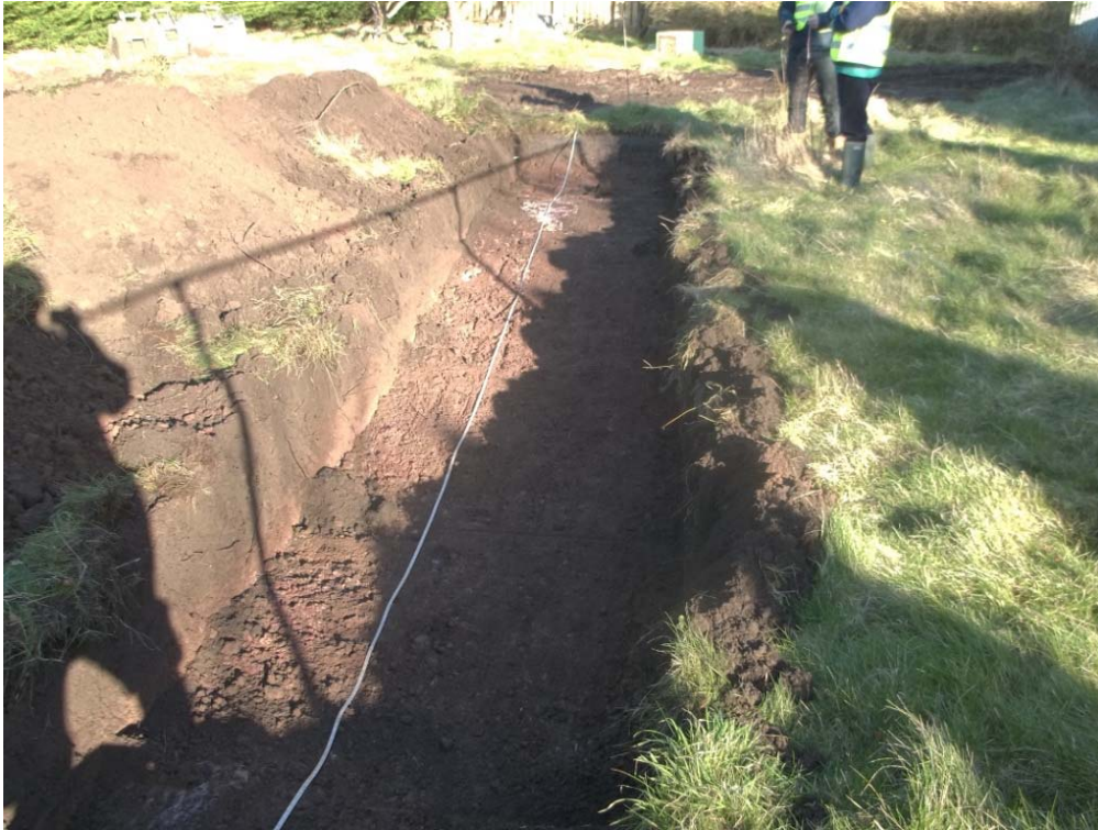
Plate 3 - Post excavation view of Trench 3
