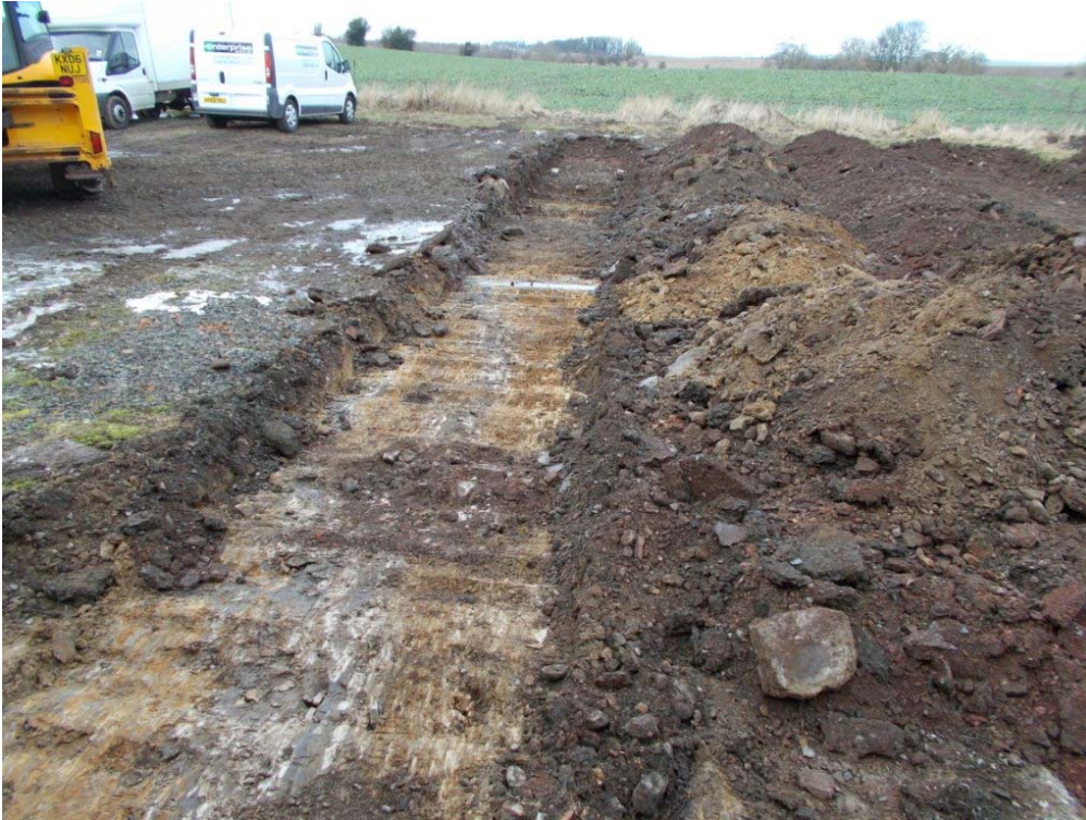
Plate 1 - General view of stripped area showing disturbed clay
