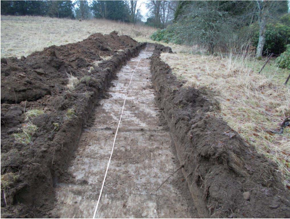
Plate 3 - Post excavation view of Trench 2
