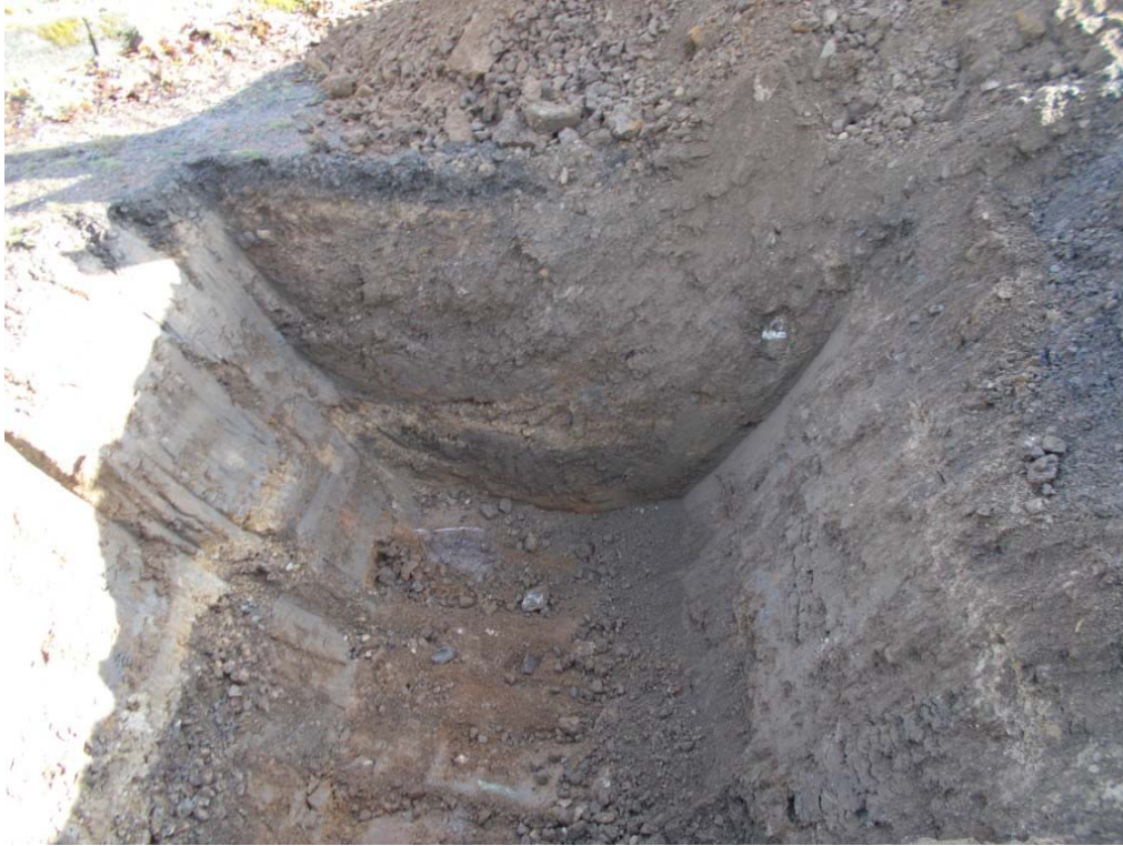
Plate 1 - Made ground within Trench 4
