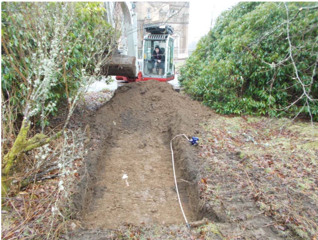
Plate 2 - Location of Trench 3 within bushes
