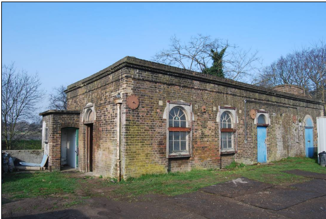
Plate 9: South End of Gas House
