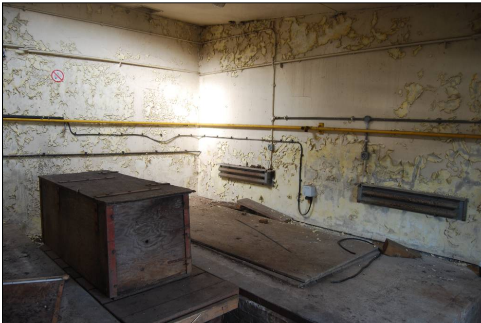
Plate 7: Room 1 Looking Northwest
