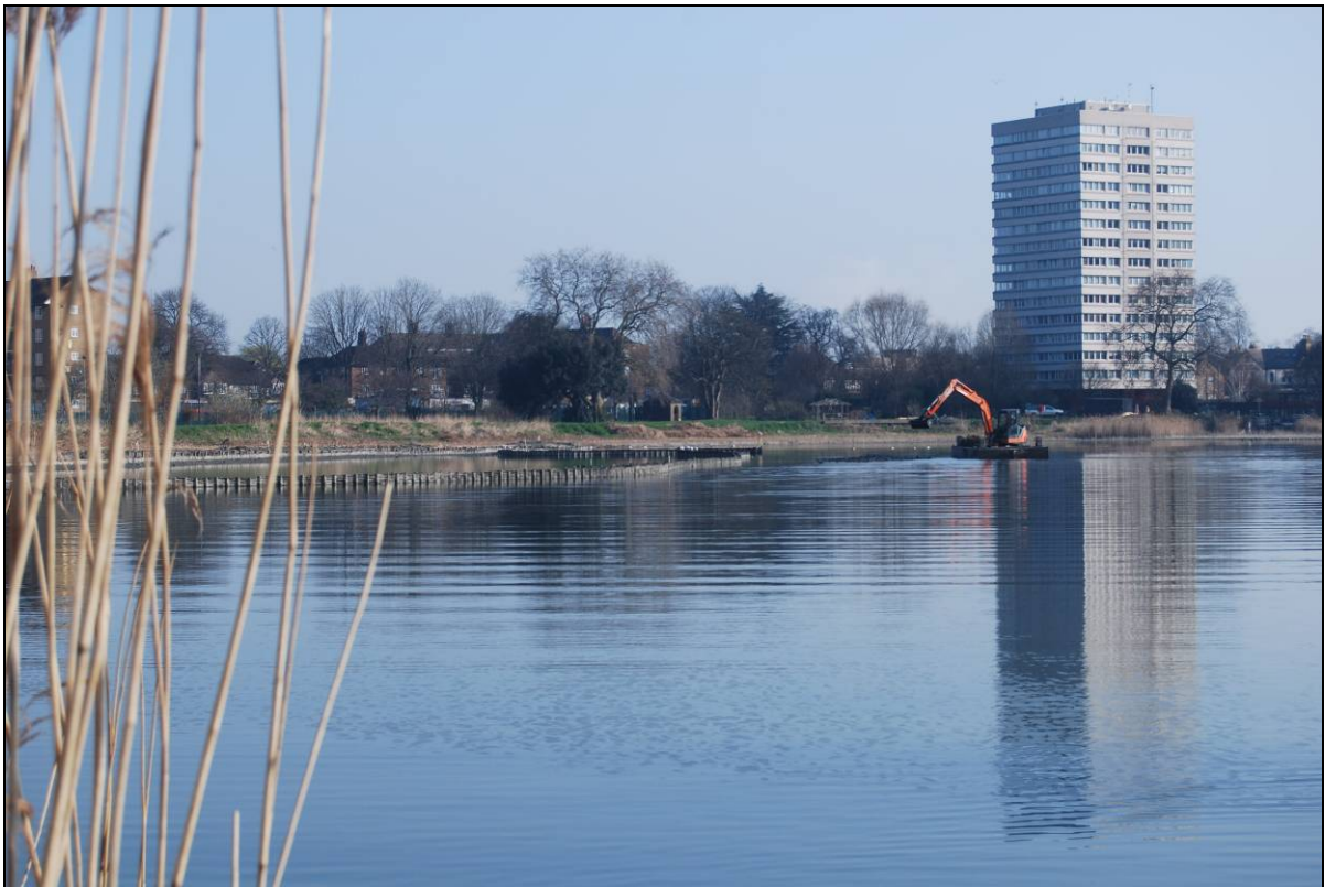
Plate 4: Overview of the Eastern Reservoir, Looking Northeast
