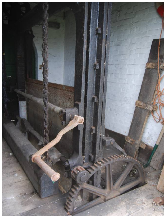
Plate 13: Sluice Mechanism Looking North
