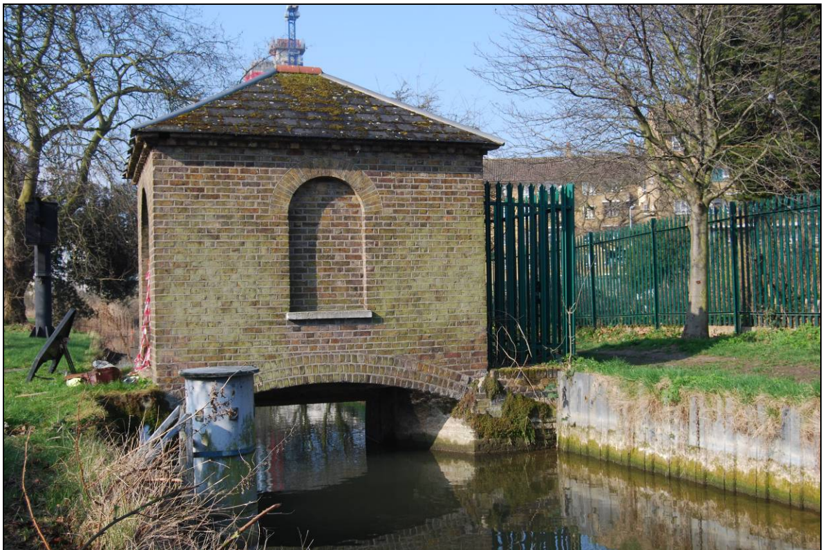
Plate 12: Ivy Sluice Gate House Looking West
