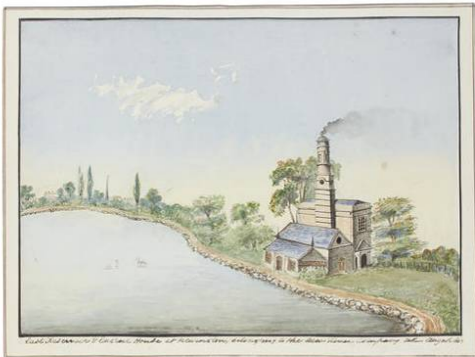
Plate 1: East Reservoir & Engine House at Newington, Belonging to the New River Company taken August 1843
