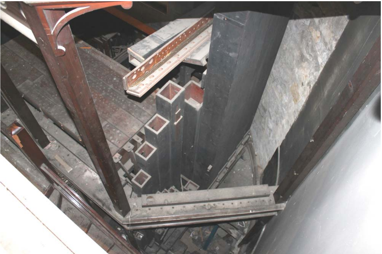
Plate 70: Room 1/1, detail of the top of the timberwork of the piping of the organ from the north
