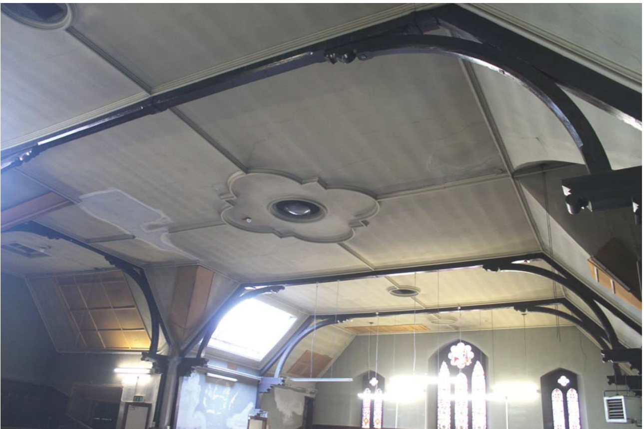
Plate 82: Room 1/1, general view of the ceiling from the south
