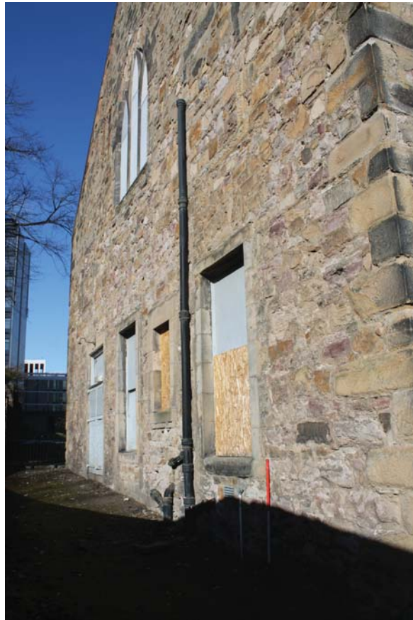
Plate 19: South-west elevation, general view from the south
