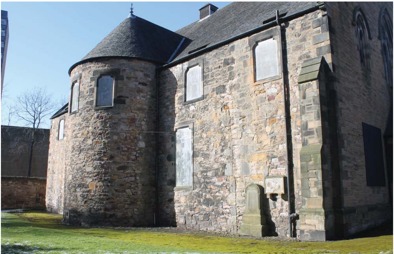
Plate 8: South-east elevation, general view from the east
