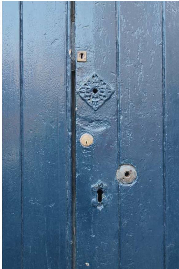
Plate 7: North-east elevation, detail of door fittings from the north-east
