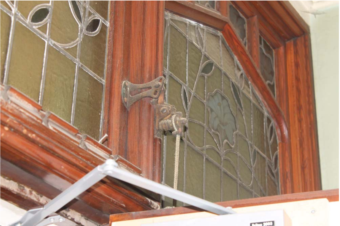
Plate 59: Room 0/4, detail of latch on partition glazing from the west
