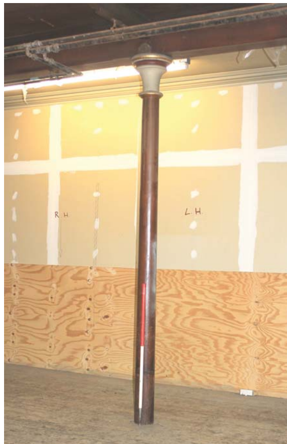
Plate 30: Room 0/1, detail of column from the north
