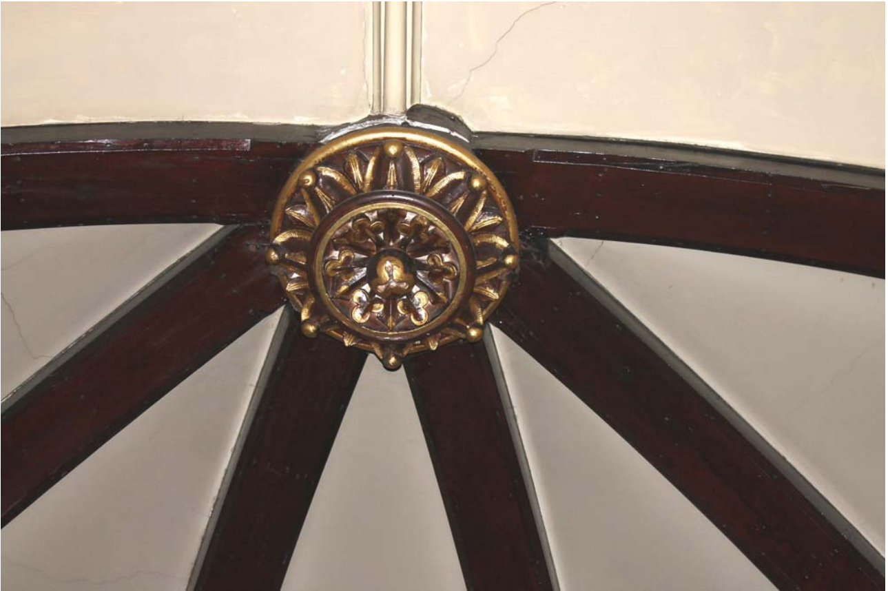
Plate 65: Room 1/1, detail of boss above organ bay from the north-west
