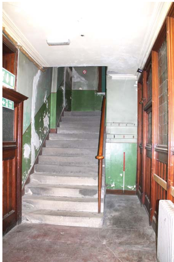
Plate 56: Room 0/4, general view of the stairwell from the south-east
