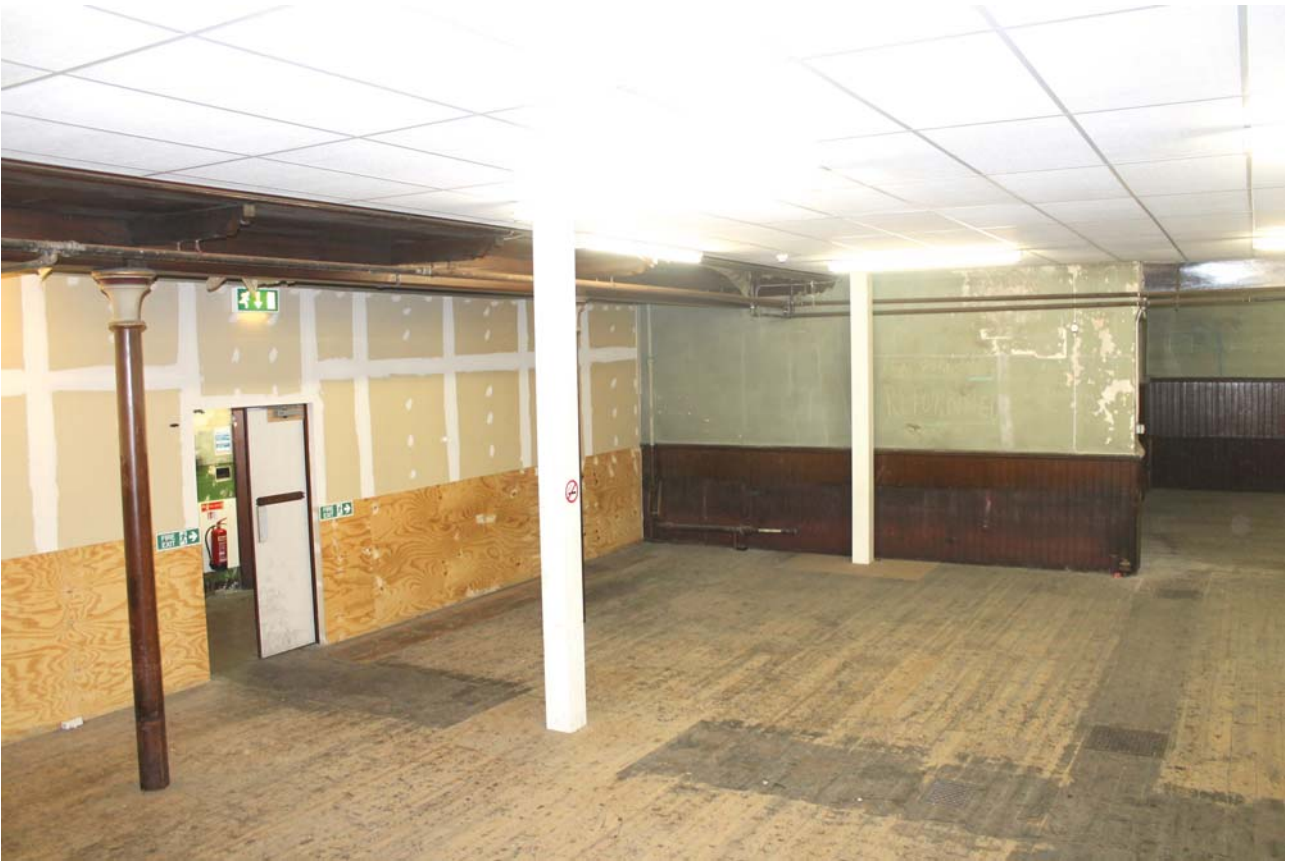
Plate 27: Room 0/1, general view from the east
