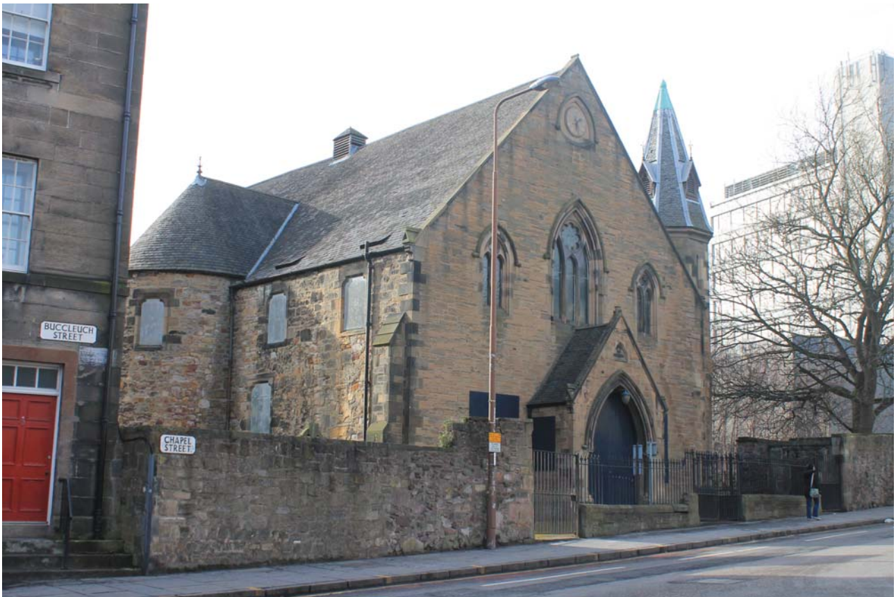
Plate 1: General view from the east
