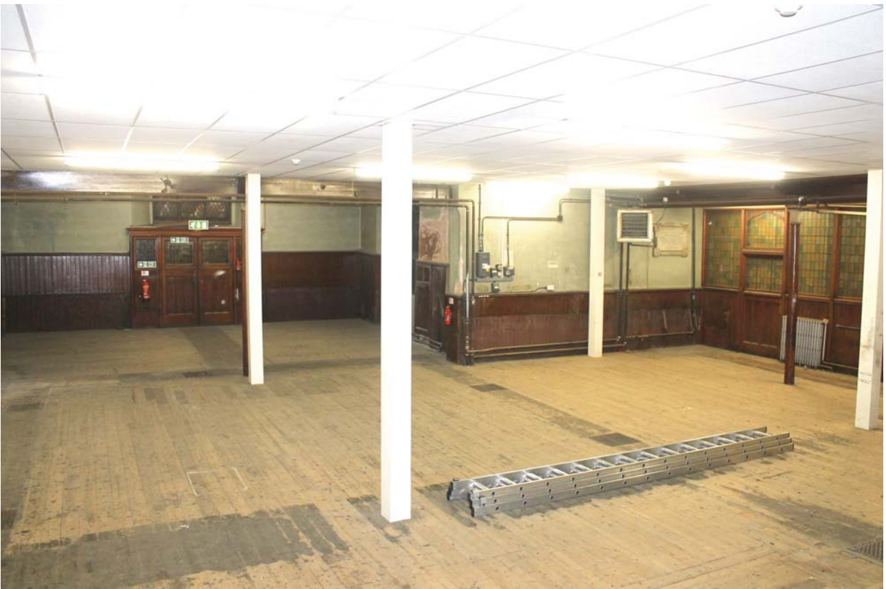
Plate 26: Room 0/1, general view from the south
