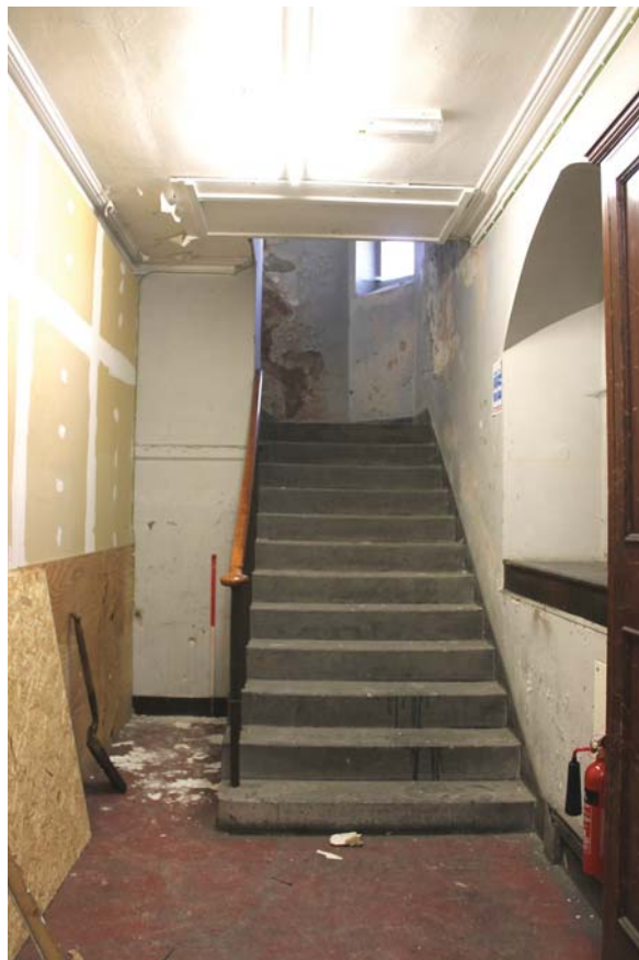
Plate 52: Room 0/2, general view showing stairs from the south-east
