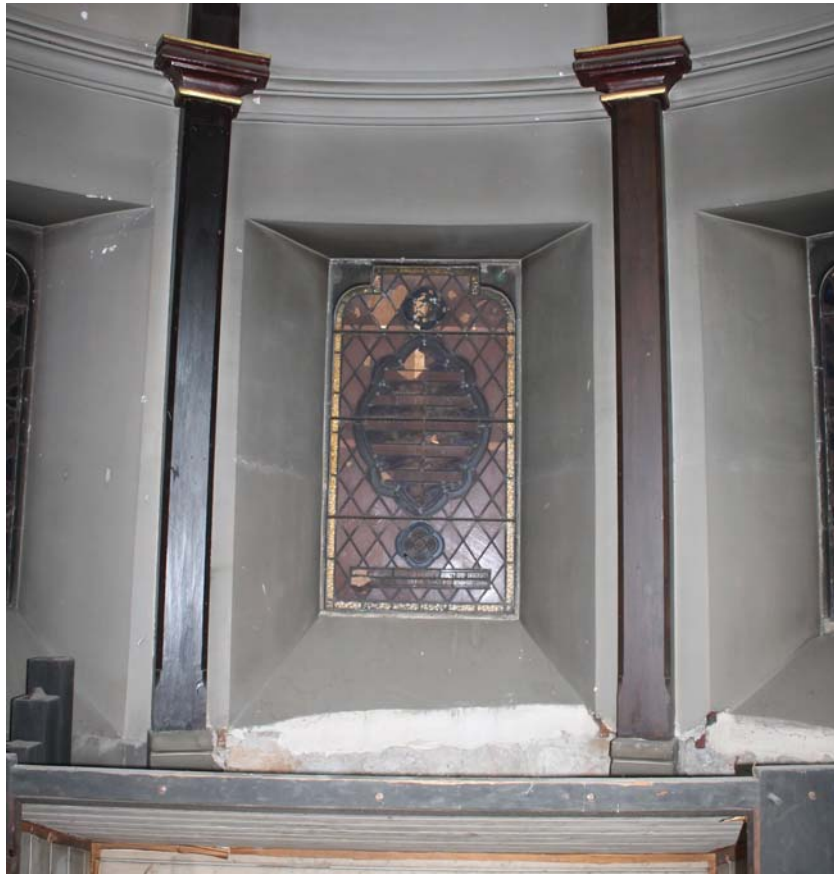
Plate 67: Room 1/1, detail of window in the organ bay from the north-west
