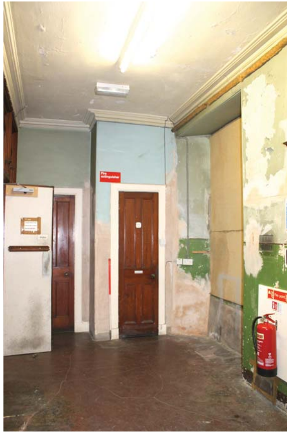
Plate 57: Room 0/4, general view from the north-west
