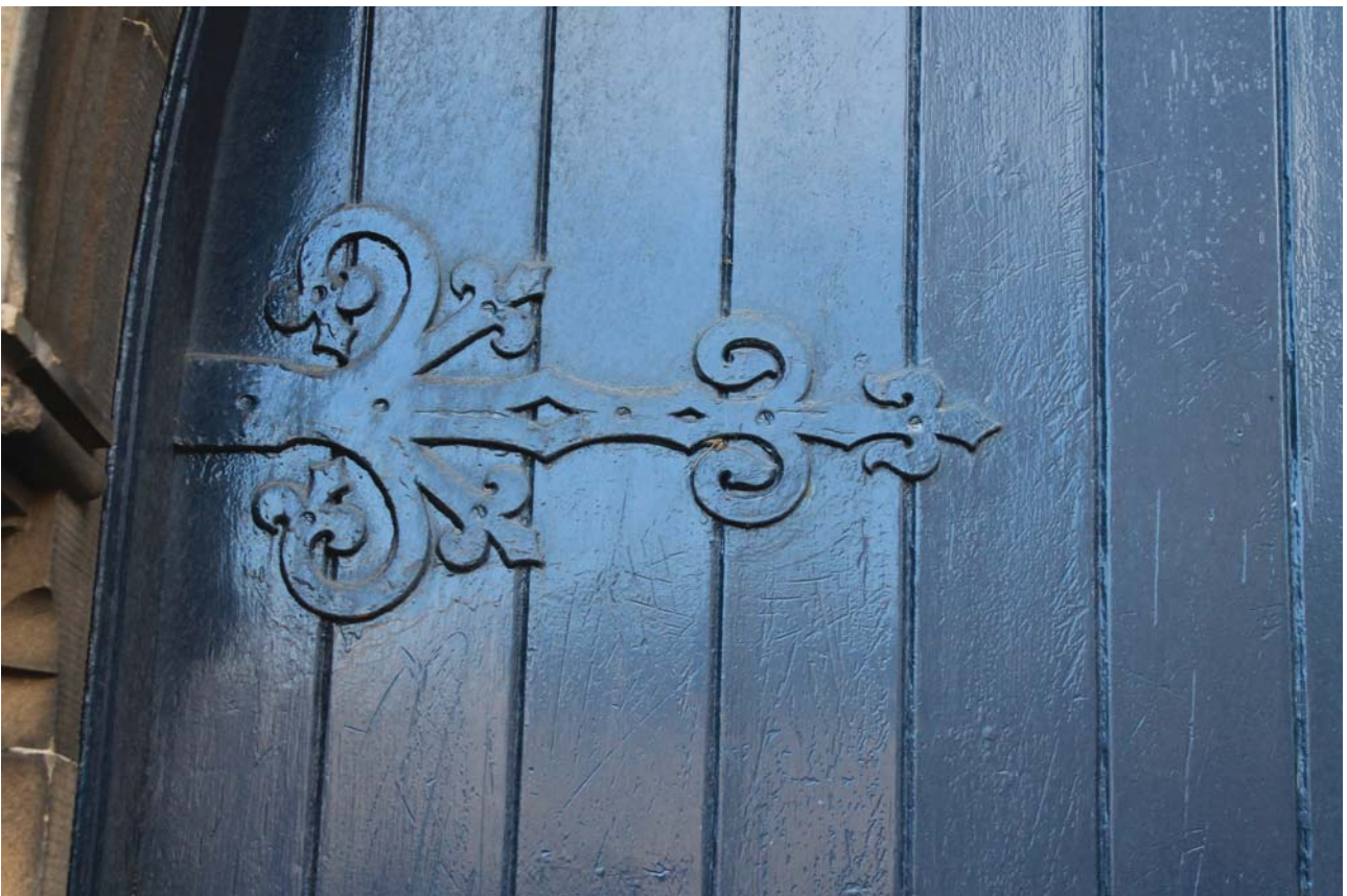
Plate 6: North-east elevation, detail of door hinge from the north-east
