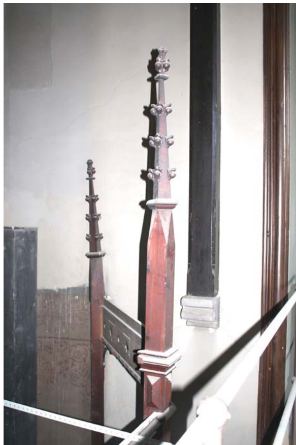
Plate 68: Room 1/1, detail of timberwork to the top of the organ from the north
