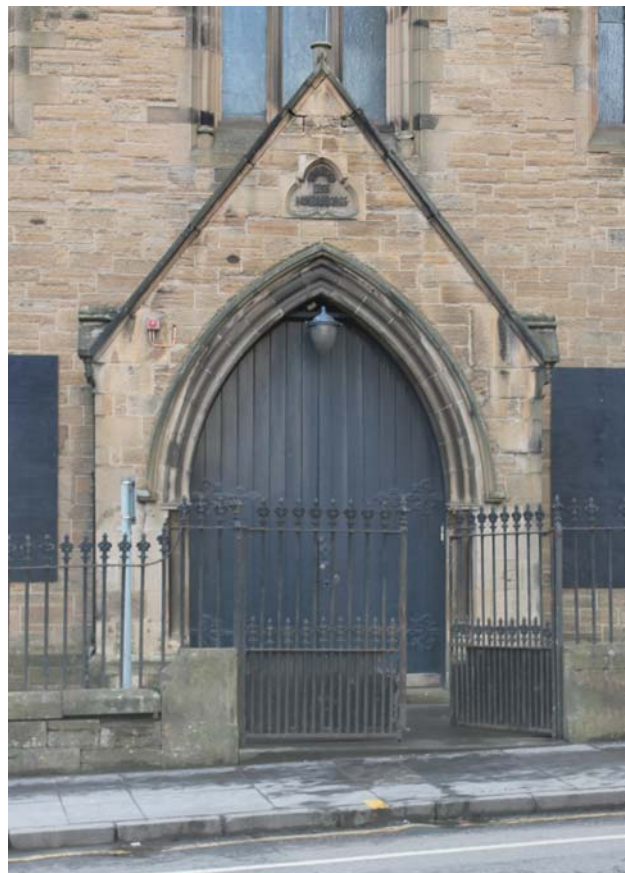
Plate 2: North-east elevation, detail of porch from the north-east
