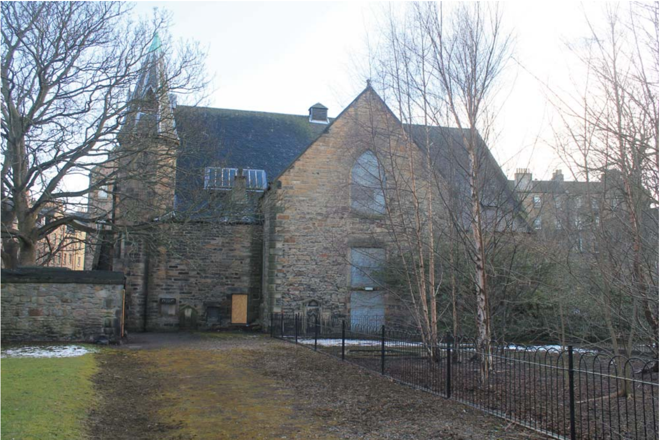
Plate 13: North-west elevation, general view from the NNE
