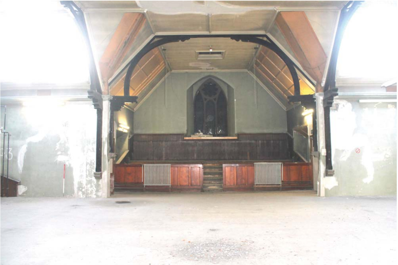
Plate 75: Room 1/1, general view of the north-west transept from the south-east
