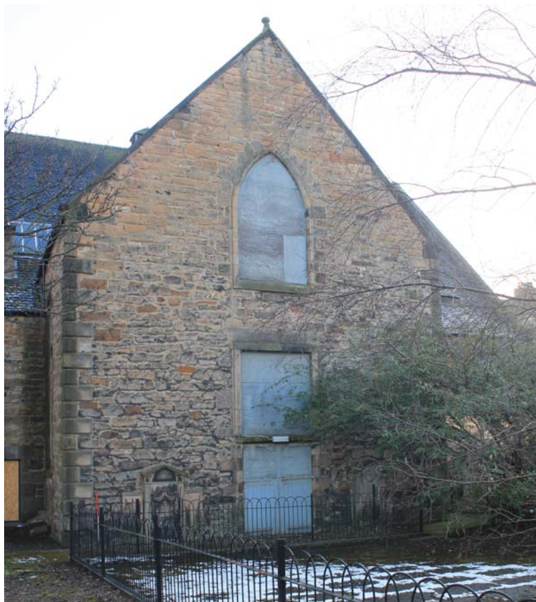
Plate 14: North-west elevation, detail of north-west transept, from the NNE
