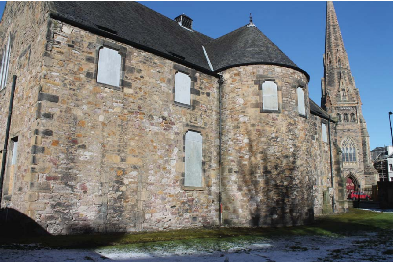
Plate 9: South-east elevation, general view from the south
