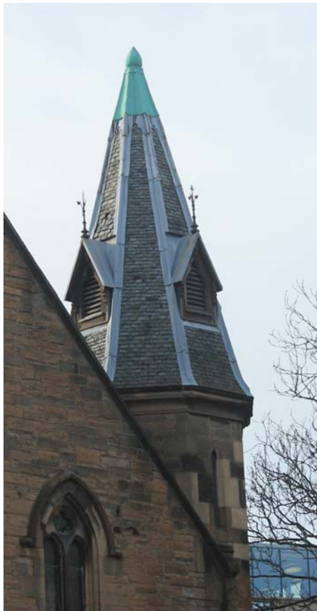
Plate 18: Detail of the north tower from the east
