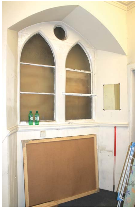
Plate 55: Room 0/3, detail of window in the north-east wall from the west
