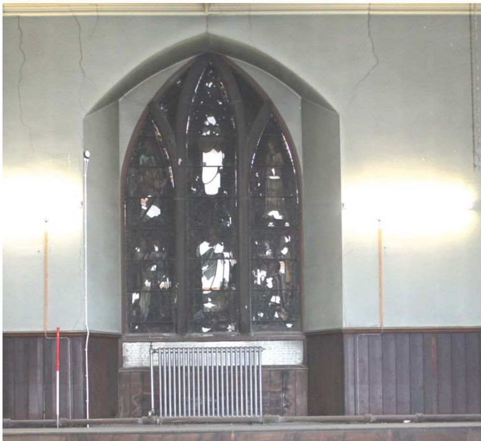
Plate 74: Room 1/1, detail of window in the north-east wall from the north-east
