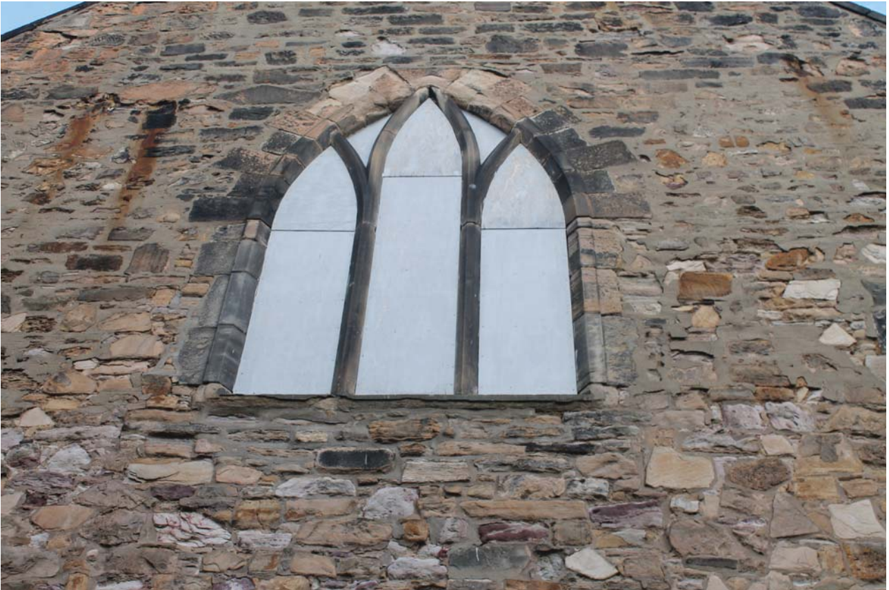
Plate 25: South-west elevation, detail of first floor central window from the south-west
