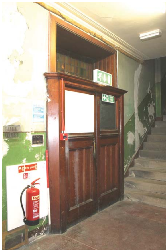
Plate 60: Room 0/4, detail of main doorway from the east
