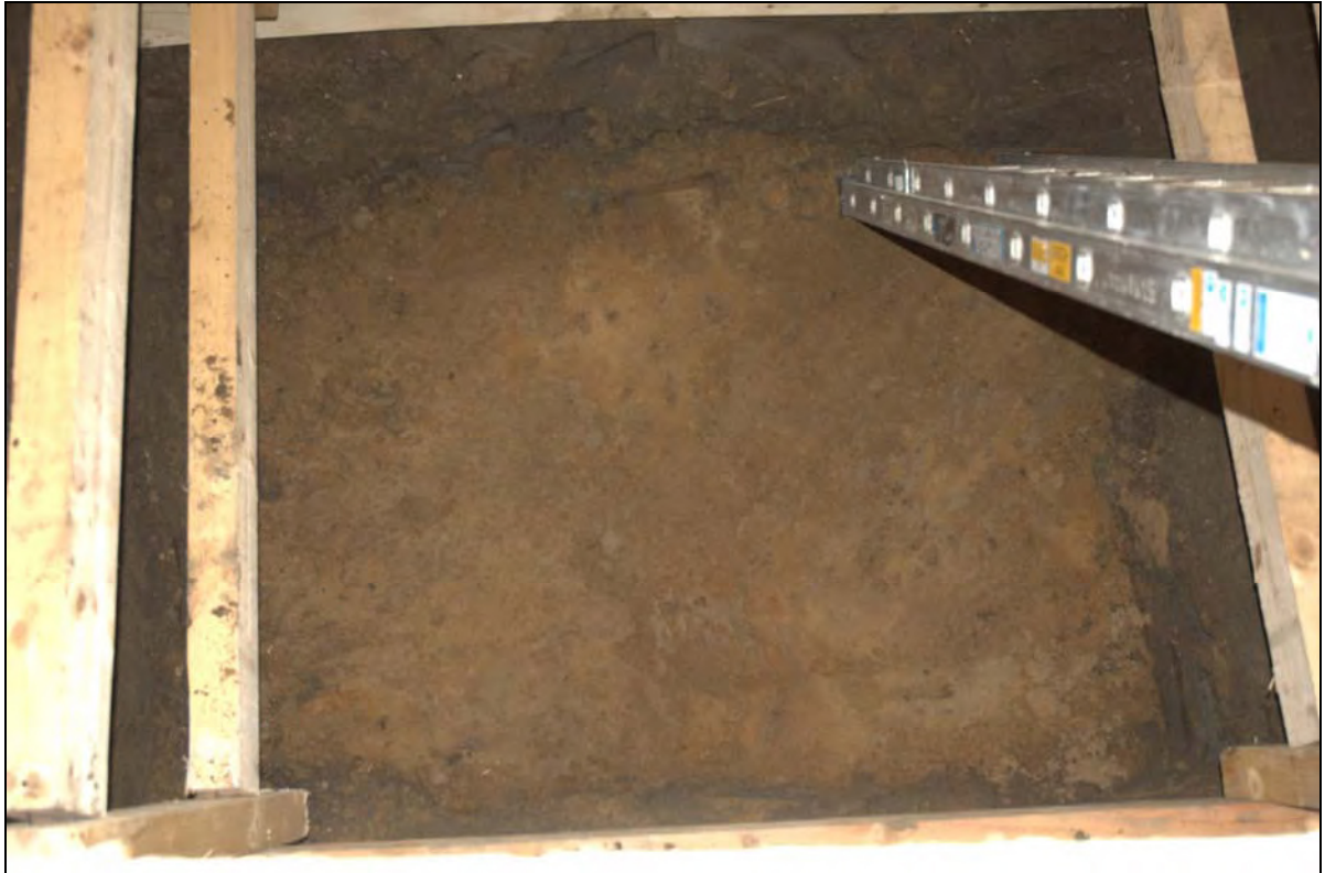
Plate A: Base of Trench looking south
