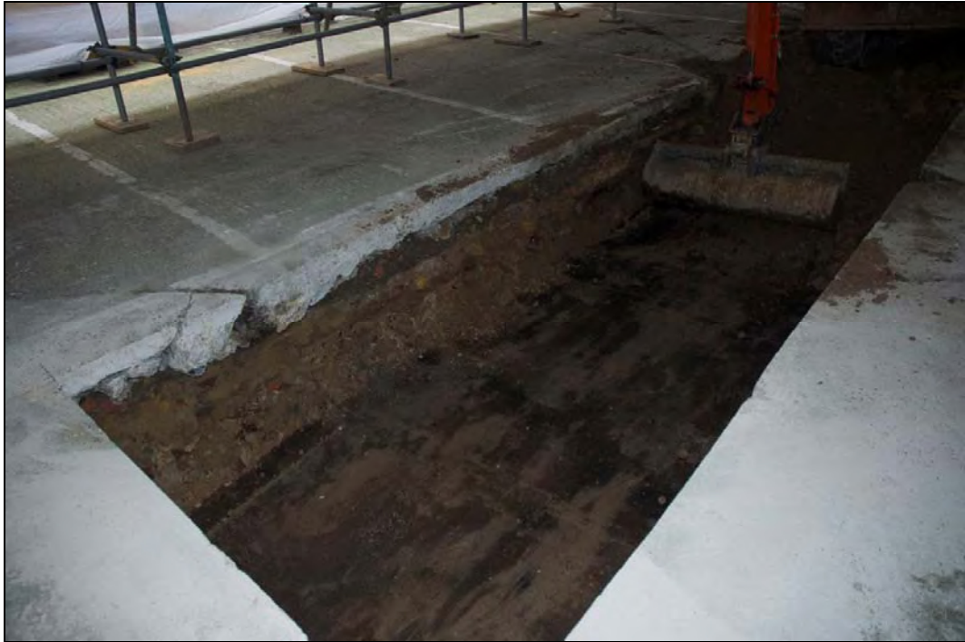
Plate B: Surface (102) during excavation, looking west
