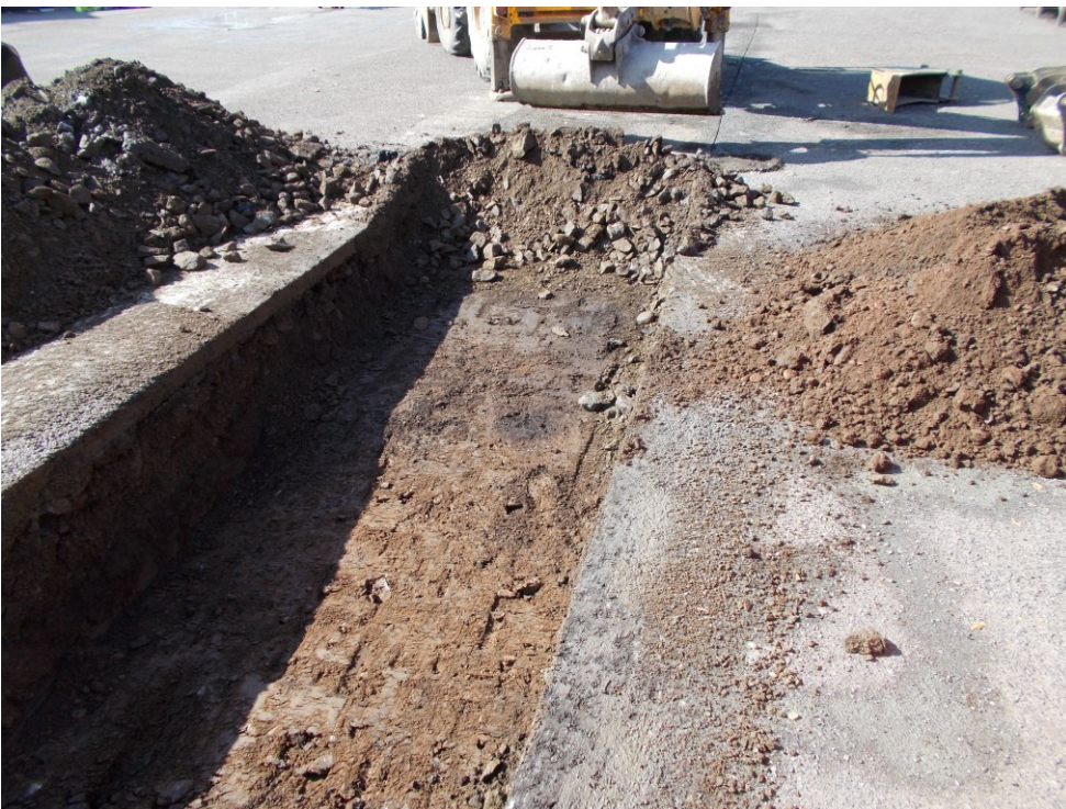
Plate 2: Exterior foundation trench running NW-SE
