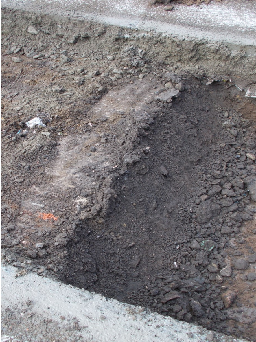
Plate 3: Interior foundation trench running NW-SE
