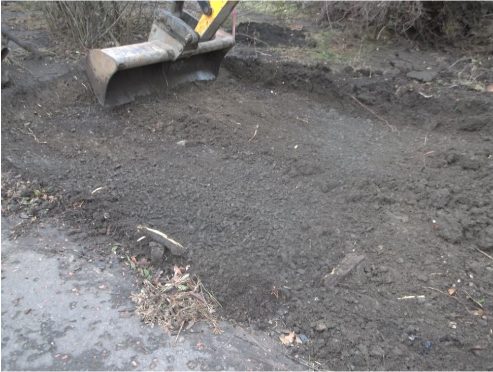
Plate 1: Pre excavation shot removing tarmac
