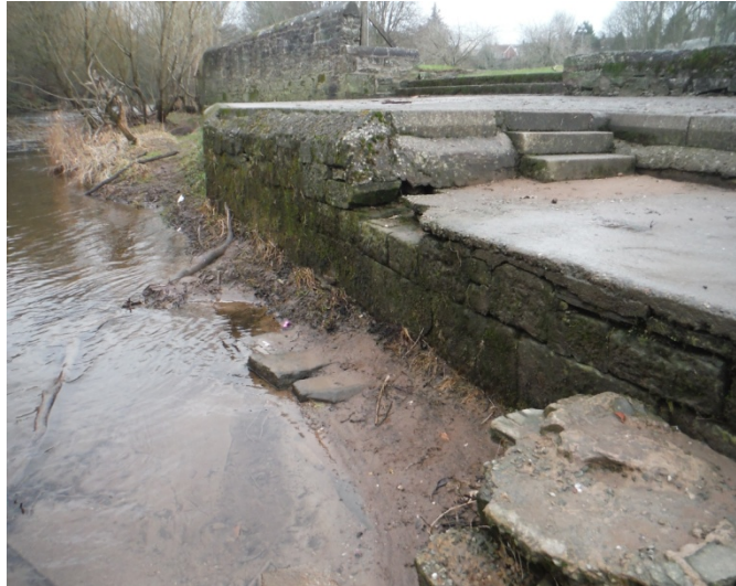
Plate 1 Zone 1 The Mooring Area from west
