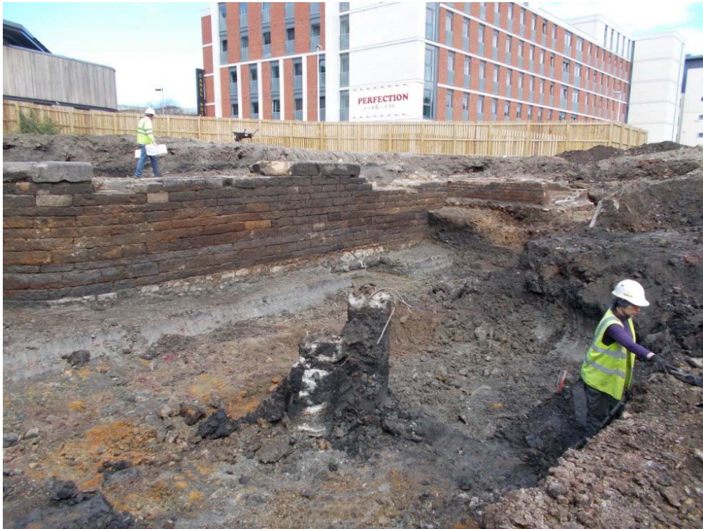
Plate 1 - Concrete piles within basin fill
