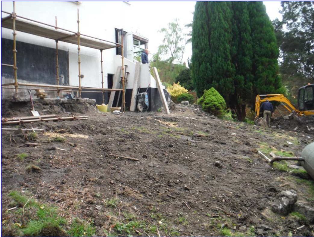
Plate 1: General view of the site (pre-excitation)
