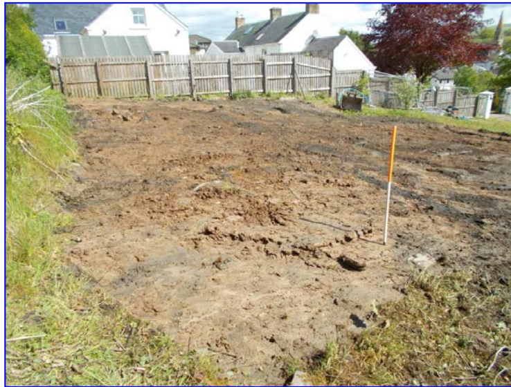
Plate 1: General view of stripped development area showing disturbance
