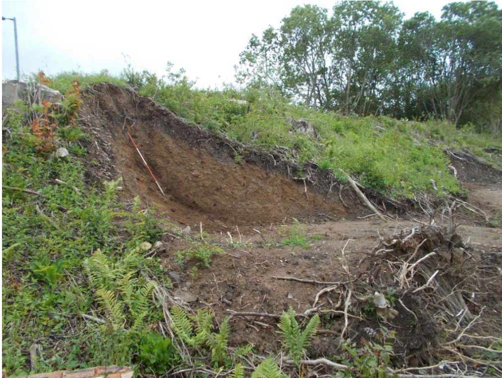
Plate 3 - General view of embankment cut
