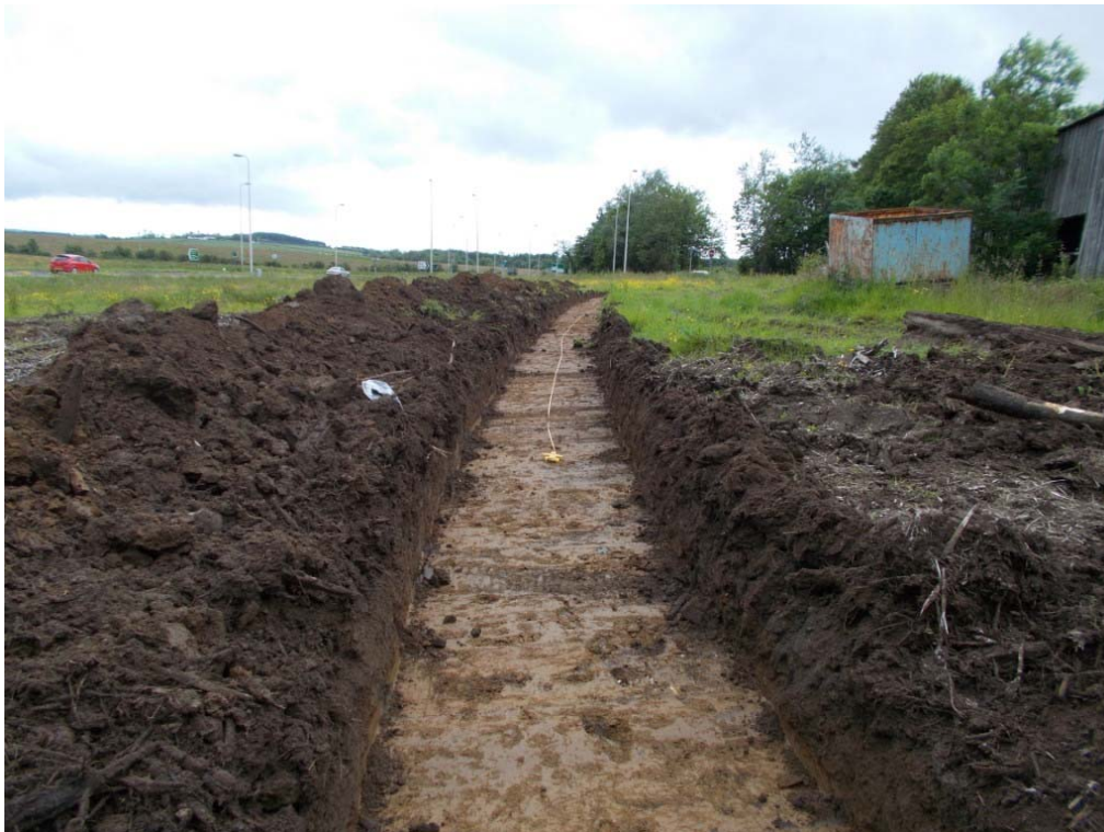
Plate 2 - Post excavation view of Trench 6
