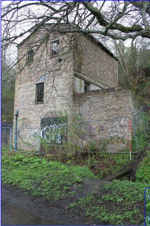
Plate 2: North elevation, general view from the north-west
