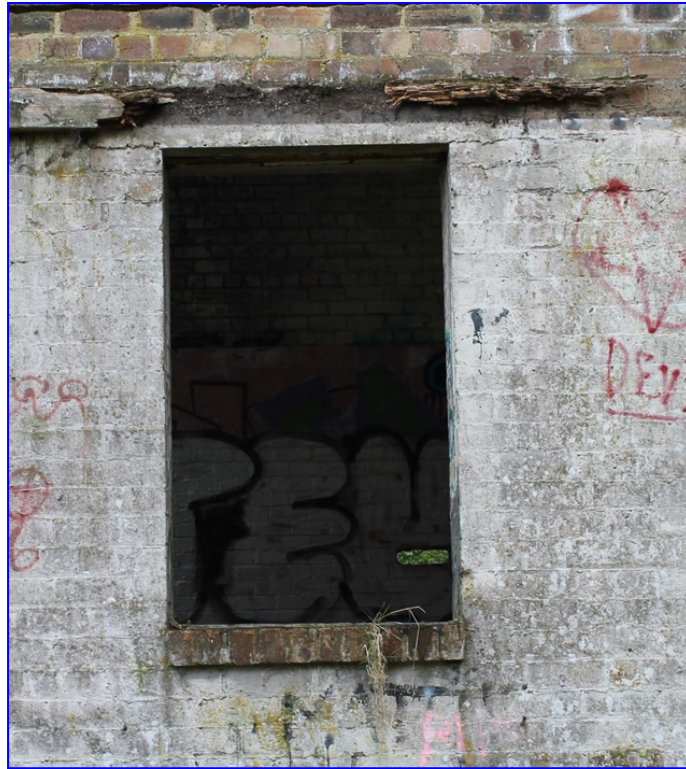
Plate 6: West elevation, detail of the ground floor window from the west
