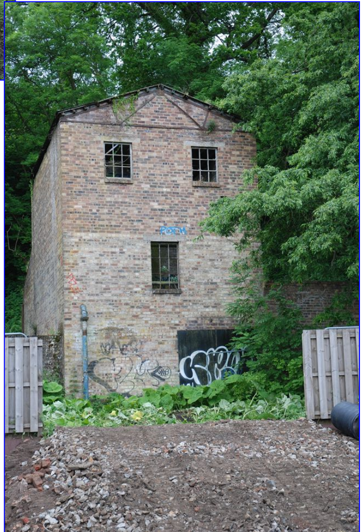
Plate 3: North elevation, general view from the NNE just prior to demolition
