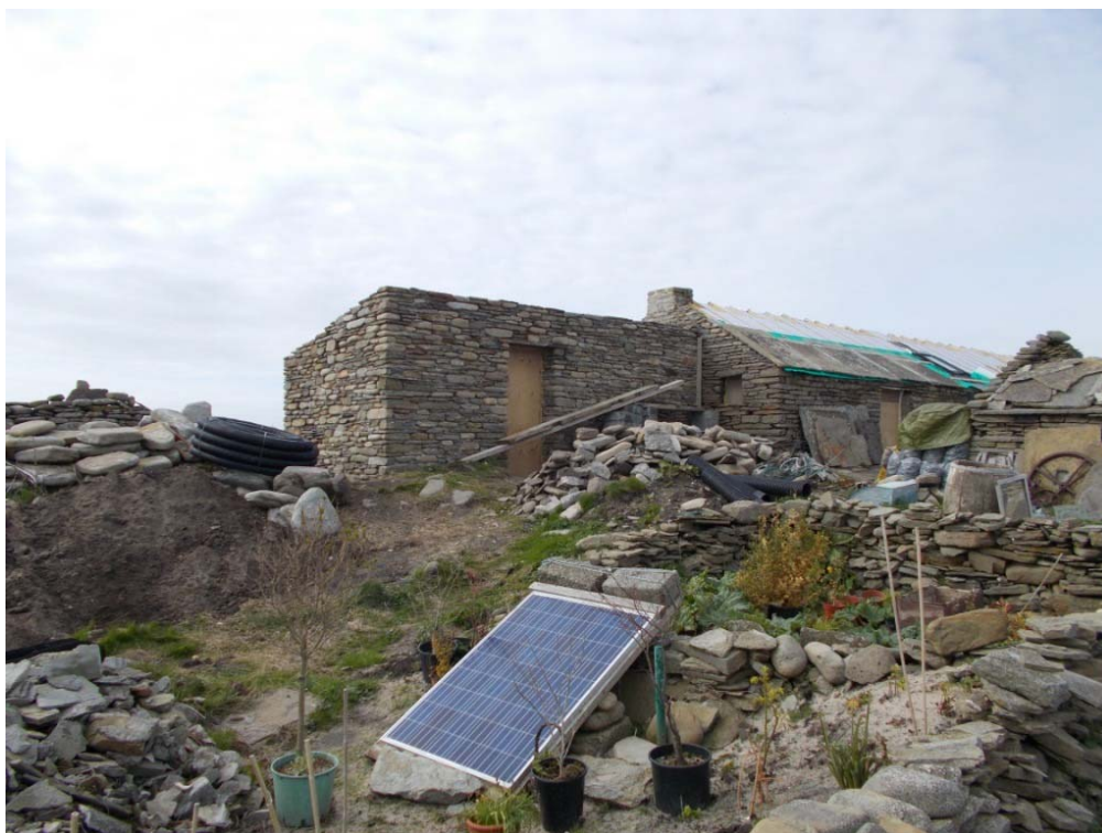
Plate 1 - General view of plant room at S end of Mayback
