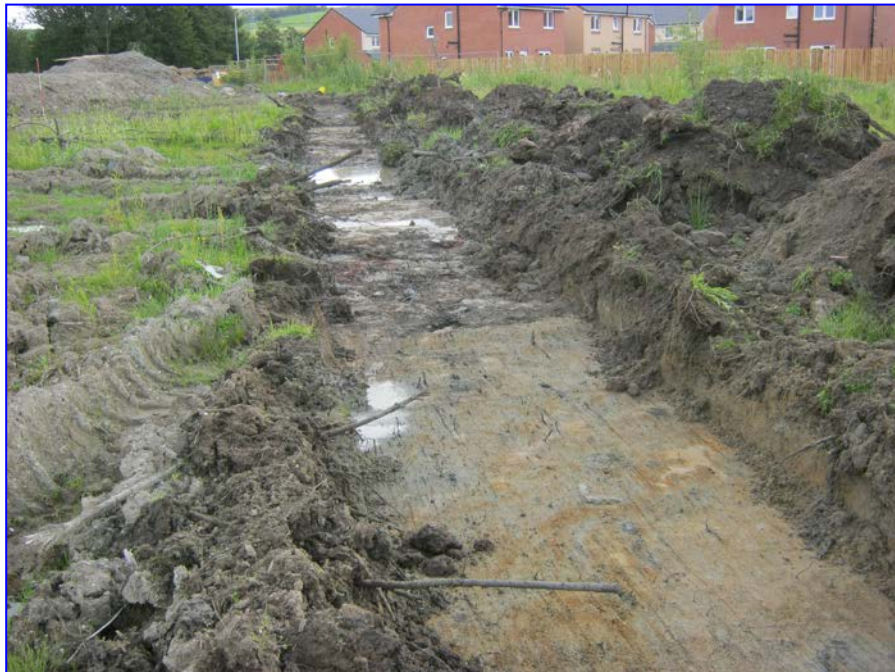
Plate 1: Trench 1, general post-excitation view from the south-west
