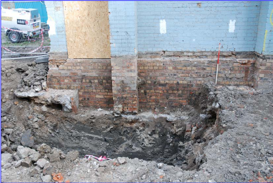
Plate 13: General view of excavations during the later watching brief in the area of Test Pit 7 showing the rubble deposits and features (now removed) resting over the highly compact black clay deposit (002)
