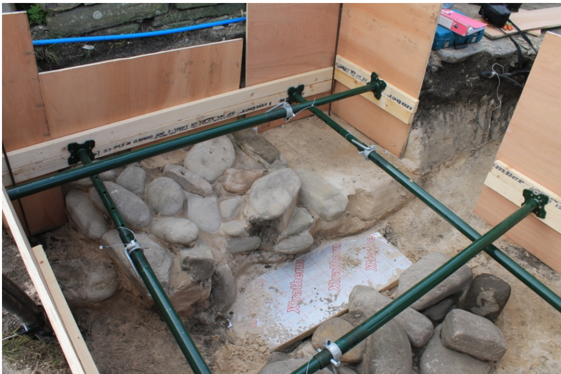
Plate 1 – Shoring in place around trench
