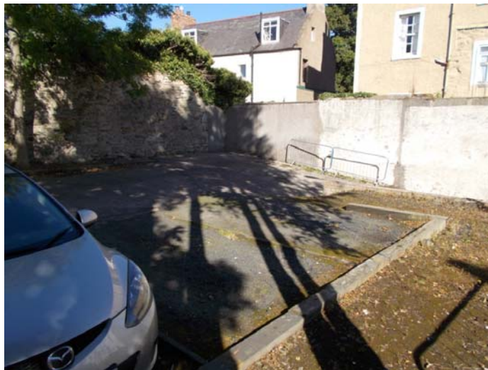
Plate 1 – View of concrete slab and car in Union Street car park
