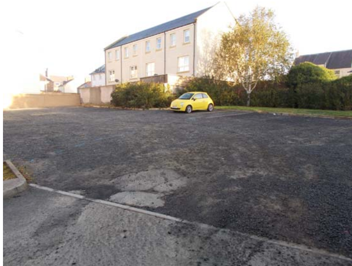
Plate 2 - View of car parked in Roxburgh Street
