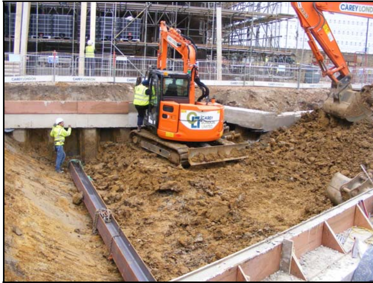
Plate 2: General shot of excavation area, looking south
