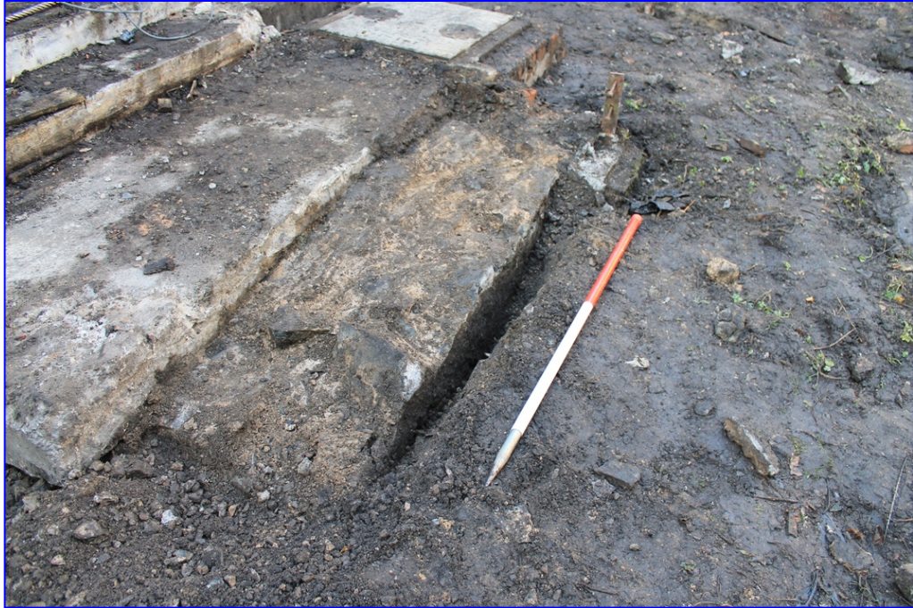
Plate 3: Remnants of stone wall [002] first exposed beneath and to the north of the concrete step to the east of the plot, from the north-east
