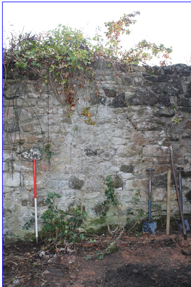
Plate 8: Detail of the boundary wall to the east side showing the mortar scar of the former position of the boundary wall, from the west
