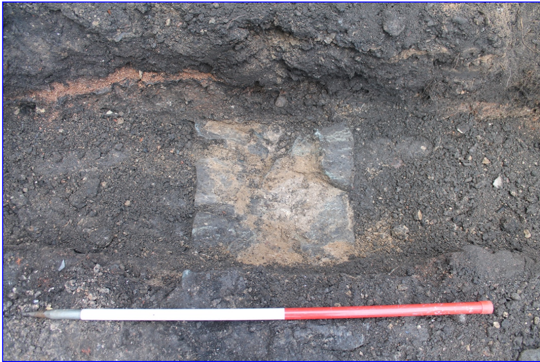
Plate 7: Small section of wall [002] exposed in the western foundation trench for the new extension from the east
