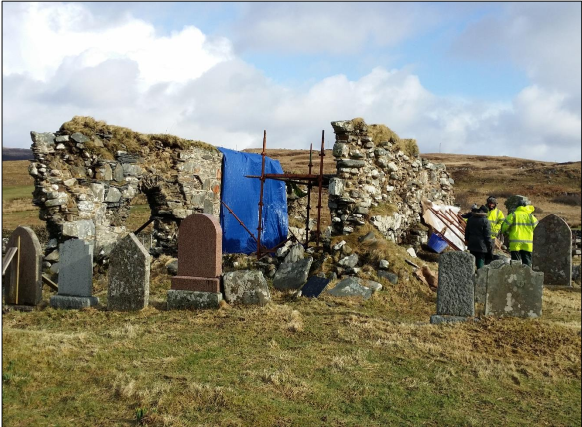
Plate 1: Kilvickeon Church, during the 2015 conservation works
