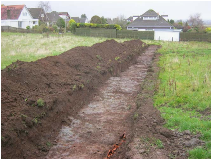
Plate 1: Trench 4 showing boulder clay and deposits of tarmac and concrete.
