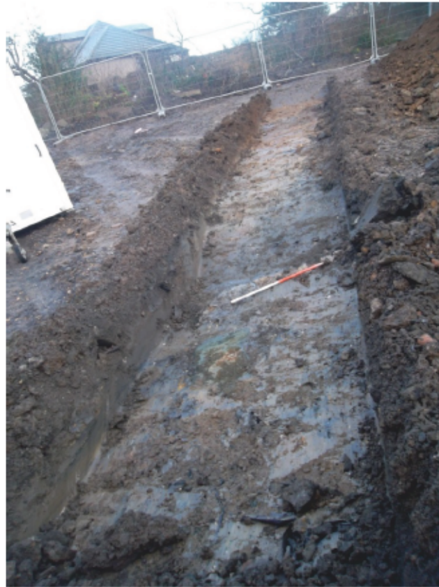
Plate 1: Trench 1: Post excavation
