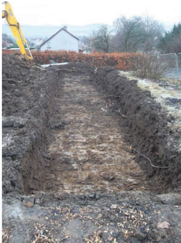
Plate 2: Trench 4: Post excavation
