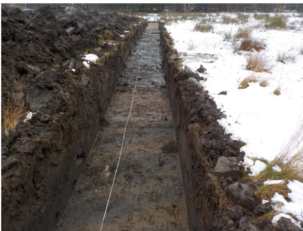
Plate 2 - Post excavation view of Trench 4
