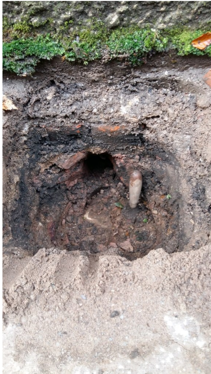
Plate 2 - View of foundation pit
