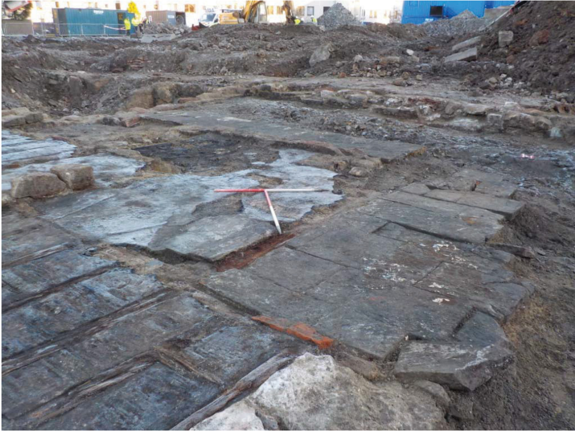
Plate 7: Upper Level, general view of Rooms 3 and 4
