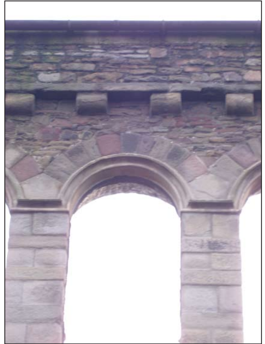
Plate 6: Detail of Upper Northern Elevation Looking South
