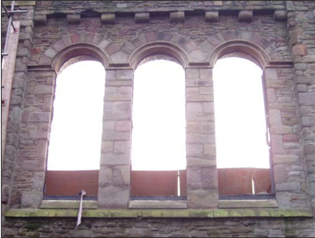
Plate 5: Detail of the Windows on Northern Elevation Looking South
