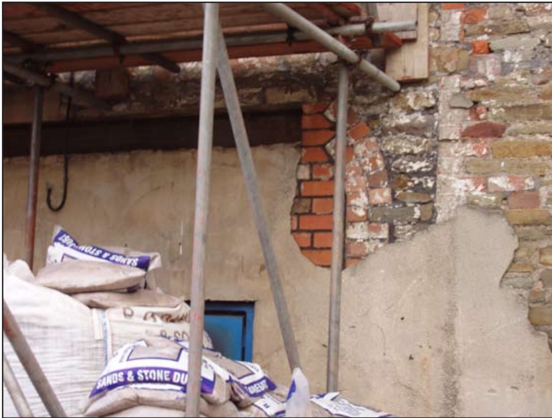
Plate 9: Detail of Phased Alterations in Eastern Elevation Looking West
