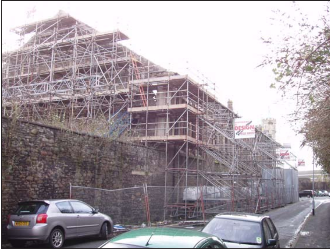
Plate 3: Northern Elevation Looking Southwest
