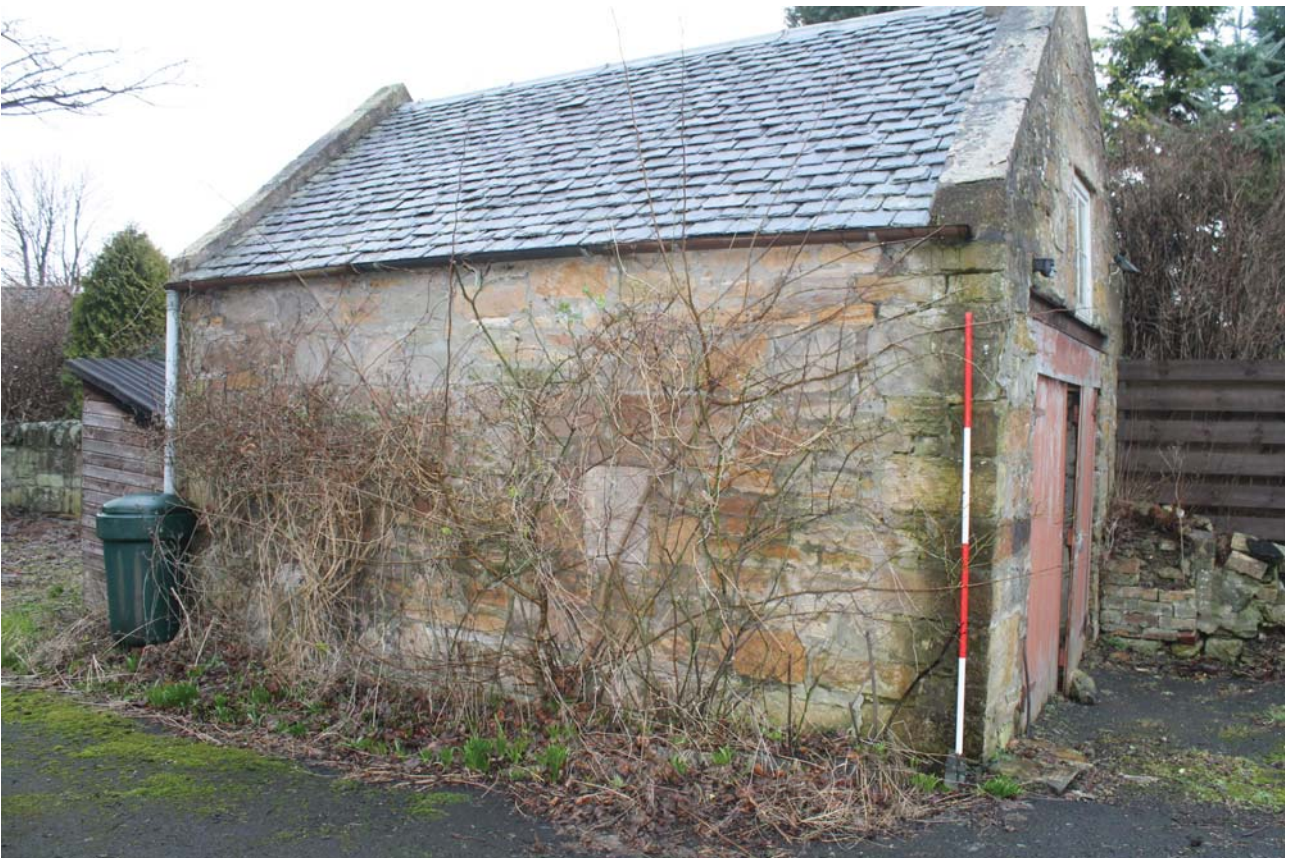
Plate 4: General view of the south-east elevation from the east
