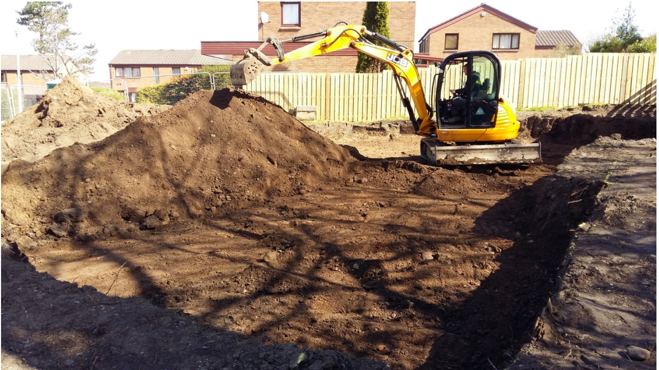
Plate 11: General view of the topsoil strip
