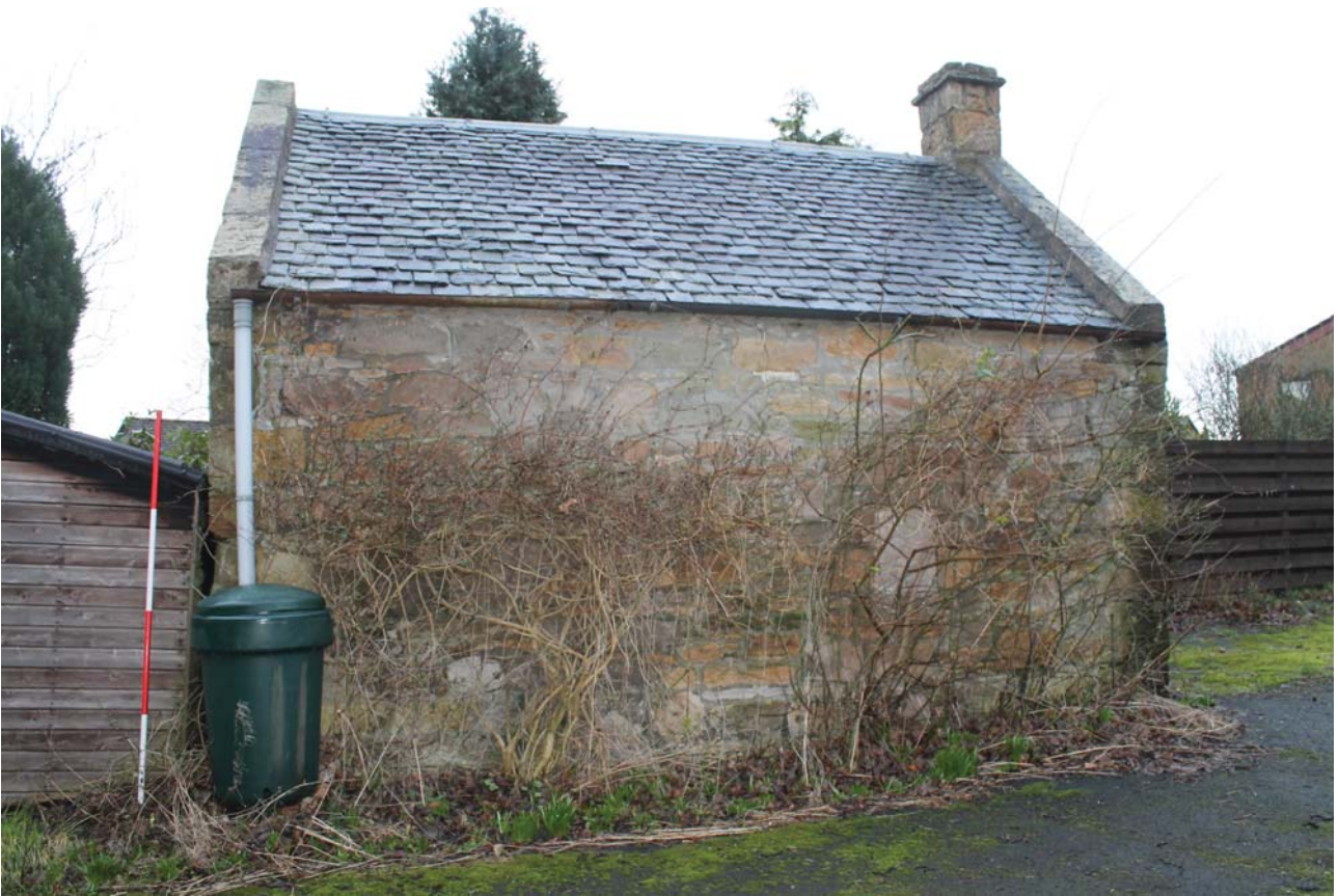
Plate 5: General view of the south-east elevation from the south-east
