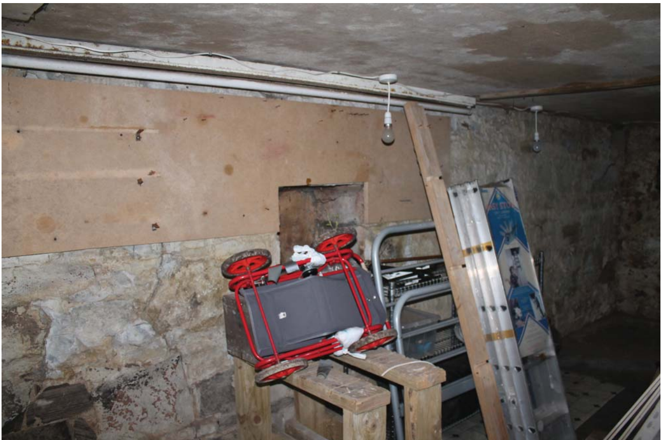
Plate 8: General view of the interior from the north
