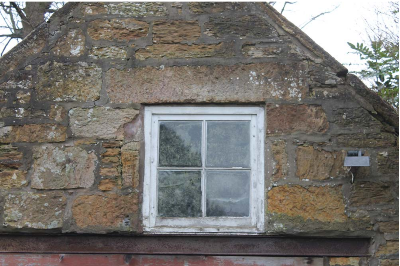
Plate 3: Detail of window on the north-east gable from the north-east
