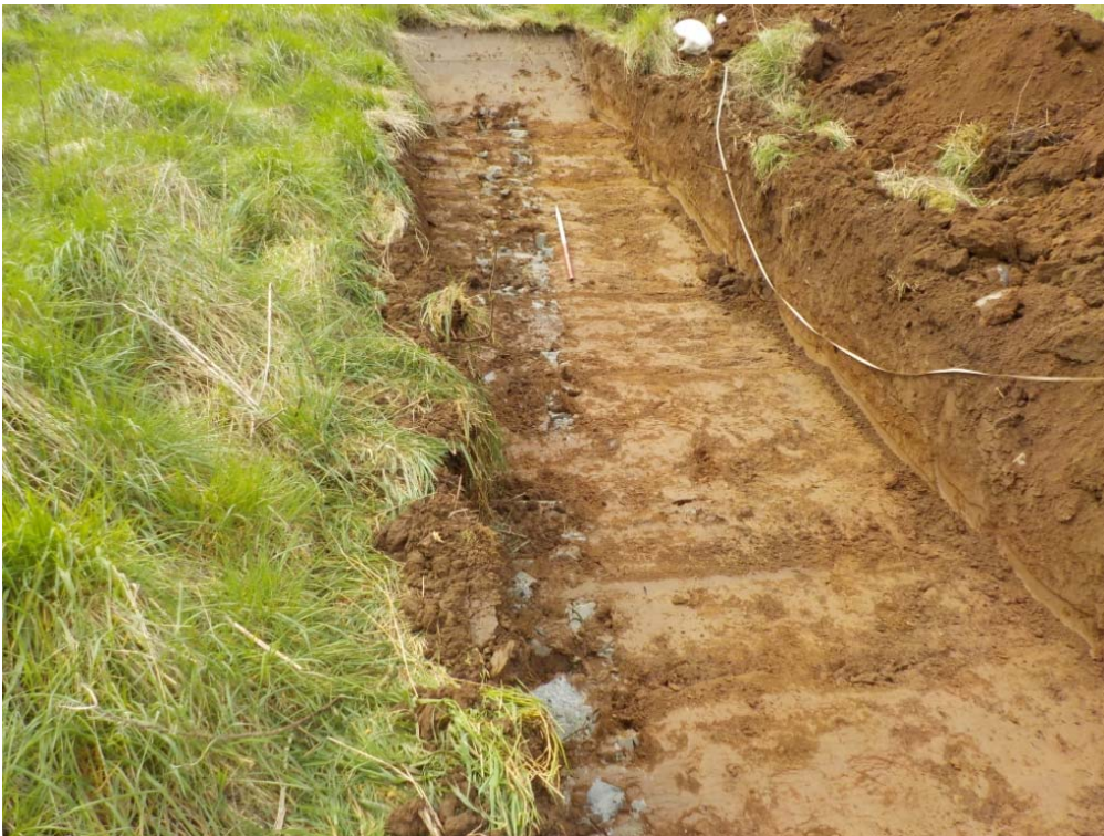
Plate 3 - General view of Culvert [2801]
