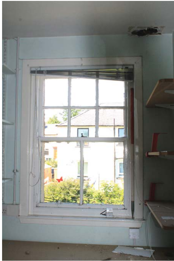
Plate 29: Room 1/8, detail of west wall window from the east
