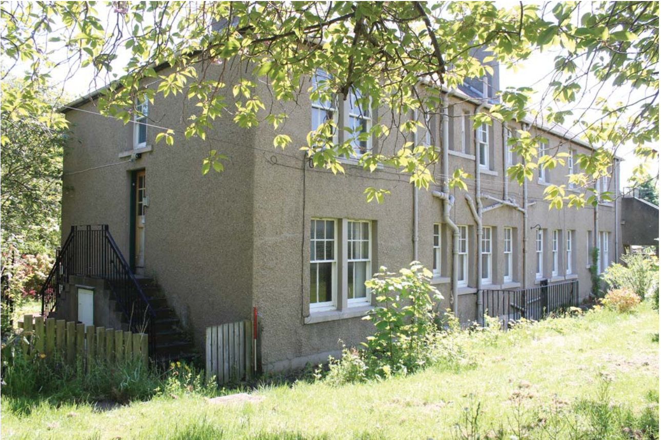
Plate 7: North & West elevations, general view from the north-east
