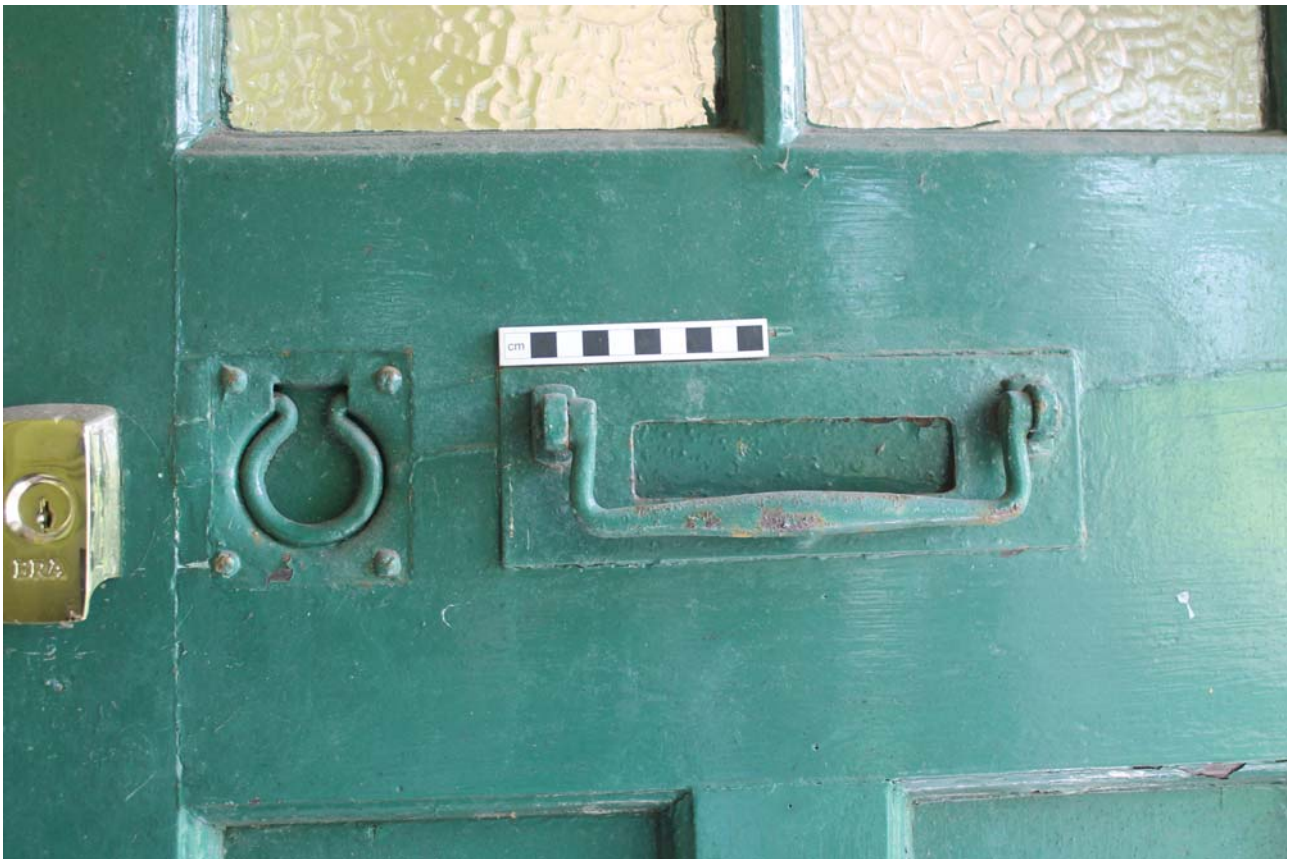
Plate 5: East elevation, detail of fittings to main entrance, from the south
