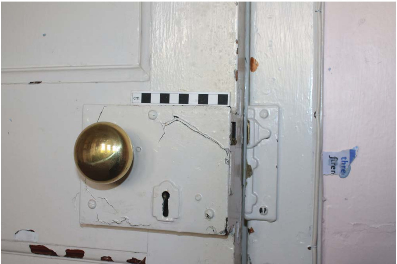
Plate 13: Room 0/5a, detail of original door fittings from the west
