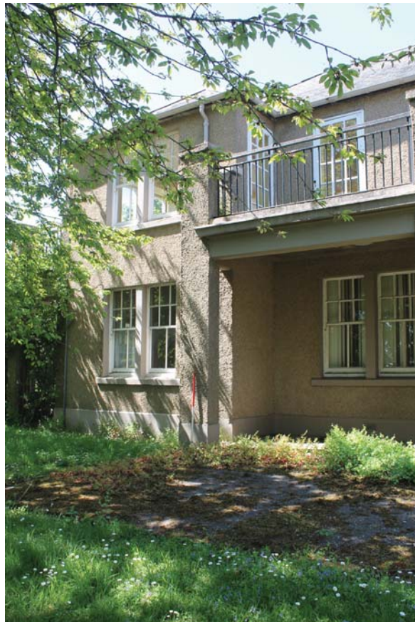
Plate 2: East elevation, general view of south side from the north-east
