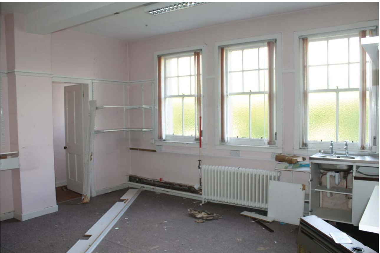
Plate 18: Room 0/5a, general view from the north-east
