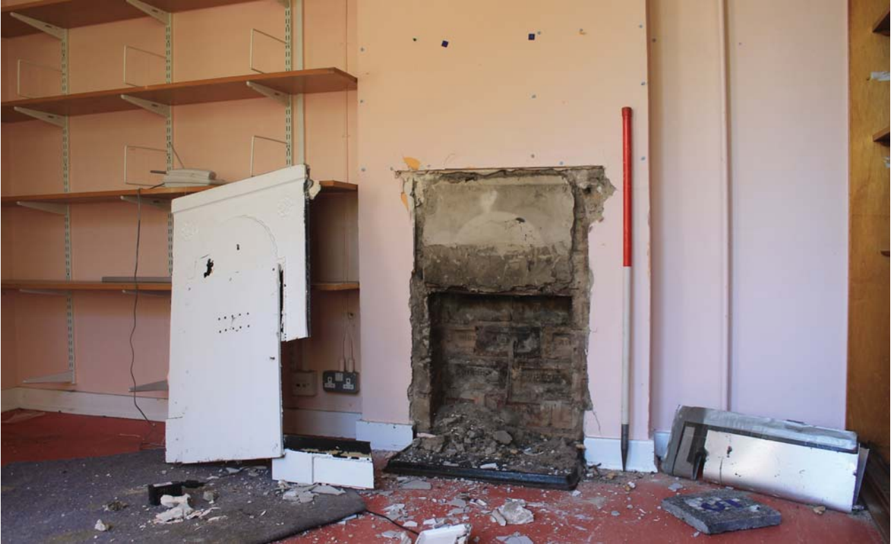
Plate 25: Room 1/3, detail of fireplace and removed surround from the east
