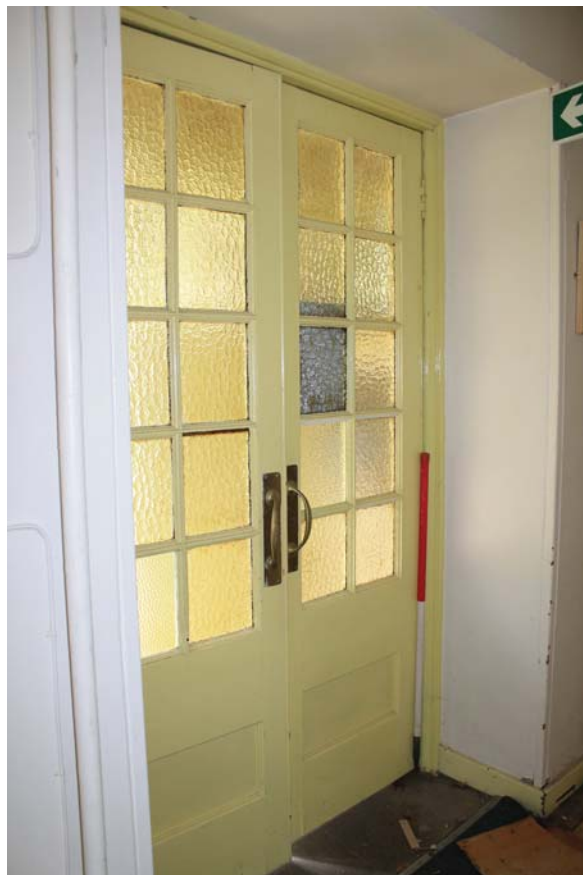
Plate 12: Room 0/1, detail from the main entrance from the north-east
