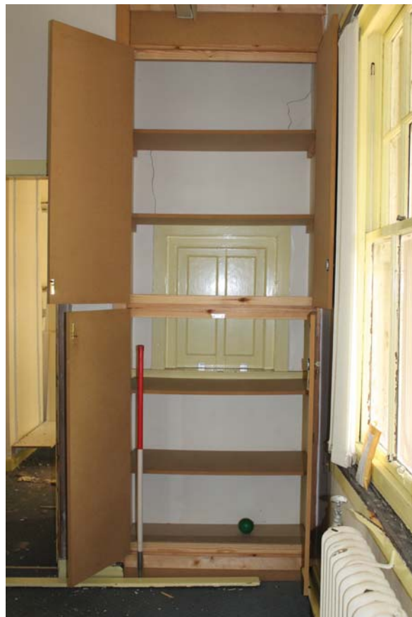
Plate 14: Room 0/1, detail of hatch in the north wall from the south
