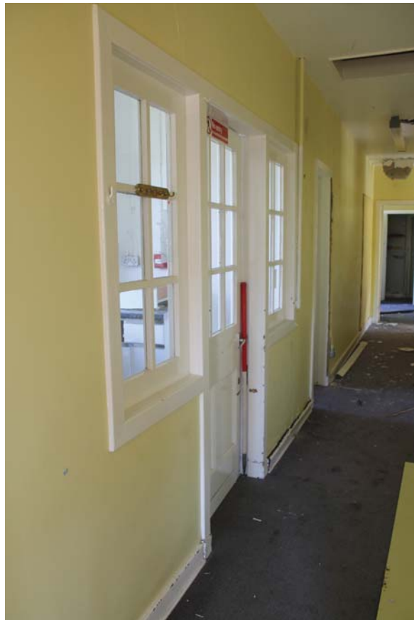
Plate 28: Room 1/2, detail of door to Room 1/7 from the south-east
