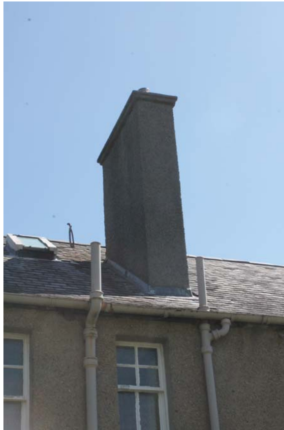
Plate 9: West elevation, detail of chimney from the NNE
