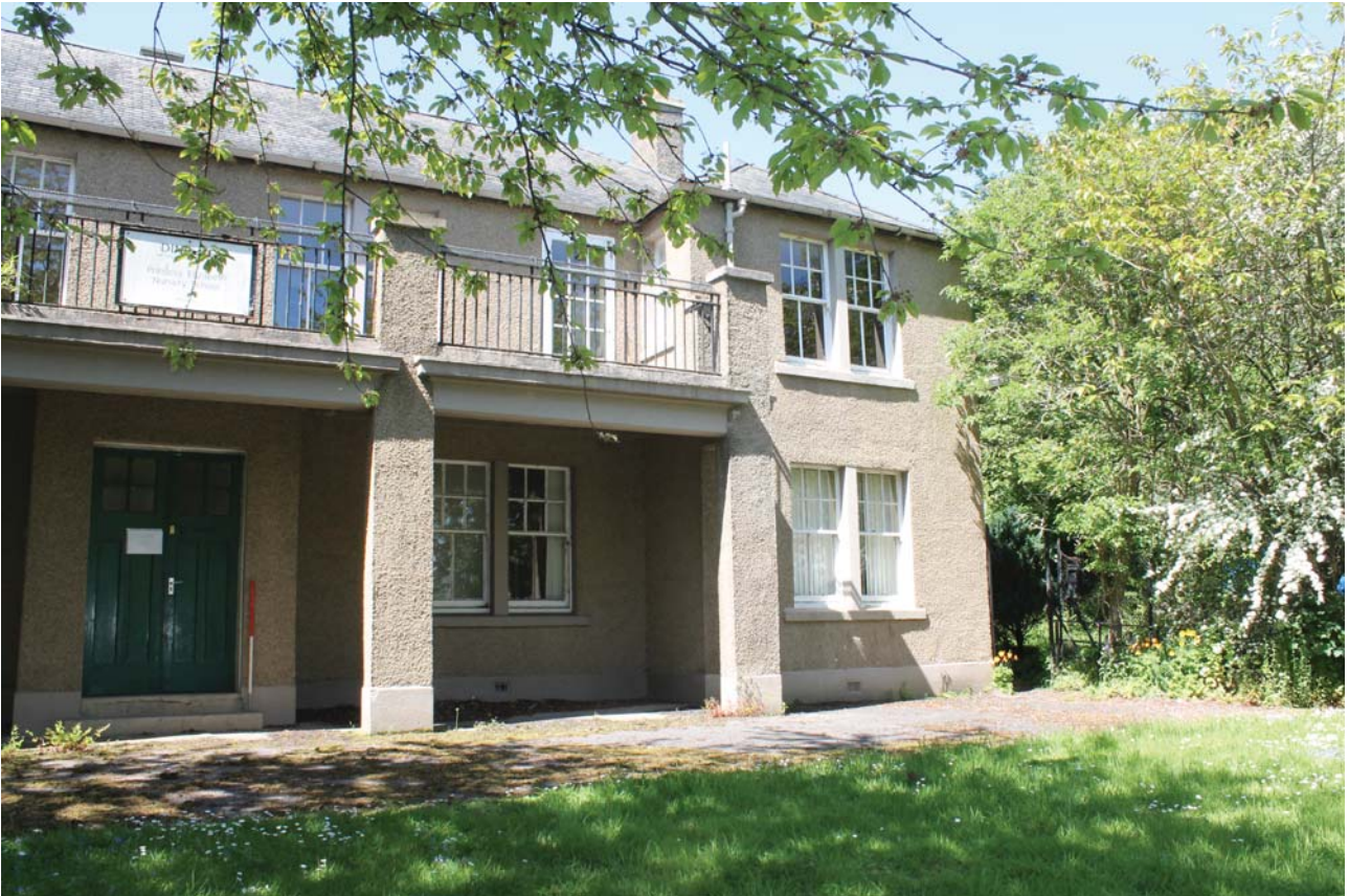
Plate 3: East elevation, general view of the north-side from the south-east
