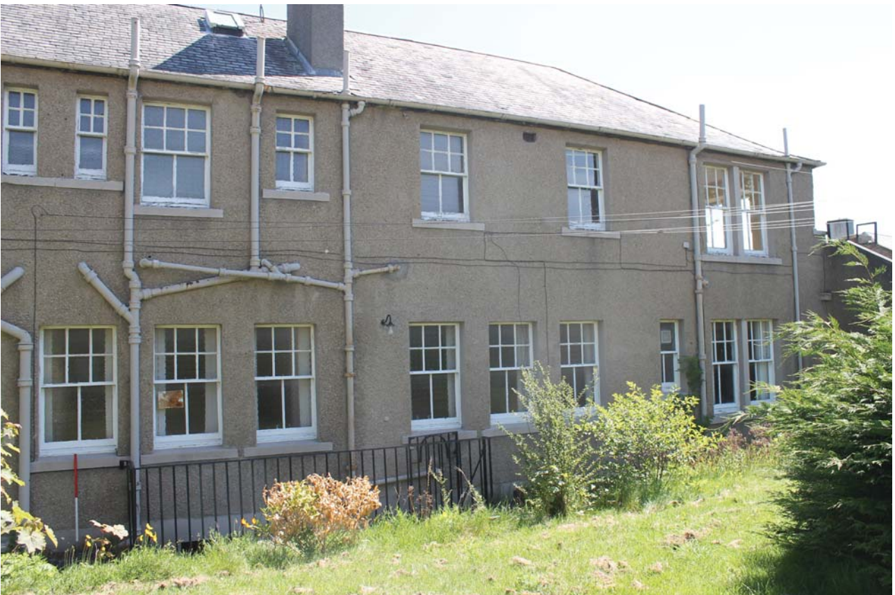
Plate 8: West elevation, general view of south side from the north-east
