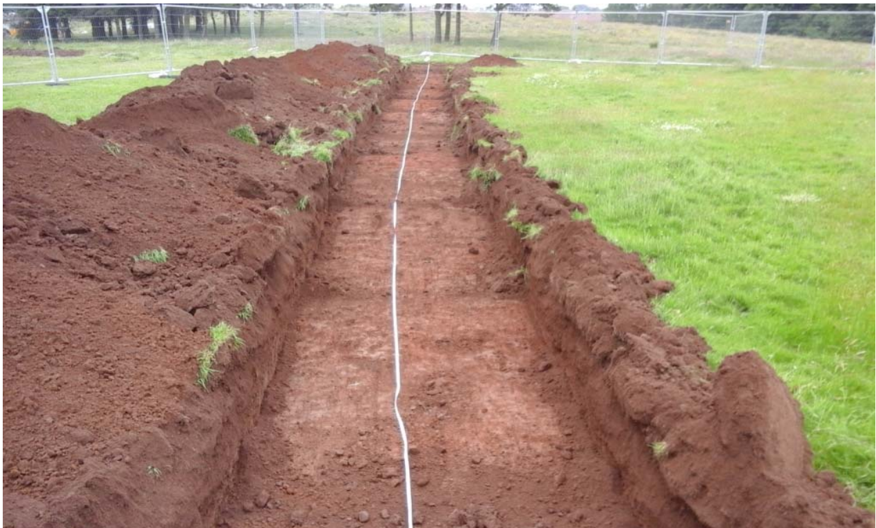
Plate 1 - General view of Trench 6
