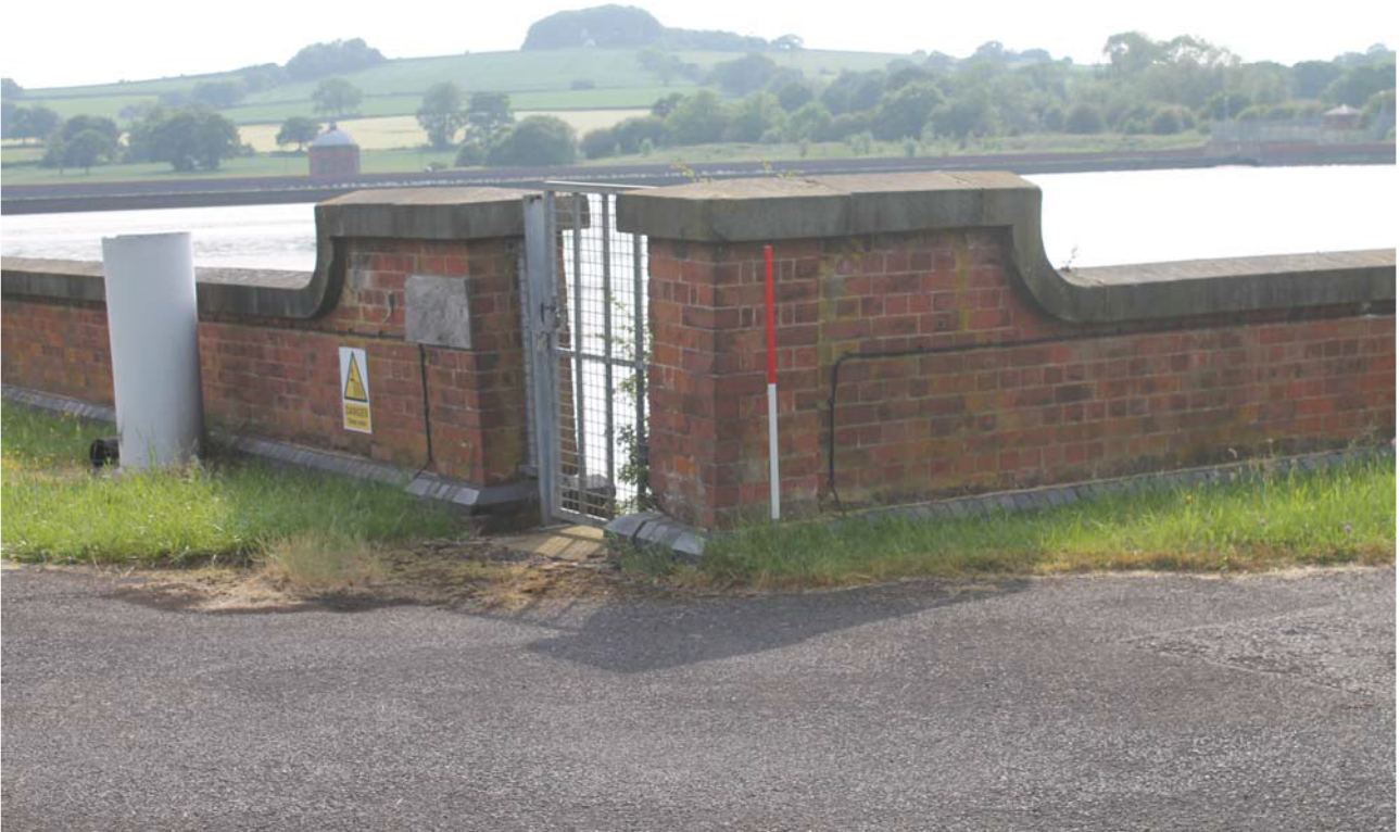
Plate 15: Reservoir, detail of entrance to the north-east corner from the east
