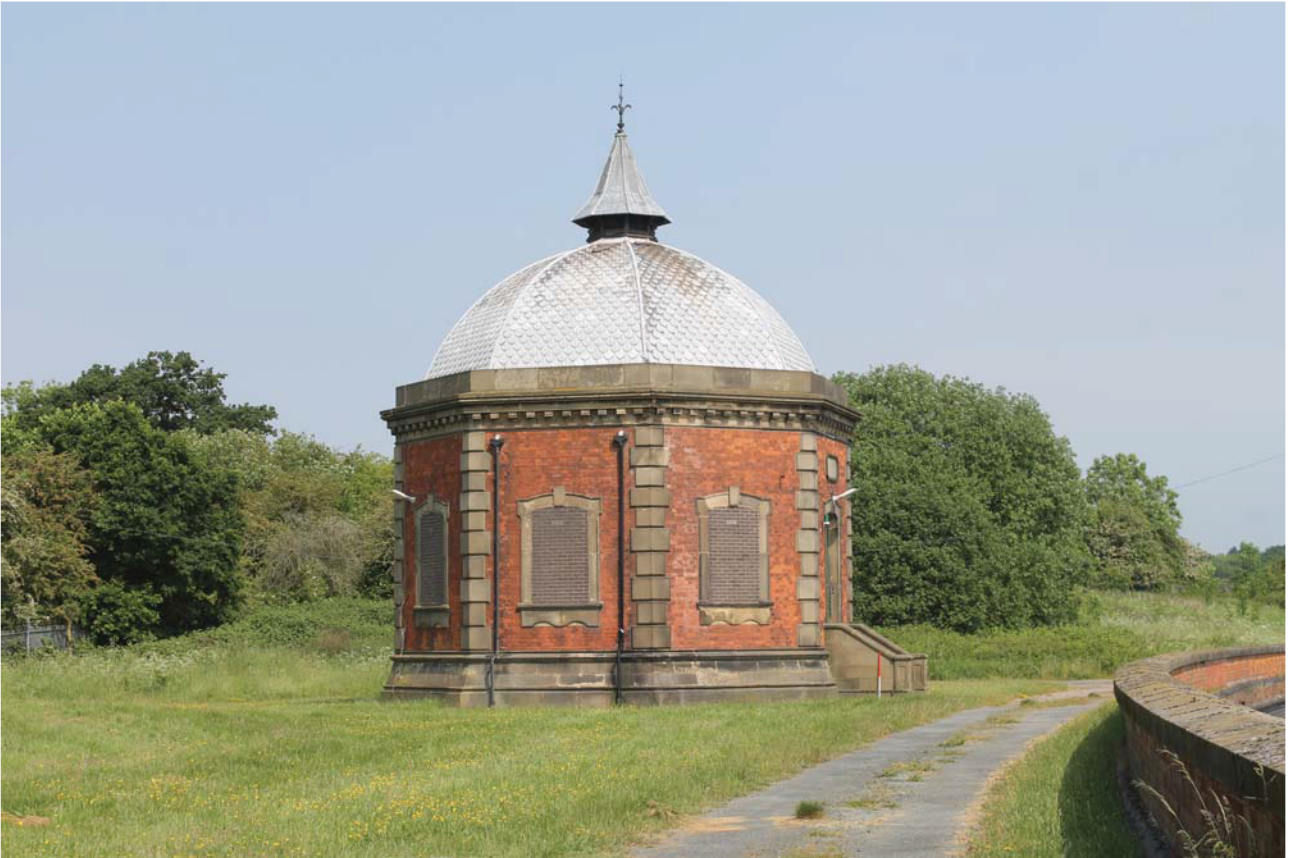
Plate 19: Outlet House 1, general view from the south
