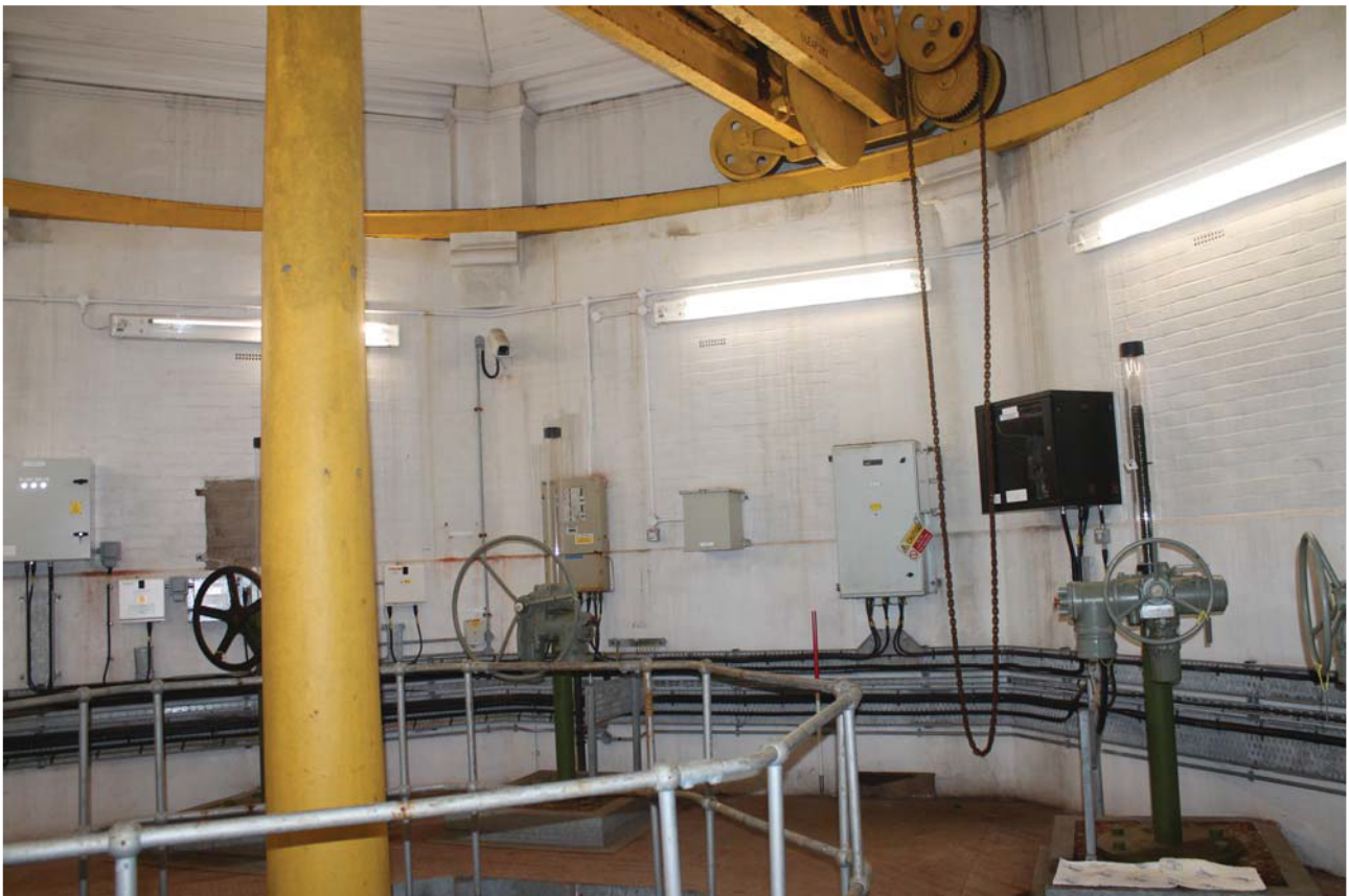
Plate 30: Outlet House 1 Interior, general view from the south-east
