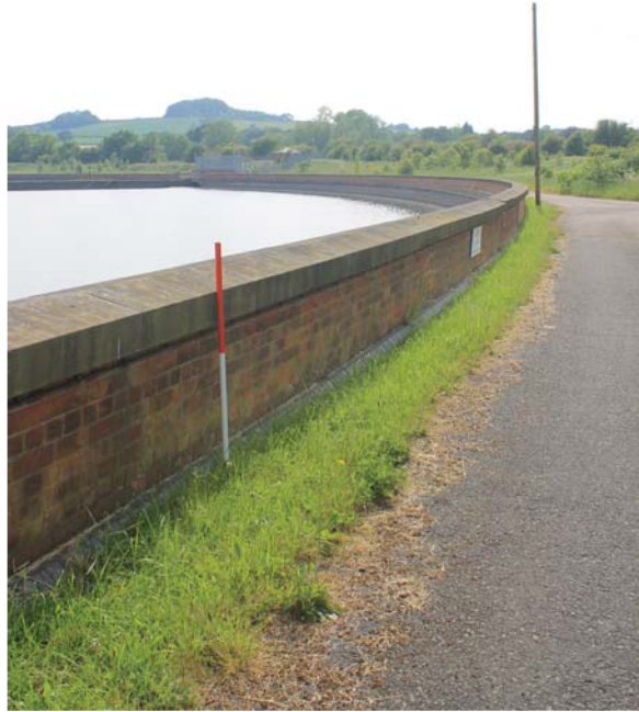
Plate 5: Reservoir, general view from the north-east
