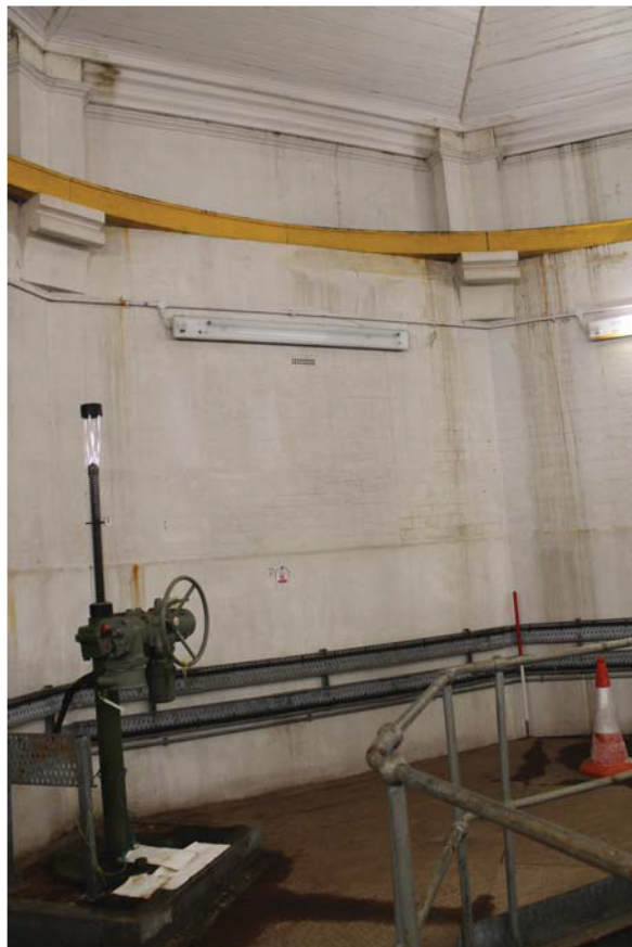
Plate 28: Outlet House 1 Interior, general view from the east
