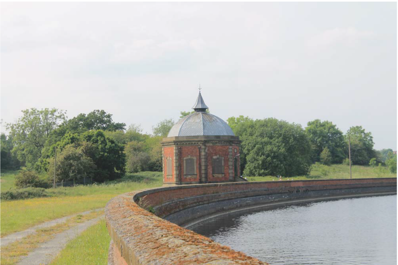
Plate 18: Outlet House 1, general view from the south
