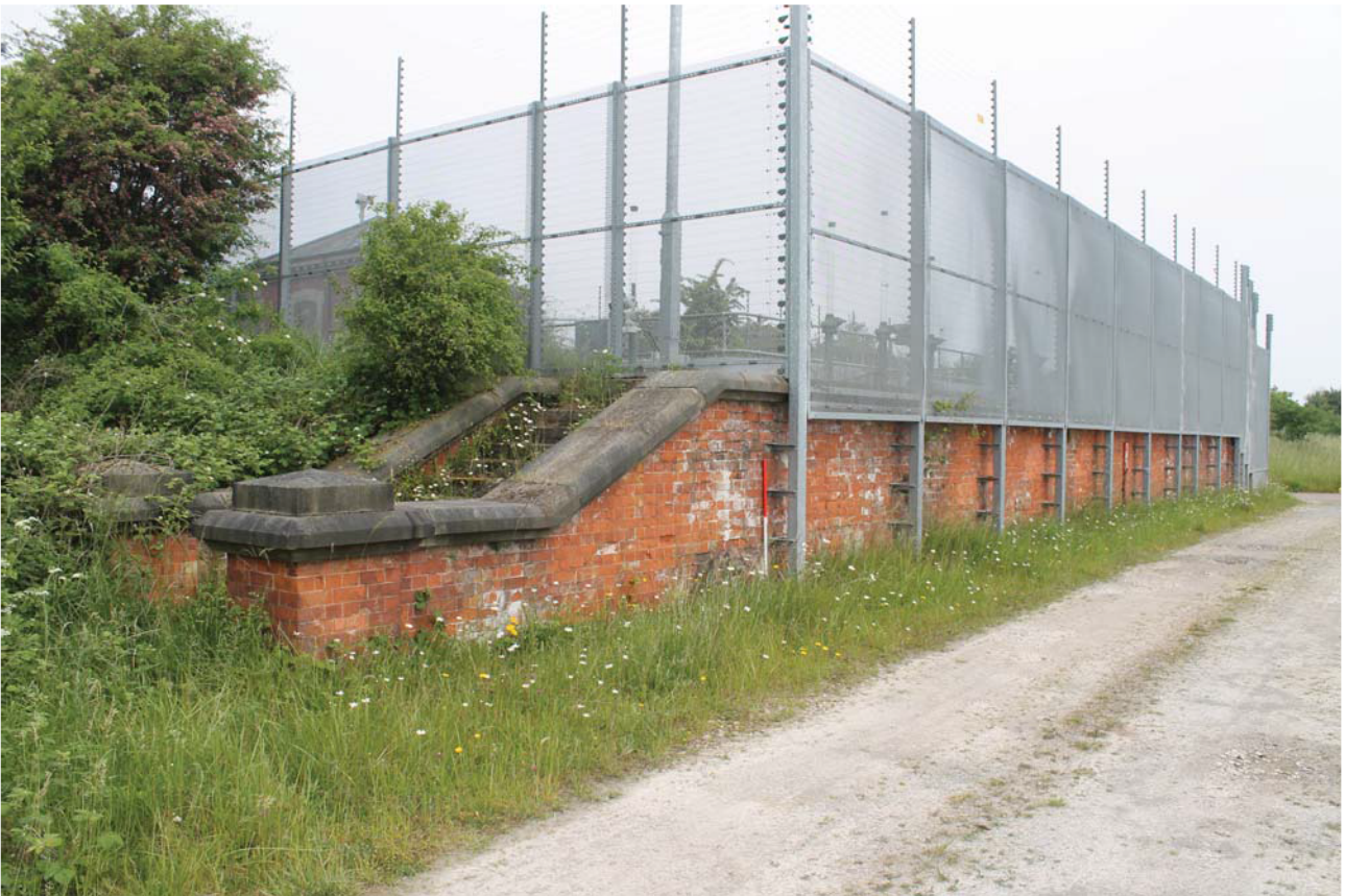
Plate 59: Inlet House, general view of south-east boundary wall from the south
