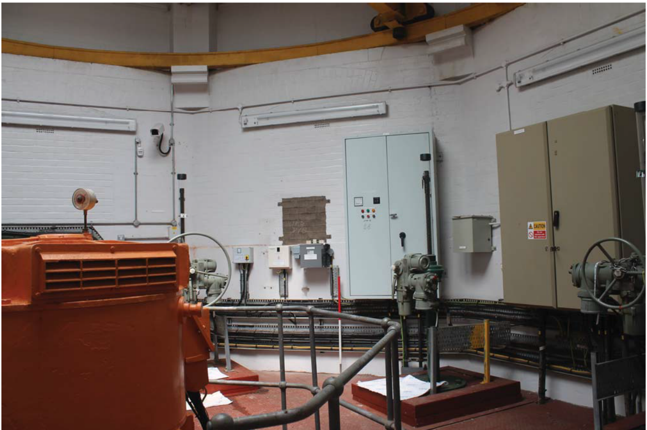
Plate 42: Outlet House 2 Interior, general view from the south
