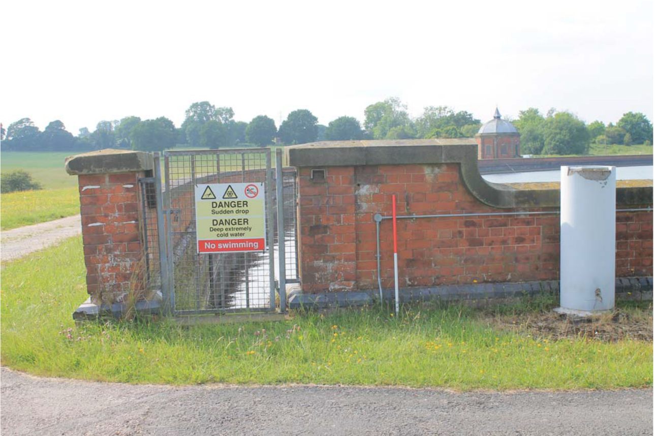
Plate 17: Reservoir, detail of entrance to the south-west corner from the north-west
