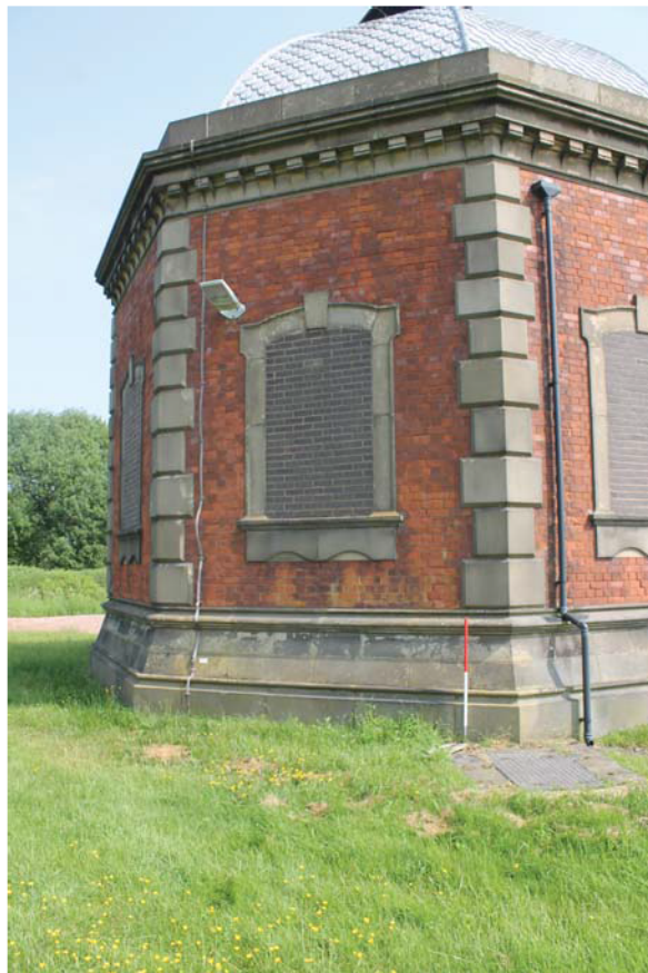
Plate 26: Outlet House 1, detail of window bay from the south-west
