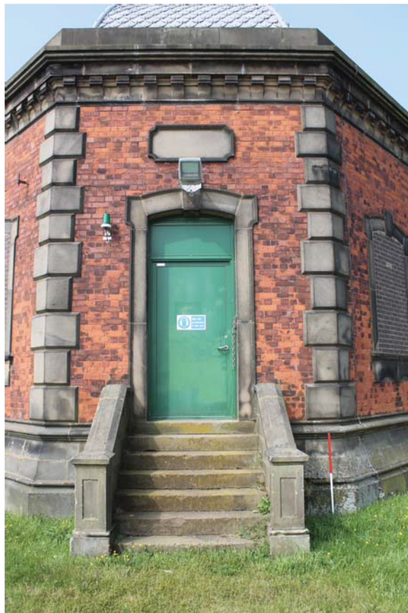
Plate 22: Outlet House 1, detail of main entrance from the south-east
