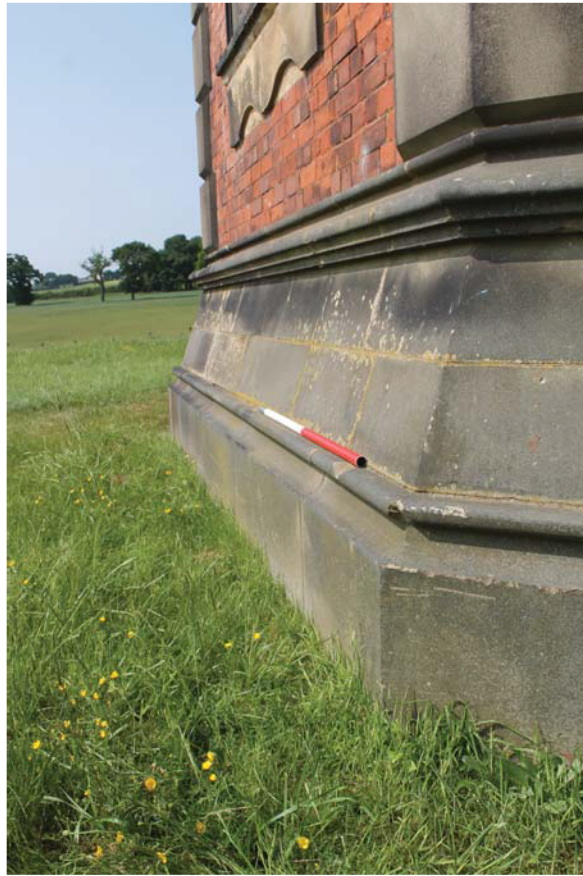
Plate 21: Outlet House 1, detail of footing from the south-east
