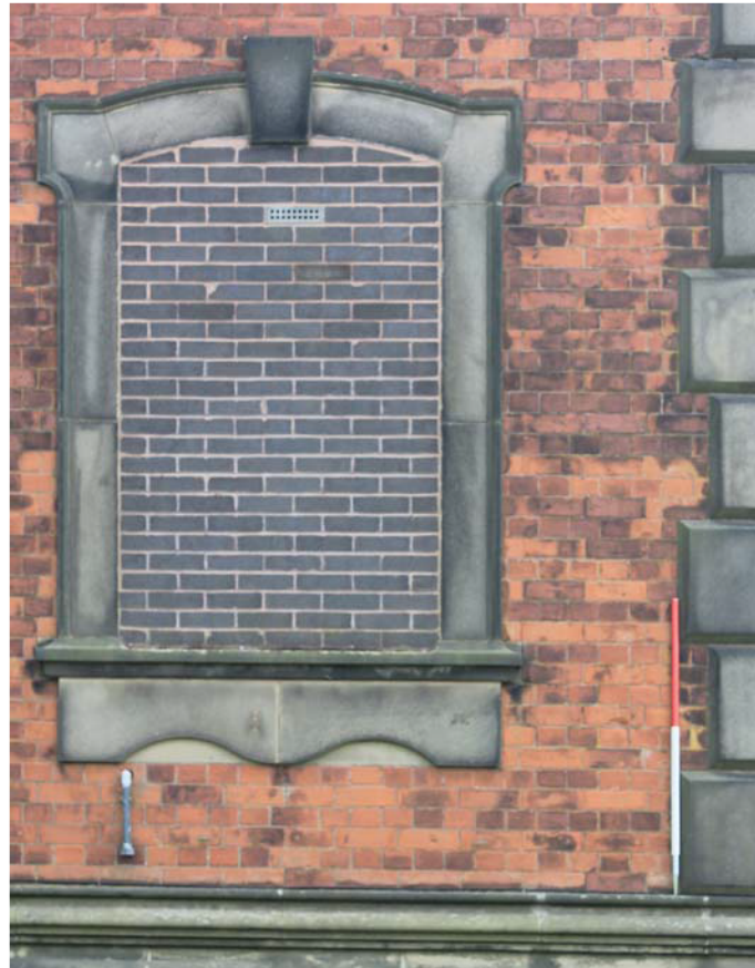
Plate 39: Outlet House 2, detail of window bay from the west
