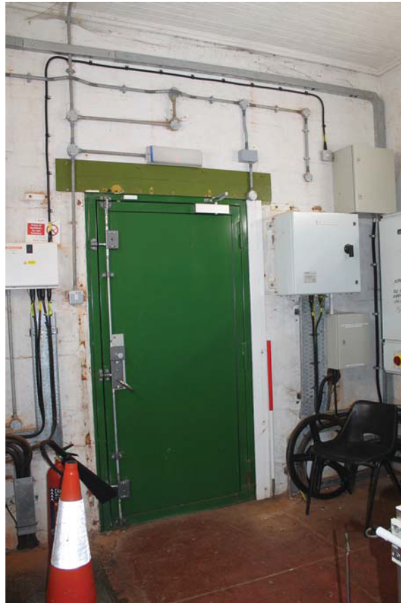
Plate 41: Outlet House 2 Interior, detail of the main entrance from the north
