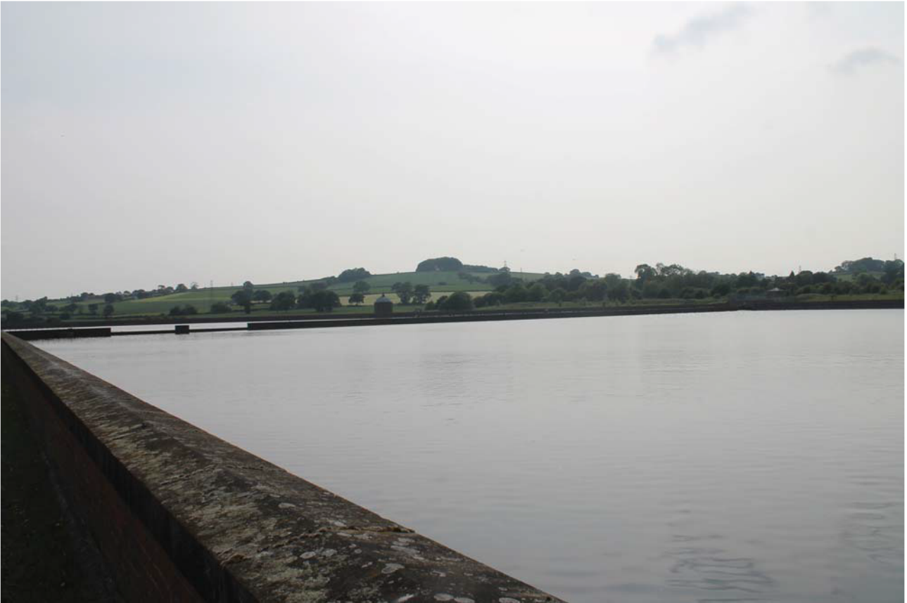
Plate 1: Reservoir, general view from the east
