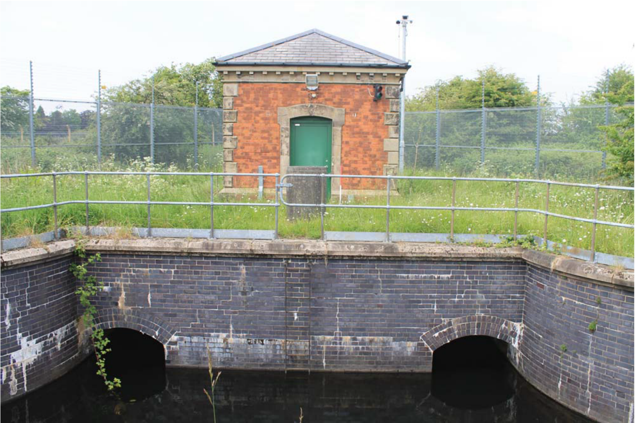
Plate 47: Inlet House, general view from the south-east
