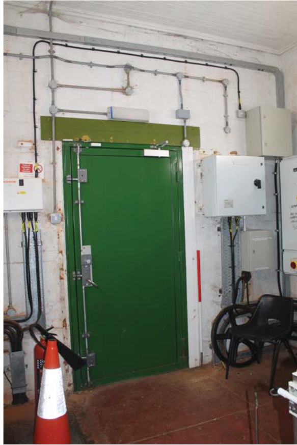
Plate 53: Inlet House Interior, detail of main entrance from the north
