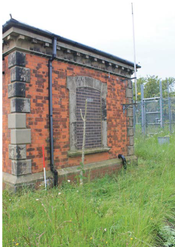
Plate 50: Inlet House, detail of north-east elevation from the east
