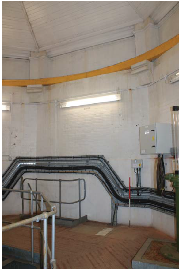
Plate 29: Outlet House 1 Interior, general view from the south
