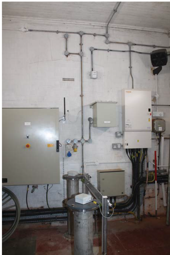
Plate 54: Inlet House Interior, general view from the south-east
