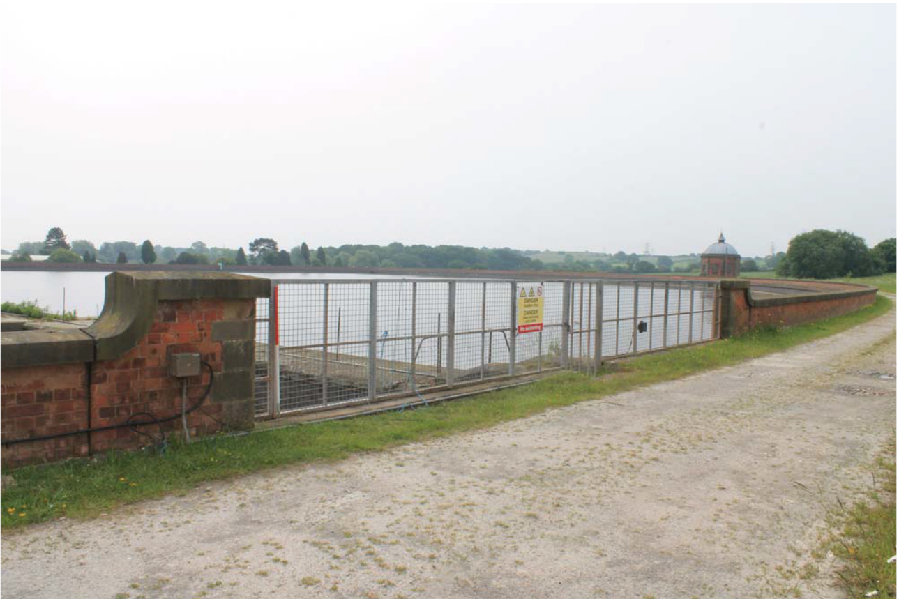
Plate 13: Reservoir, detail of entrance in the north-west wall from the north-west
