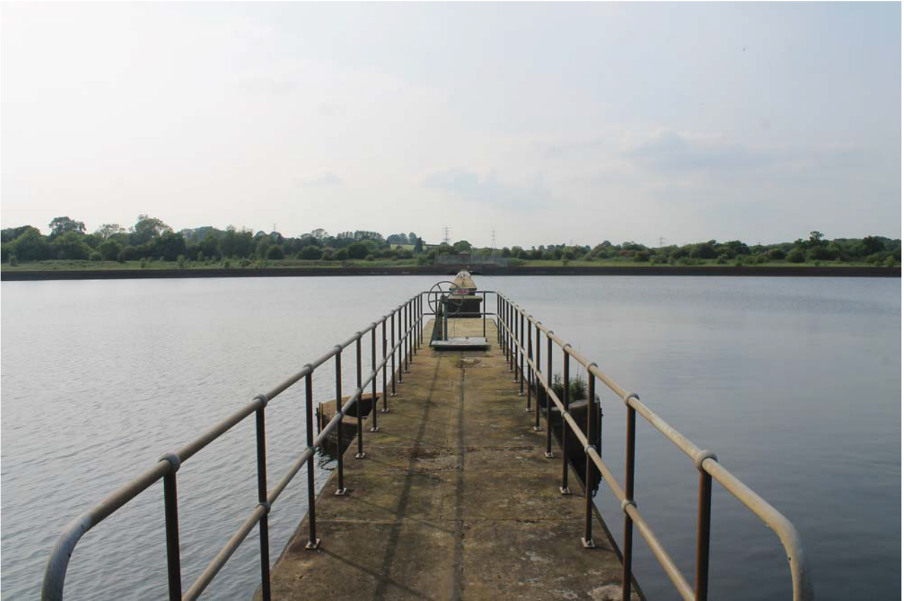
Plate 9: Reservoir, detail of central dividing wall from the north-west
