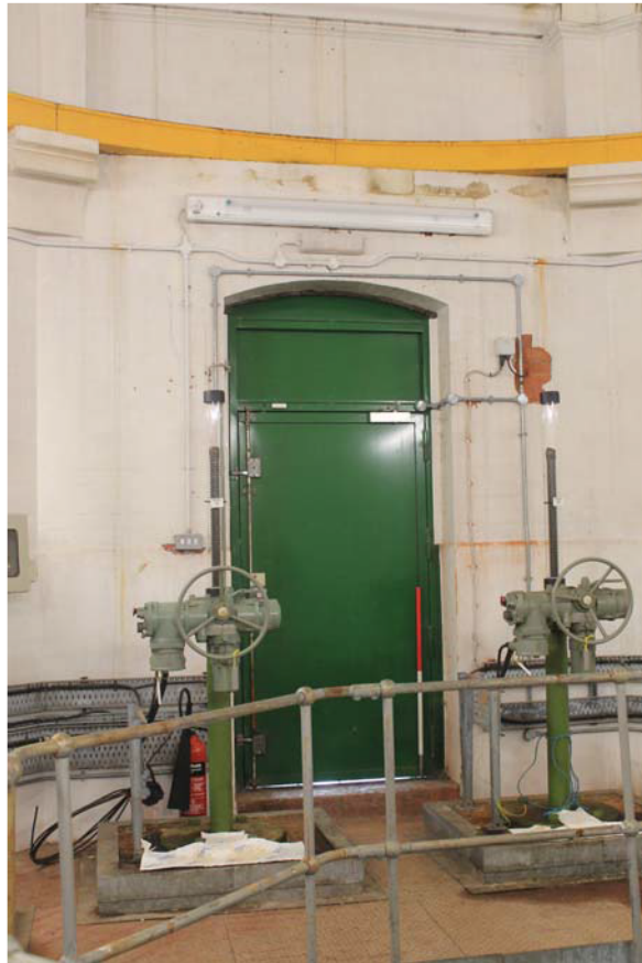
Plate 27: Outlet House 1 Interior, detail of main entrance from the north
