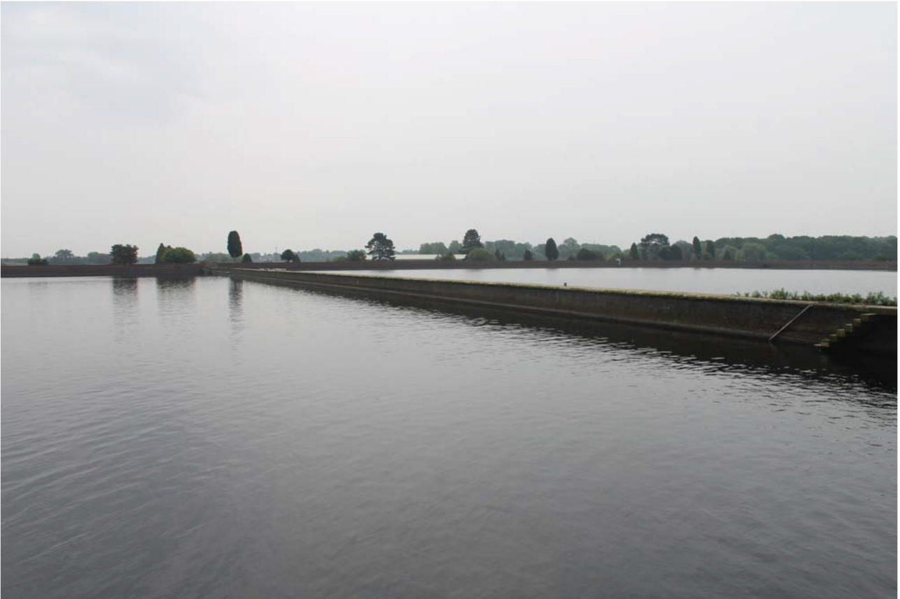
Plate 11: Reservoir, general view of the central dividing wall from the north
