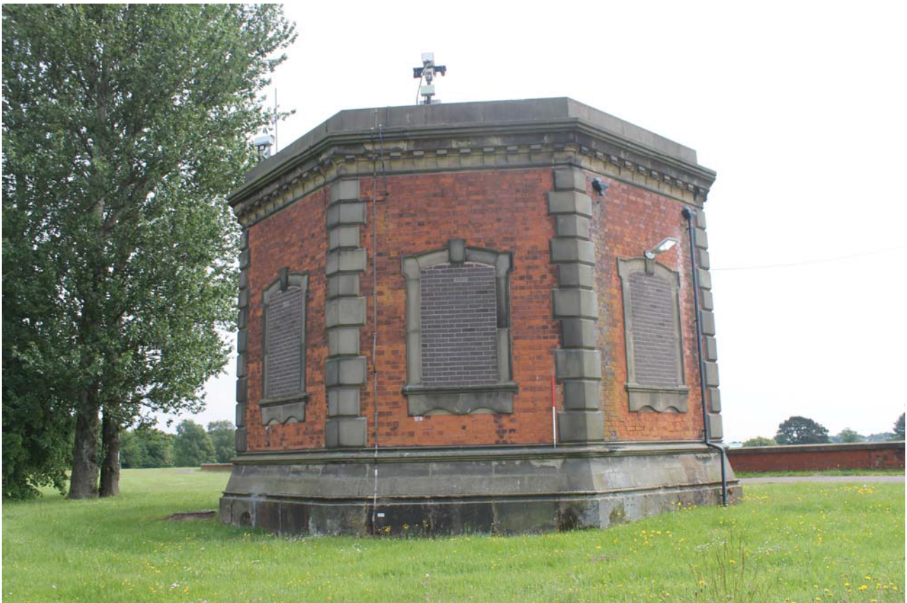
Plate 40: Outlet House 2, detail of window bay from the west
