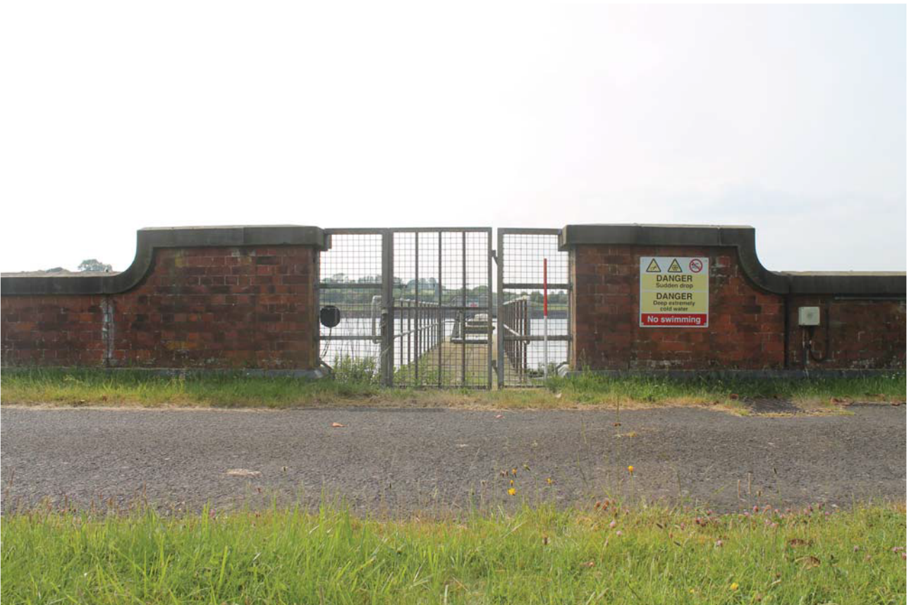
Plate 14: Reservoir, detail of entrance to the south corner from the south-east
