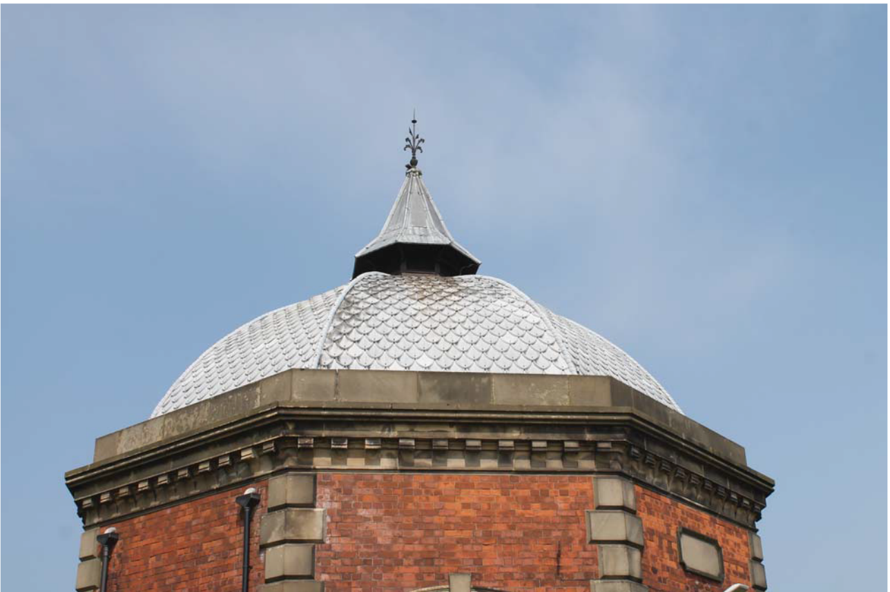
Plate 20: Outlet House 1, detail of roof from the south
