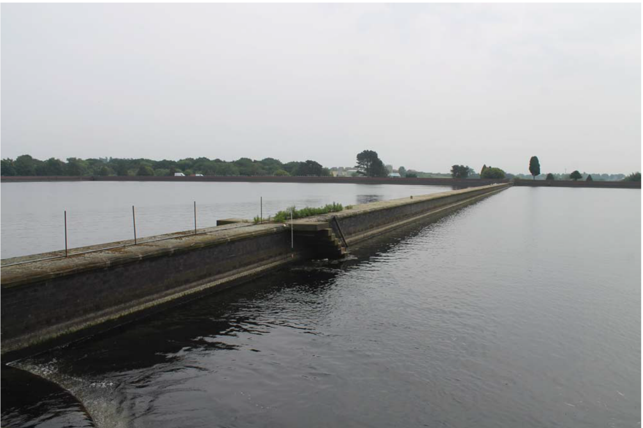
Plate 10: Reservoir, general view of the central dividing wall from the west
