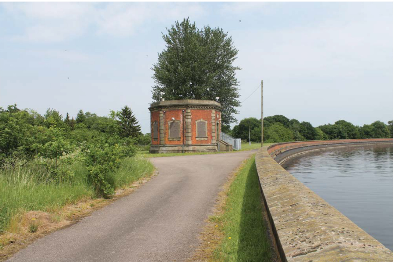
Plate 34: Outlet House 2, general view from the south-west
