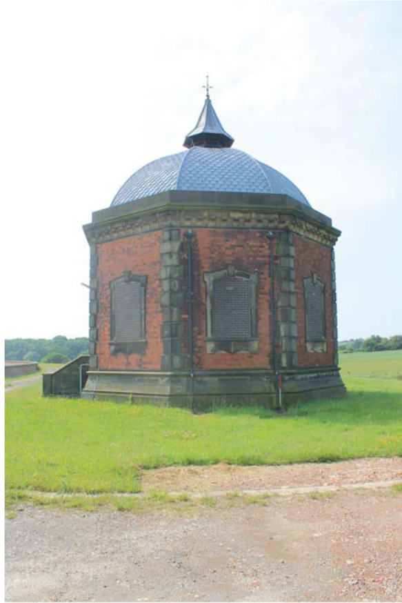
Plate 25: Outlet House 1, detail of window bay from the north-east
