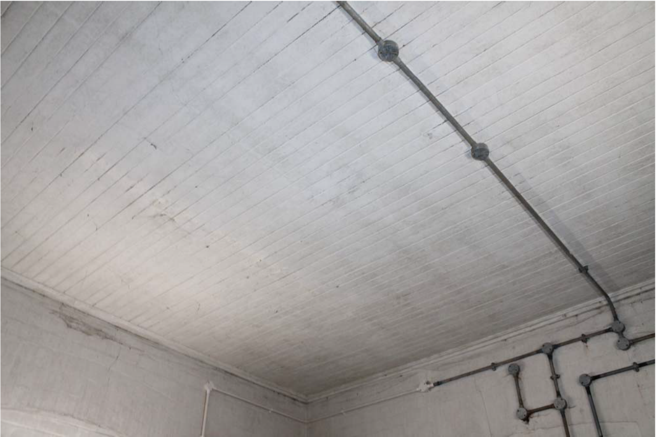
Plate 55: Inlet House Interior, detail of ceiling from the east
