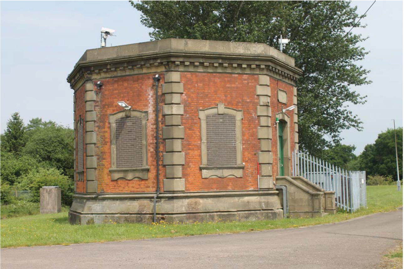
Plate 35: Outlet House 2, general view from the south-west
