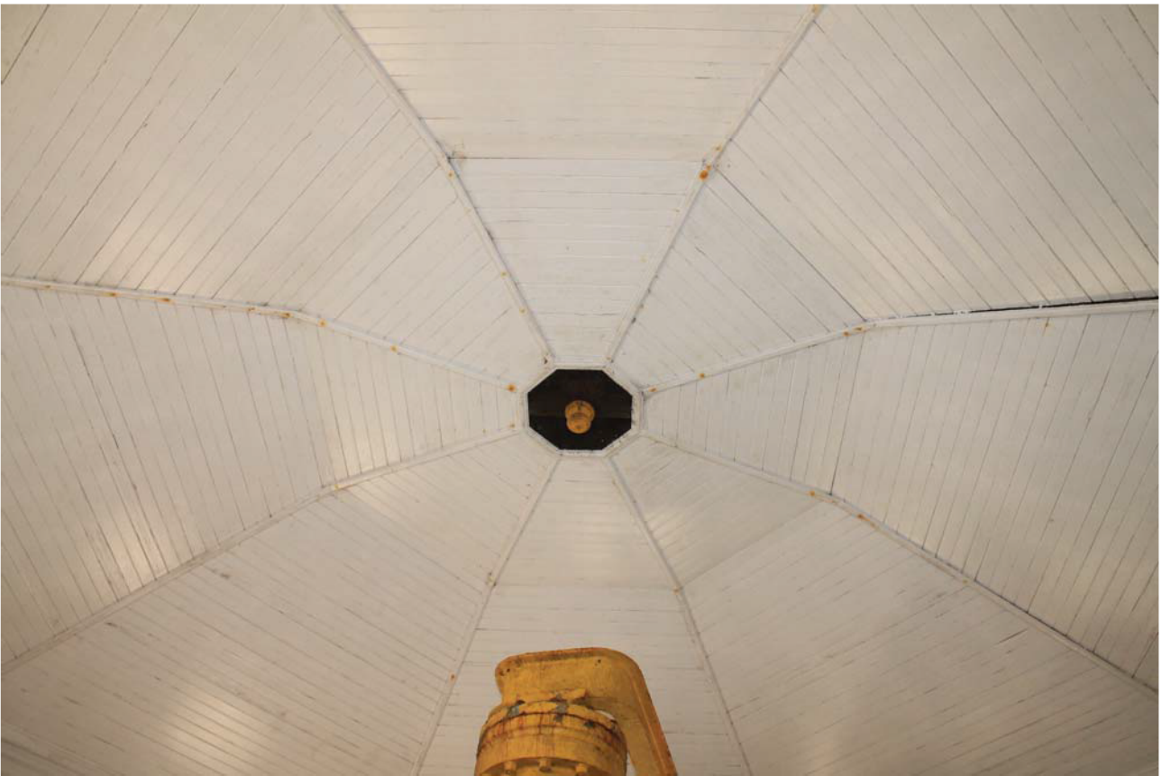
Plate 33: Outlet House 1 Interior, detail of the roof from the south-east
