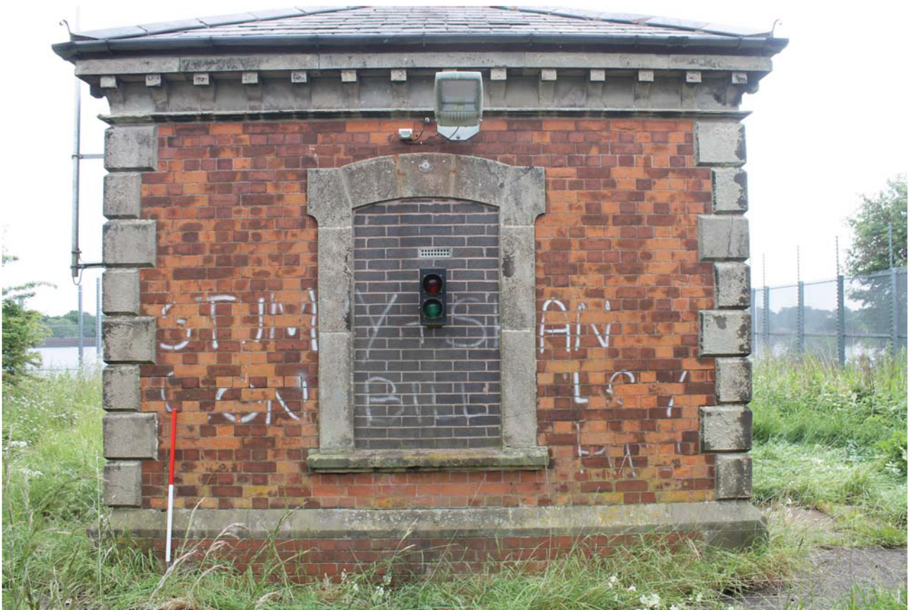
Plate 51: Inlet House, detail of the north-west elevation from the north-west
