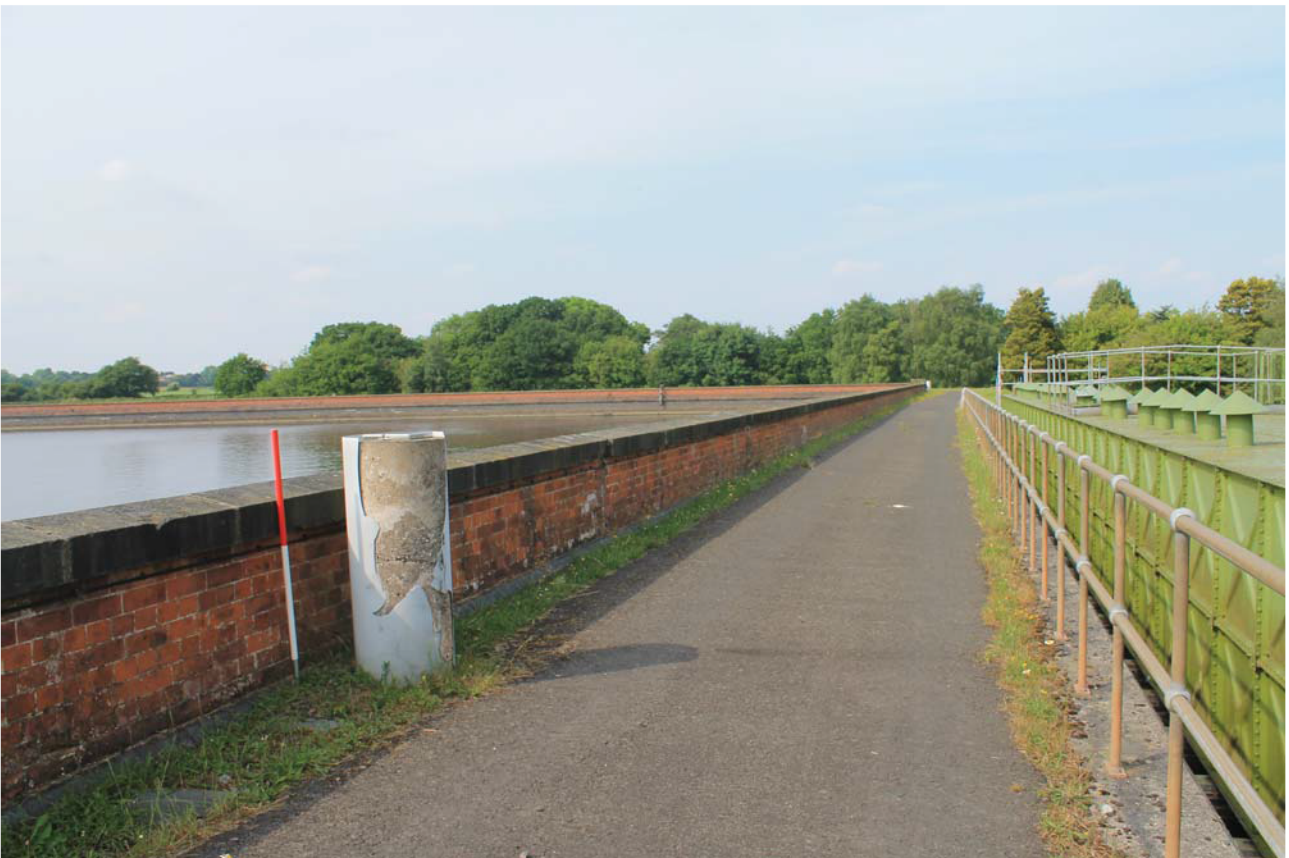
Plate 2: Reservoir, general view from the SSW
