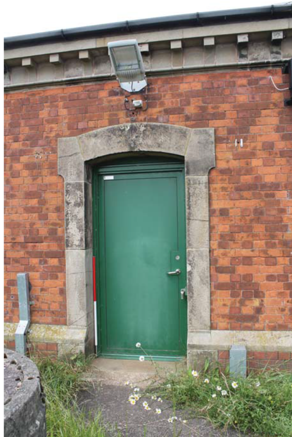
Plate 49: Inlet House, detail of the main entrance from the SEE
