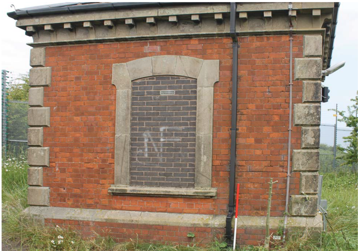
Plate 52: Inlet House, detail of the south-west elevation from the SSW
