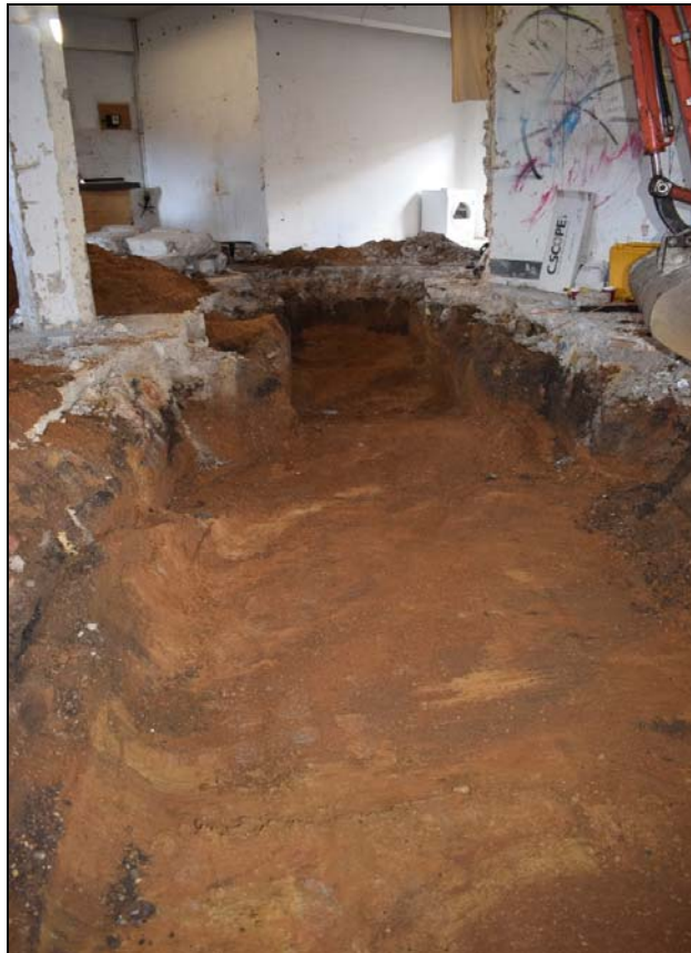
Plate 2, Trench, Looking North
