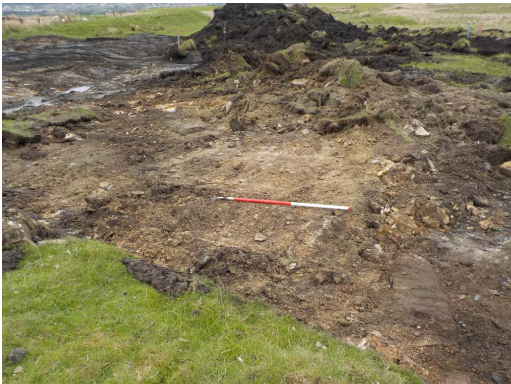
Plate 1: Post-ex Building foundations [102]
