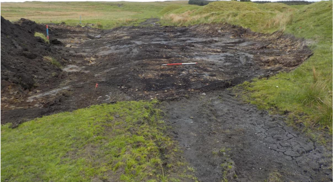
Plate 2: Post excavation view of Turbine 12 area, showing trackway [103]
