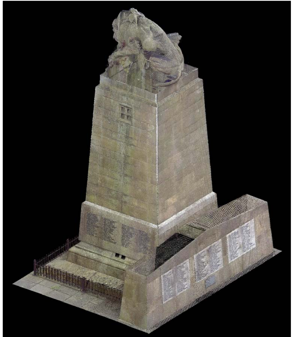
Figure 14: War memorial perspective north-east and south-west views, ortho-images of the laser scan data
