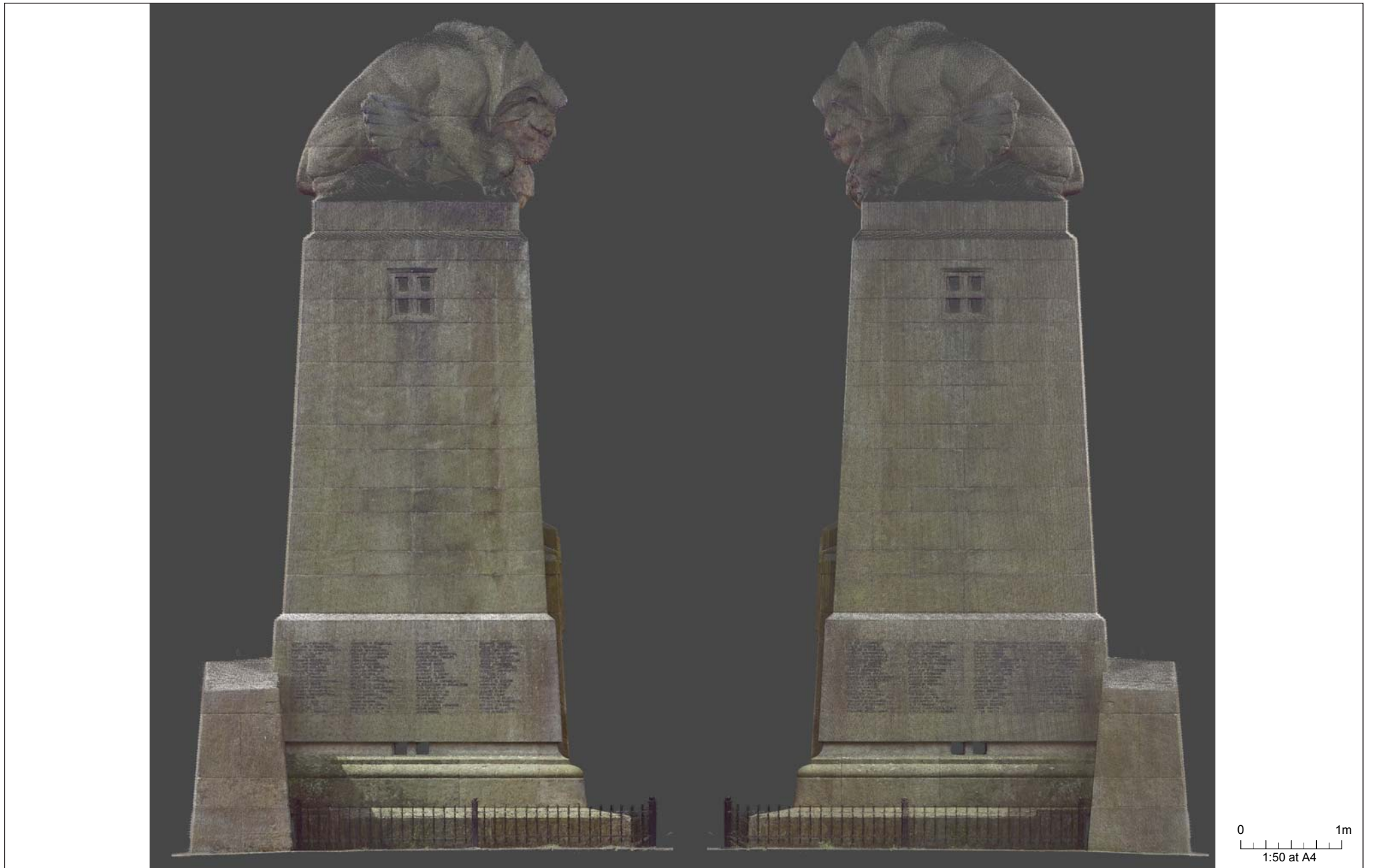
Figure 12: War memorial east and west elevation ortho-images of the laser scan data
