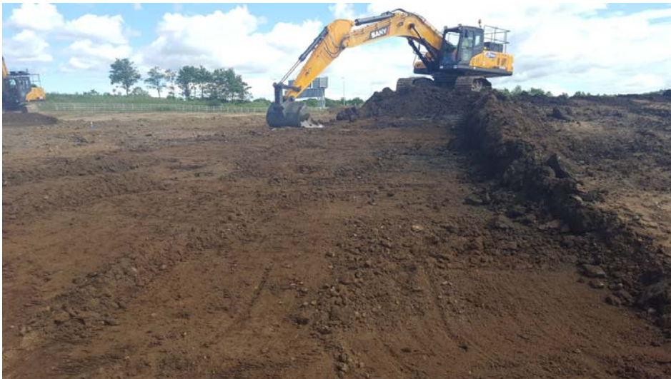
Plate 1: Topsoil stripping Plots 7 and 8
