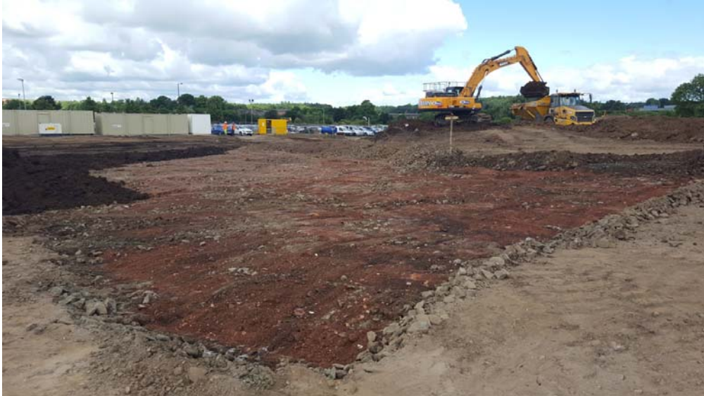
Plate 2: Made ground across the south of Plots 7 and 8
