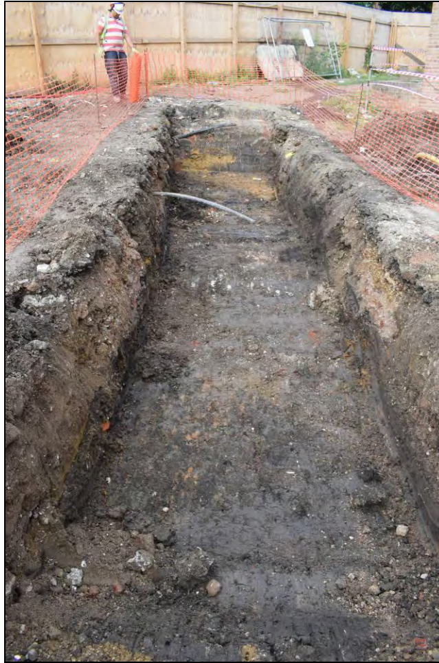
Plate 11: Trench 3 looking north-east prior to excavation of a sondage showing (304)
