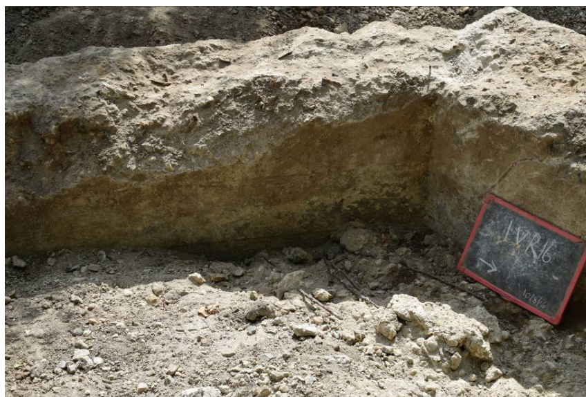
Plate B: Rebar visible in base, looking southwest
