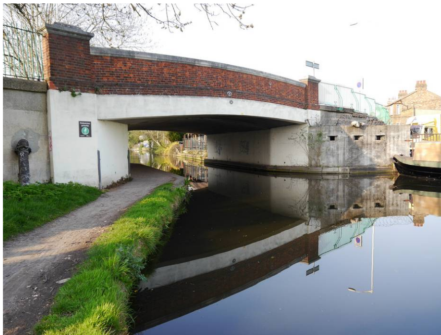
Plate G: Pillbox on Dolphin Bridge (Cousins, 2015)
