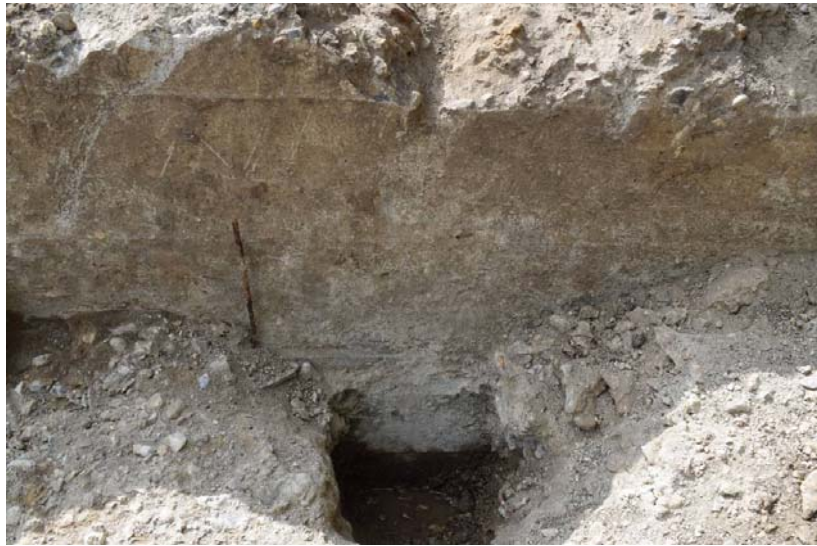
Plate C: Wooden shuttering marks, looking west
