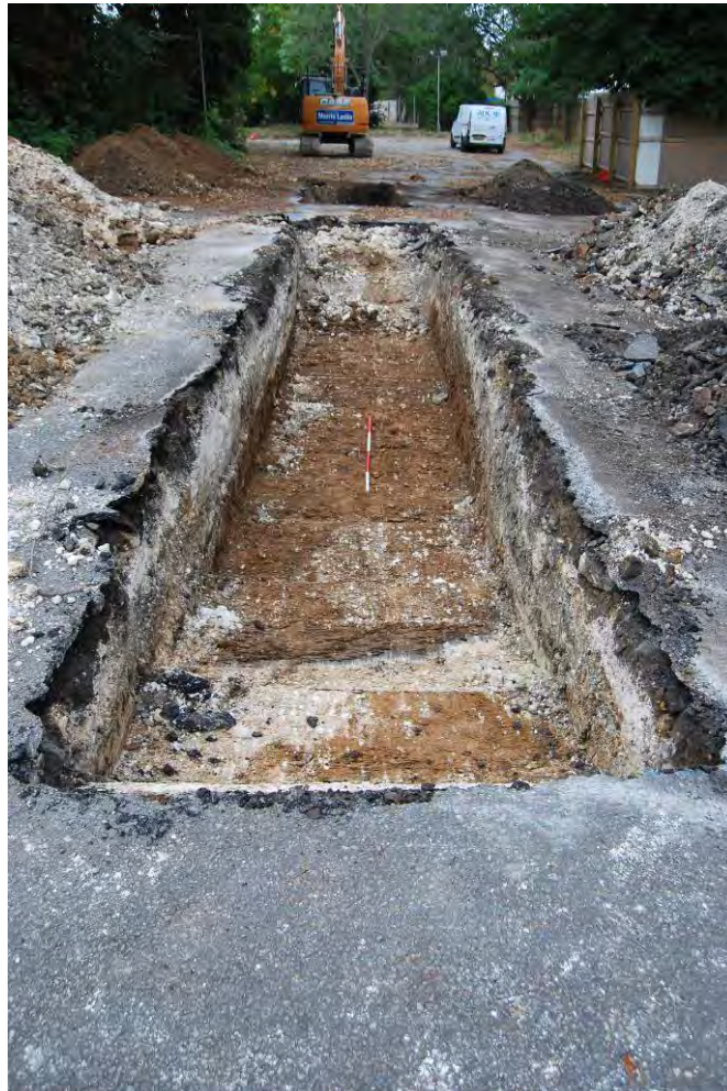
Plate 1: Trench 1 (looking north-west)
