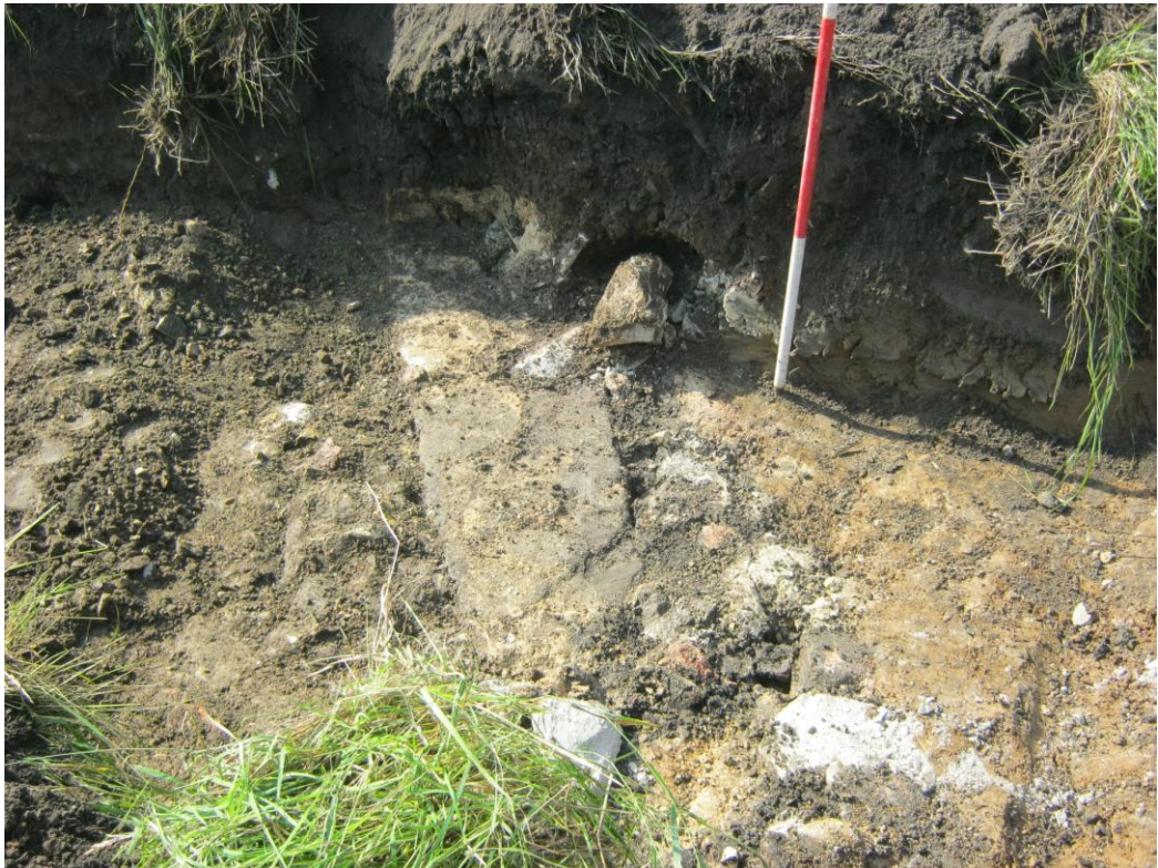
Plate 1: Boundary wall foundation [1601]
