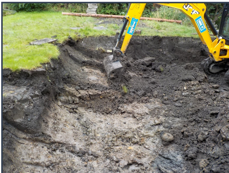
Plate 1 - General view of excavation area
