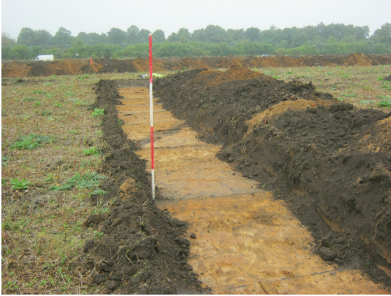
Plate 1: Trench 29 Post excavation with ceramic field drain
