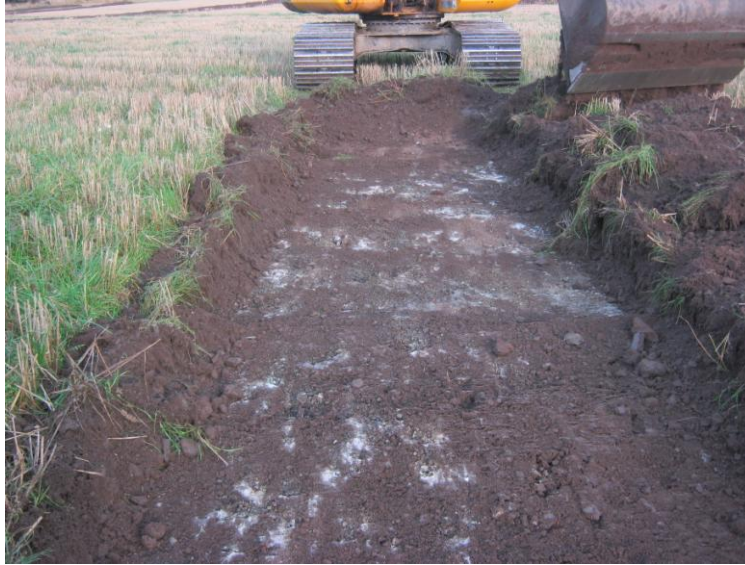
Plate 1 Excavation showing exposed bedrock
